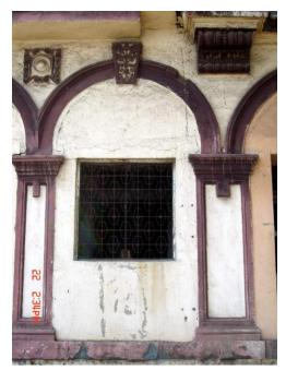
Pilasters below the arch and a window without shutters and framing
