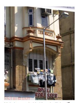
Malad stone cladded façade till the  $1^{\text{st}}$  floor
