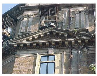
Window opening is refilled and the dentils of the pediment are broken
