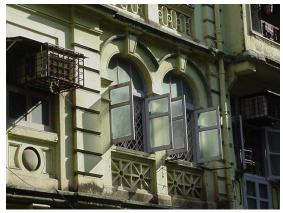
Detail of the semicircular windows with keystone and concrete jali at parapet level
