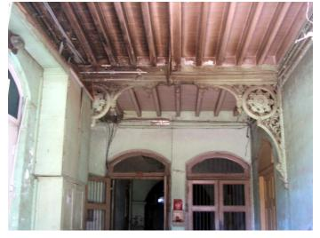
Wooden joist flooring with girders supported by decorative cast iron brackets
