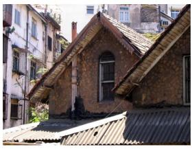
Detail of sloping roof with the downtake pipe puncturing it
