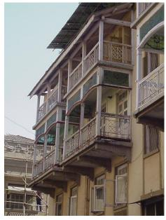
Projecting balconies with stained glass ventilators seen above the 1st floor
