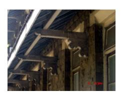
Wooden brackets to support the sloping roof
