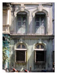
Semicircular openings on the ground floor and segmental openings on the 1<sup>st</sup> floor
