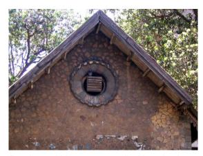
Random rubble masonry wall with a circular ventilator
