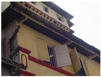
Roofing supported by wooden trusses
