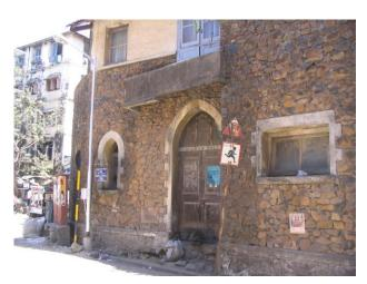
Equilateral point arches for the openings on the ground floor
