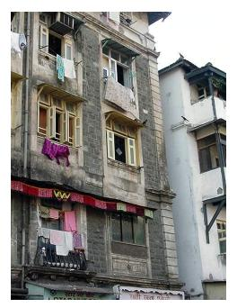
Some parts of the façade are Black Basalt stone cladded
