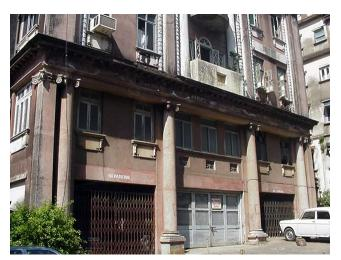
Projecting cornice band at 2<sup>nd</sup> floor level supported by Ionic columns
