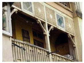
Opaque weather shed supported by wooden brackets
