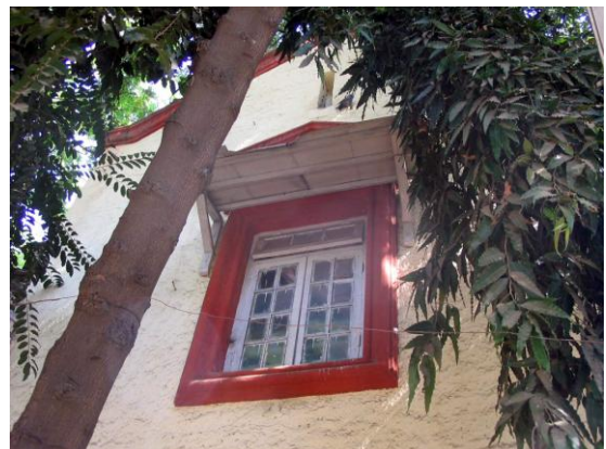
Window detail of building
