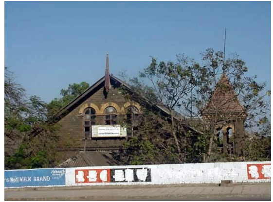
Front view of institutional building from N.M. Joshi road
