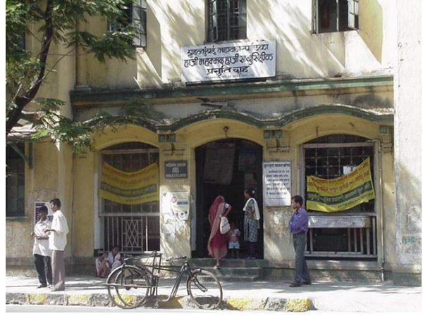
View of main entrance of structure from Dr. Annie Besant Road.
