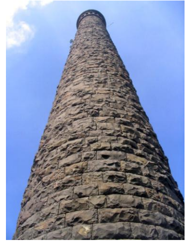
Black Basalt stone coursed masonry used for Chimney
