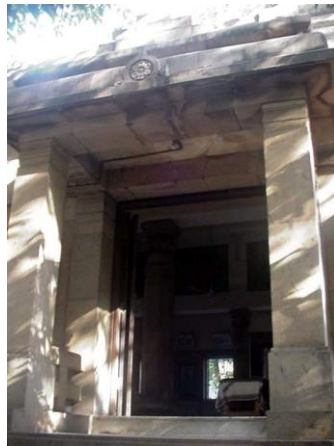
View of main entrance of Mandir.
