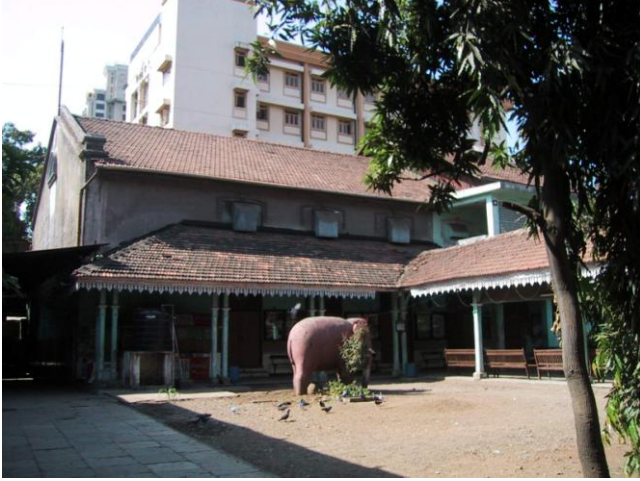
Inside court view of cinema
