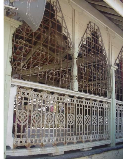
Detail of wooden arches and cast iron jali of Sabha guruh of Mandir.
