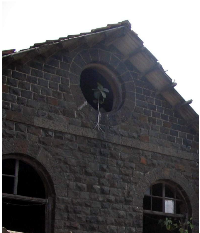
Detail of Black Basalt stone gable wall with circular openings
