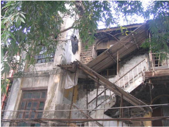
External dog-legged staircase added subsequently on the front façade
