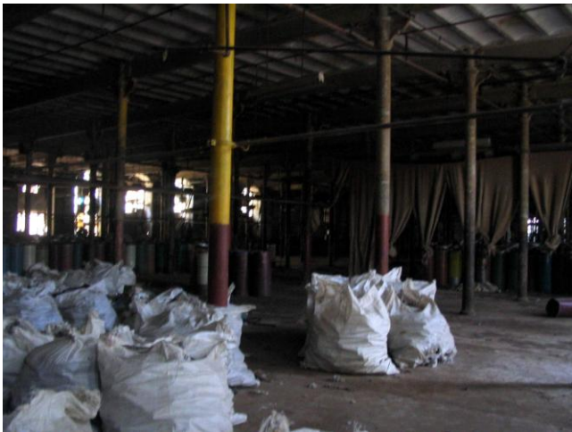
Brick jack arch floor supported on M.S. columns with capitals
