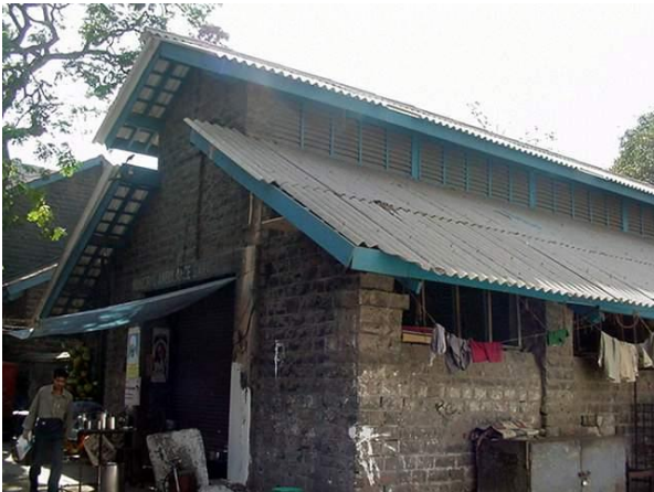
Municipal Ambulance Garage east block corner view from Sane Guruji road
