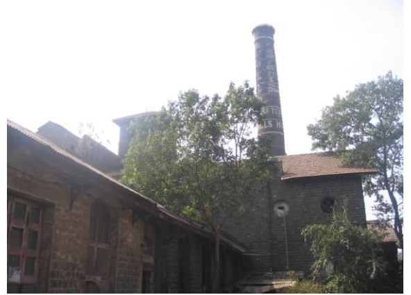
View of Boiler Room and Chimney
