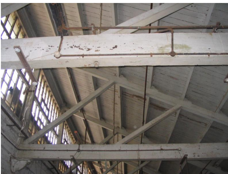
Truss detail with north light
