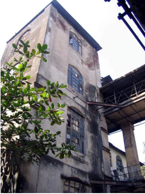
Tower like corner of the Blow Room with segmental arched windows
