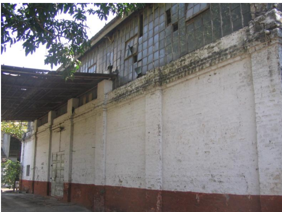
Semicircular arches with architraves around- a fine blend of Vernacular and colonial styles
