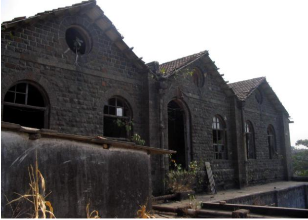
Front view showing multiple sloping roofs on Black Basalt stone gable wall and semicircular arches
