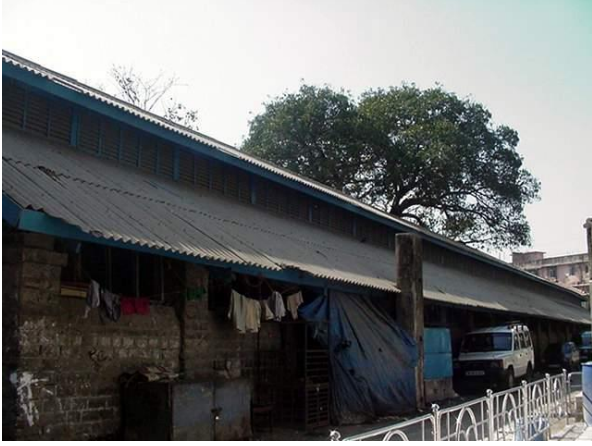
Municipal Ambulance Garage view from side lane on east side.
