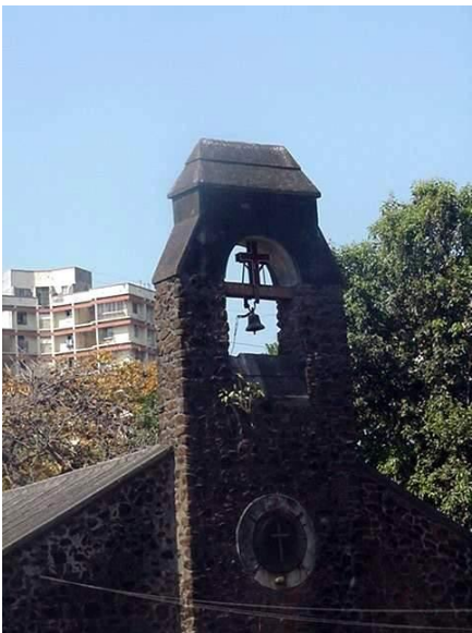
Details of buttresses and bell tower
