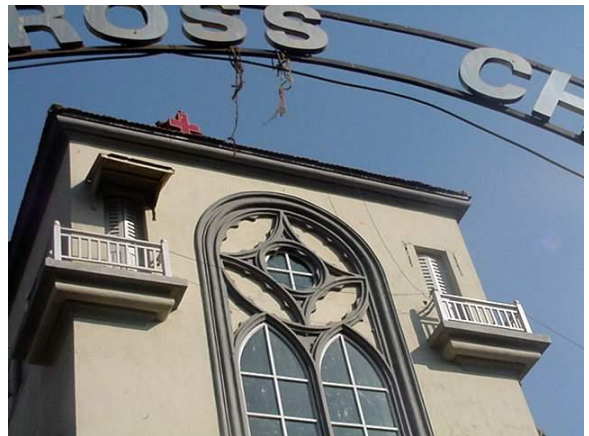
Detail of front tower and balcony with wooden railing
