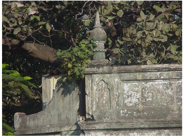
Detail of parapet wall of cemetery from Dr. E. Moses road.
