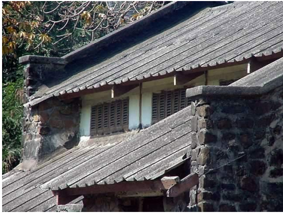
Details of buttresses, roof and ventilators
