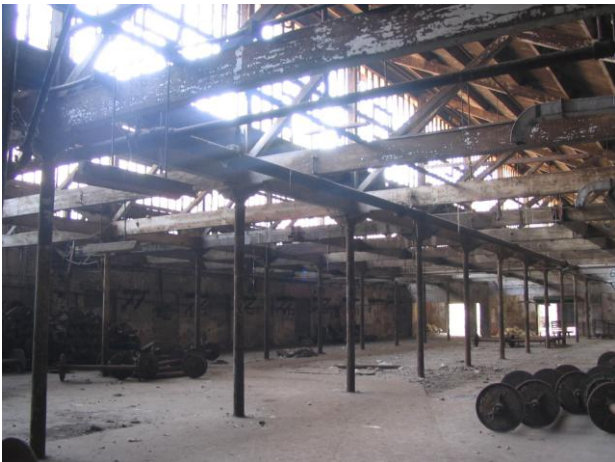
North light wooden trusses for Auto loom department
