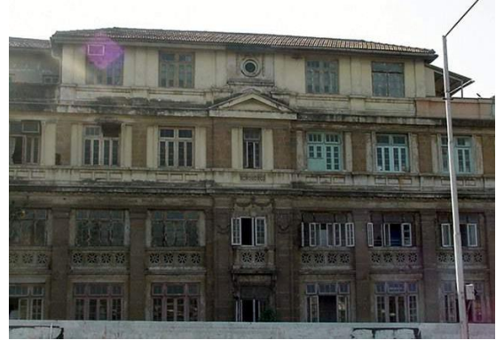
Part front view of building
