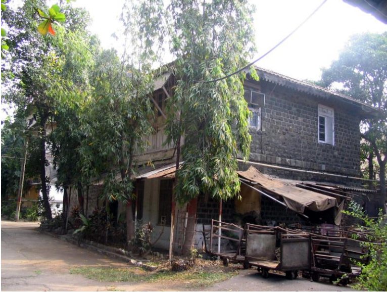
Vernacular style plain stone façade with Mangalore tiled sloping roof
