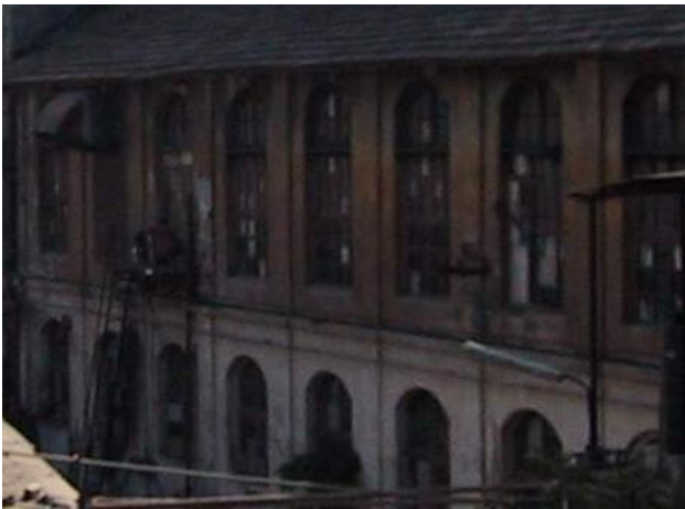
Segmental arched windows at equal intervals on the elongated façade
