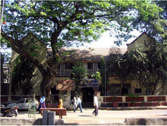
Front view of building from Sakhubai Mohite Marg
