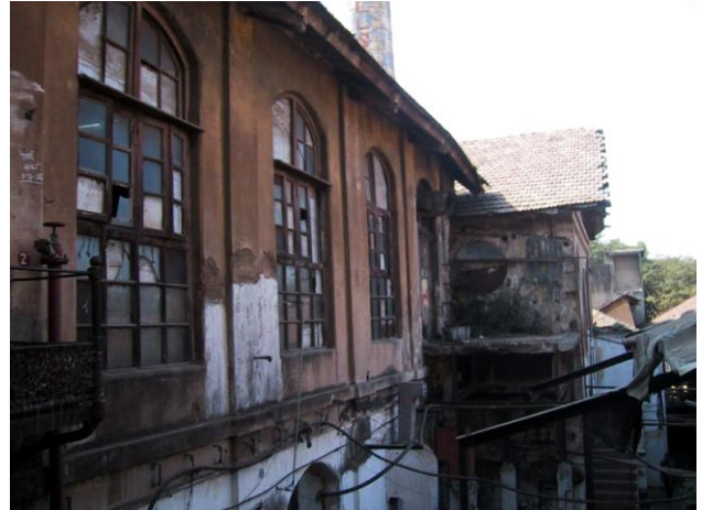
Window detail on first floor
