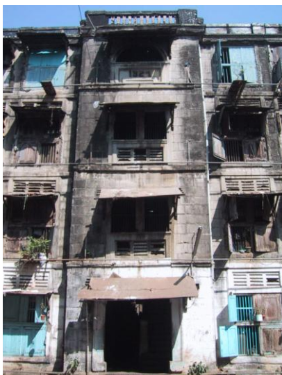
Front view of staircase block of B.D.D. Chawl.
