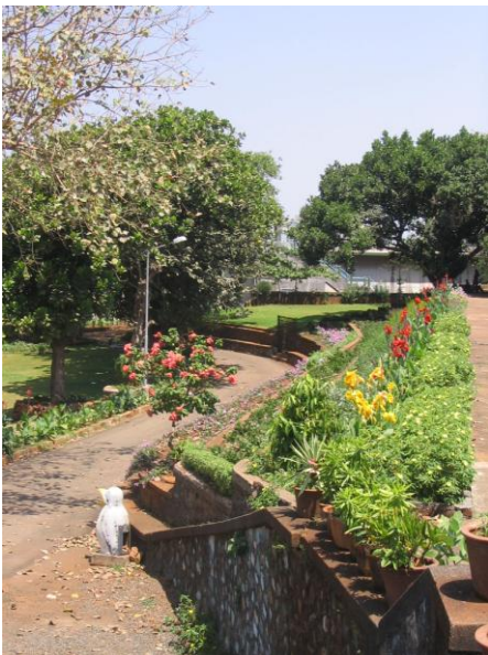
Retaining wall of Reservoir
