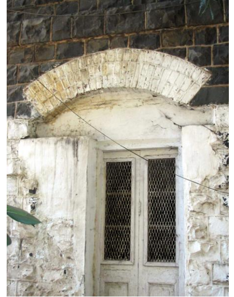
Segmental arch in brick masonry over the opening
