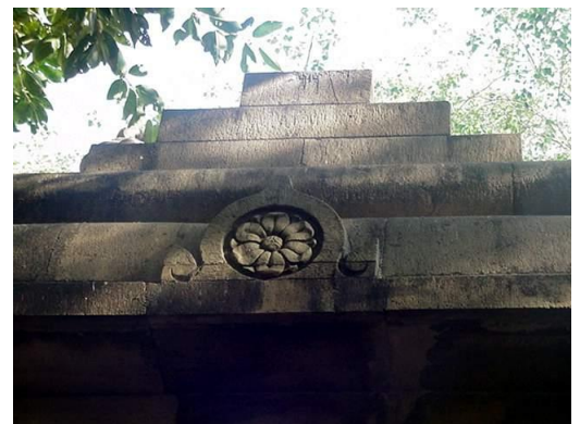
View of floral motif and corbelled shikhar over main entrance of Mandir.
