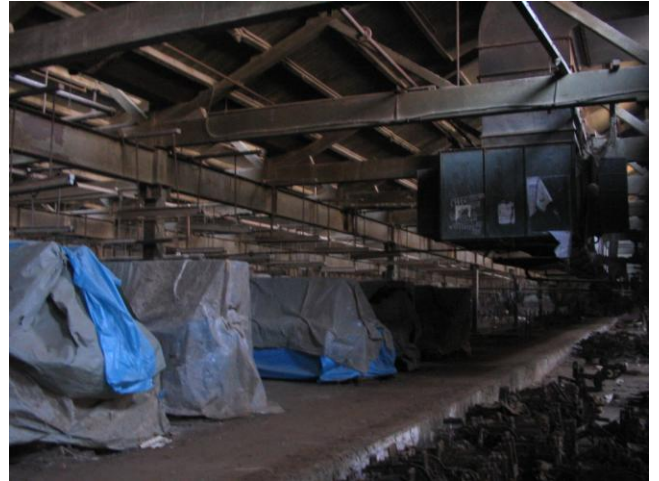
Wooden trusses over the large hall with raised upstand
