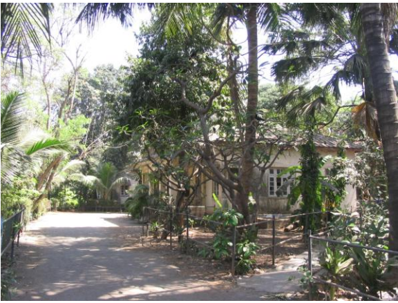
Front view of caretaker's office.
