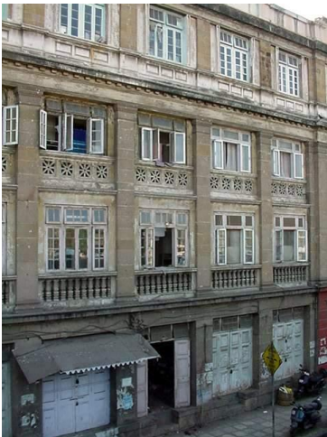
Part front view of building
