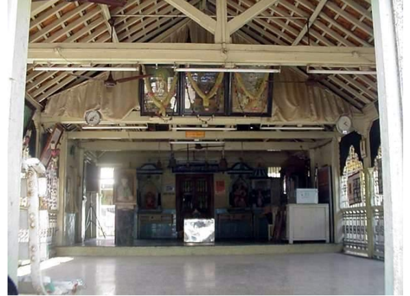
Detail of wooden truss inside Sabha guruh viewing shrine.
