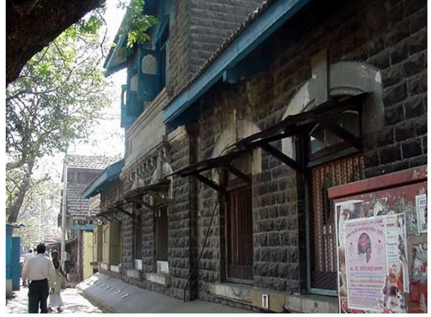
Municipal Ambulance Garage front façade from Sane Guruji road.
