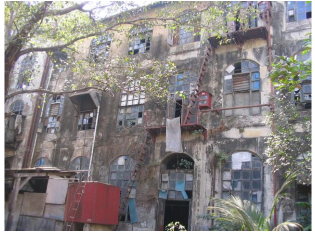
Plain façade of Carding and Framing department with segmental arched windows
