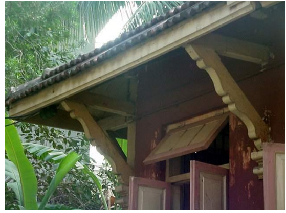
Detail view of wooden bracket supporting roof of Mandir
