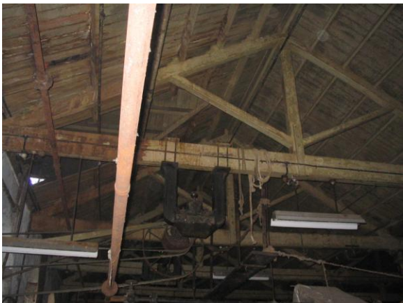
King post wooden trusses for Mangalore tiled sloping roof
