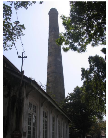
View of Chimney
