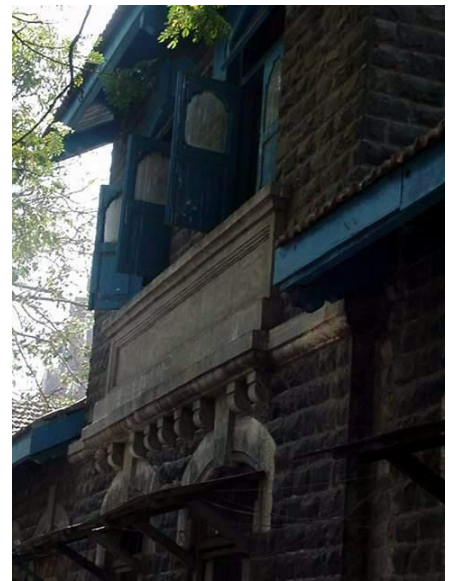
Municipal Ambulance Garage office block window detail
