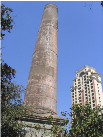
View of the chimney
