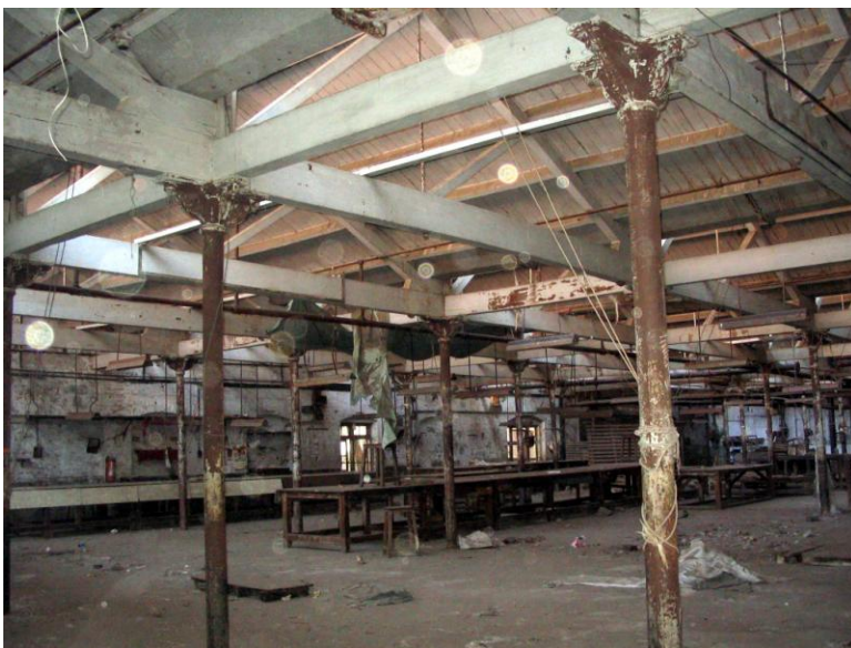
North light wooden trusses supported on M.S. pillars with capitals
