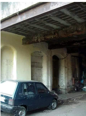
Front view of Rangari Badak Chawl no. 1 from N.M. Joshi road with window detail
