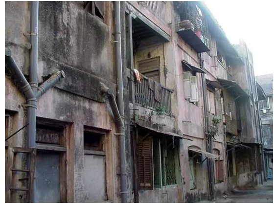
Back view of Rangari Badak Chawl no. 1 from open space.
