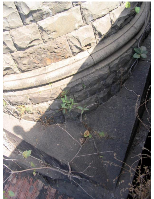
Square base in Black Basalt stone ashlar masonry for chimney
