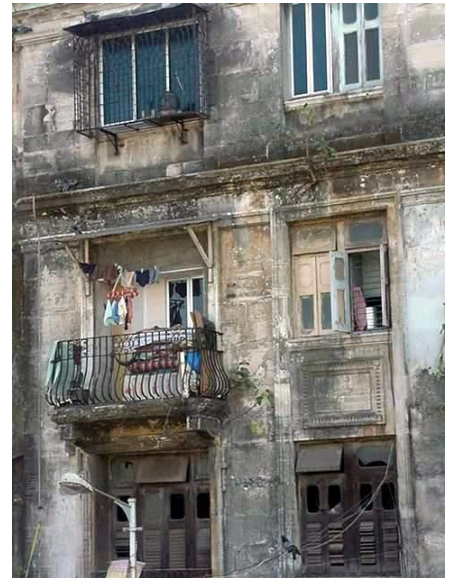
Detail of balcony with cast iron jali and supporting bracket
