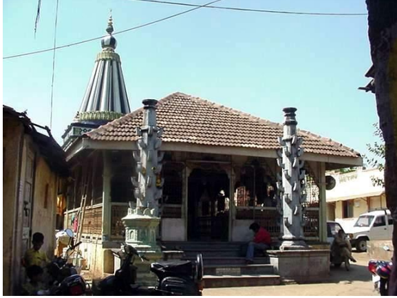
Front view of structure from V.B. Woralikar Marg.
