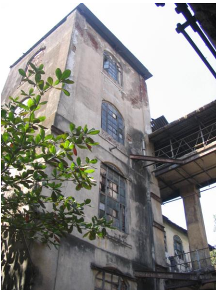
View of Blow Room
