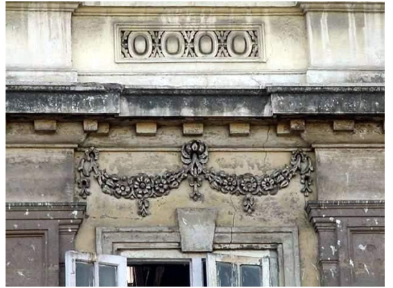
Detail of husk on window with cornice band
