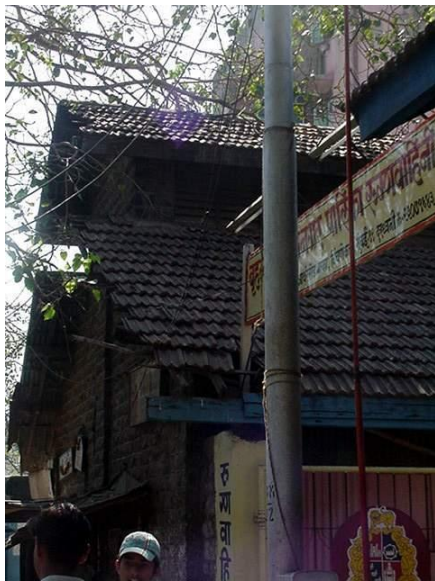
Municipal Ambulance Garage vehicular entrance and west block
