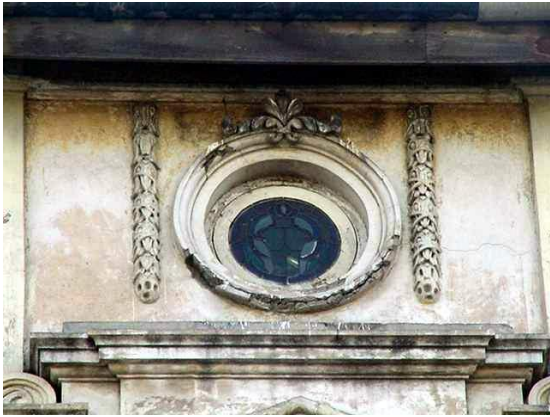
Detail of sun window with cornice band
