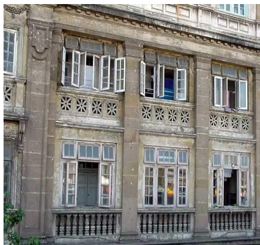
Part front view of building with different stone railing
