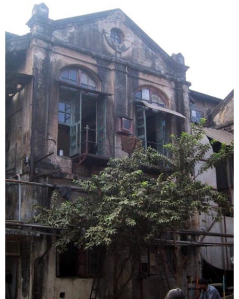
The structures have moderate ornamentation and in fair state
