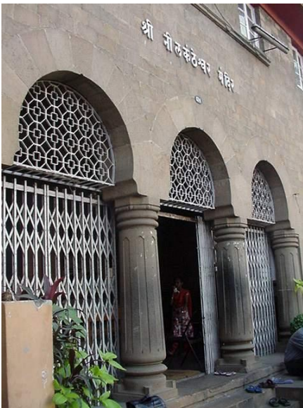
Arched main entrance of Mandir Supported on columns
