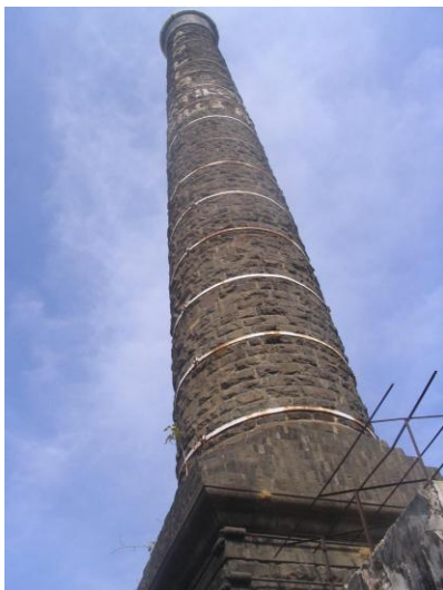
View of the Chimney
