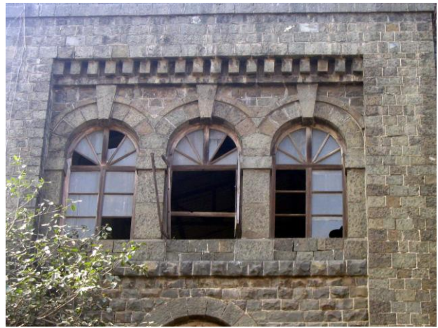
Group of three semicircular arched windows with architrave and dentiled band
