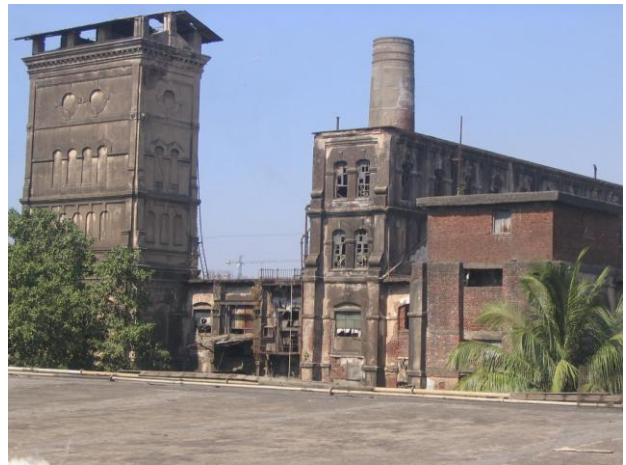
View of the Lancashire chimney and chimney in mill premises
