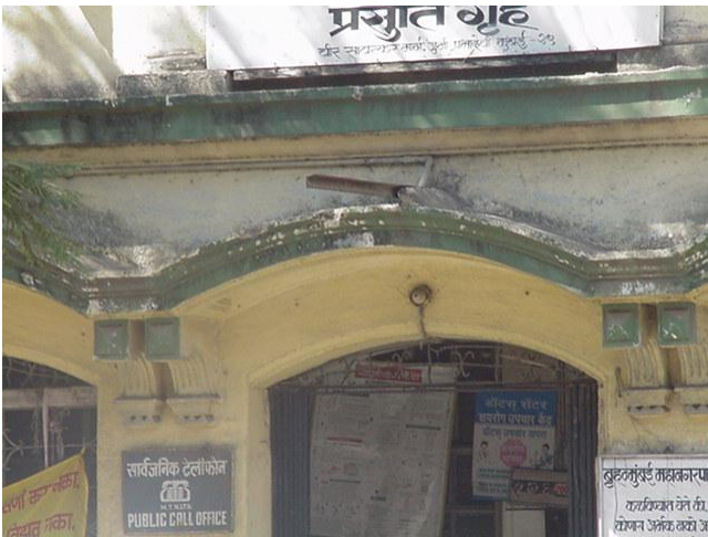
Detail of jack arch of main entrance.
