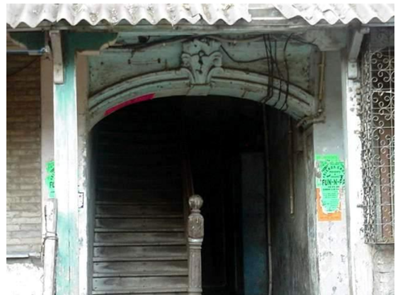
Detail of wooden staircase and segmental arch.
