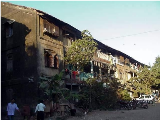
View of Rangari Badak Chawl no. 3 and front open space
