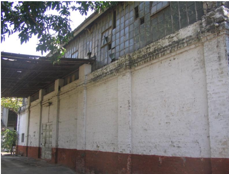
External elevation with dead walls and north light roof truss
