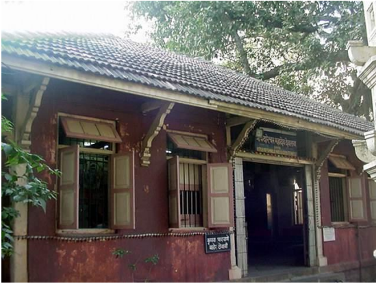
Front view of Mandir from inside of Mandir compound.
