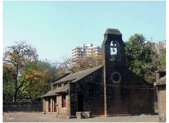
Front view of church from open space
