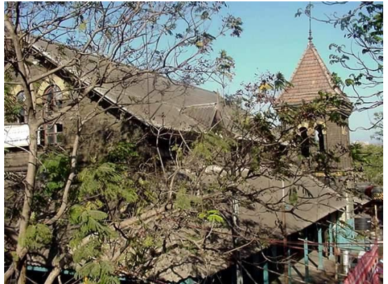
Roof step from N.M. Joshi road
