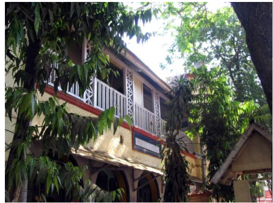
Detail of façade with wooden railing on first floor
