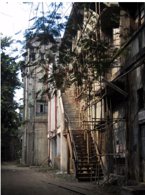
View of the external staircase
