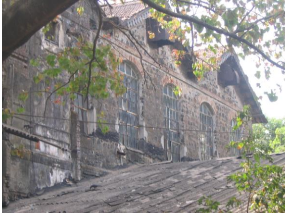
Triple sloping roof over the stone gable with semicircular arched windows
