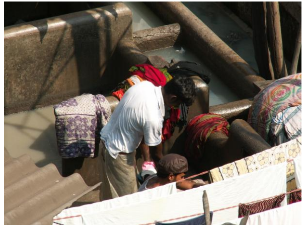
Detail of washing bays
