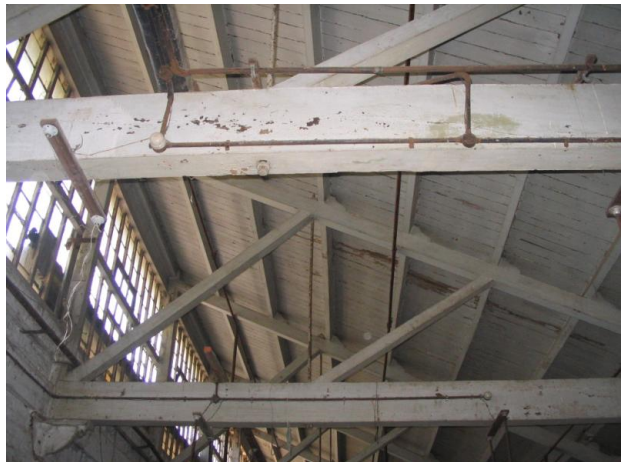
Detail of wooden trusses
