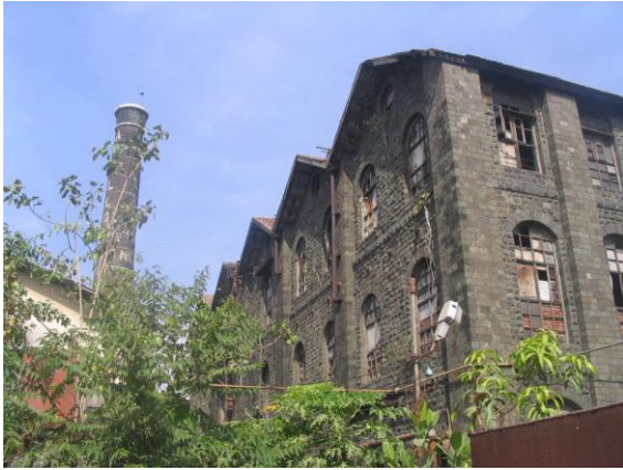
One of the two N.T.C. Mills with structures in stone masonry
