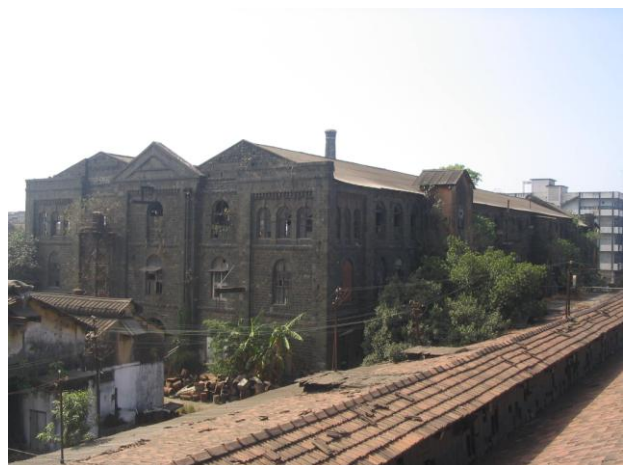
View of impressive stone façade of the Processing department with central triangular pediment
