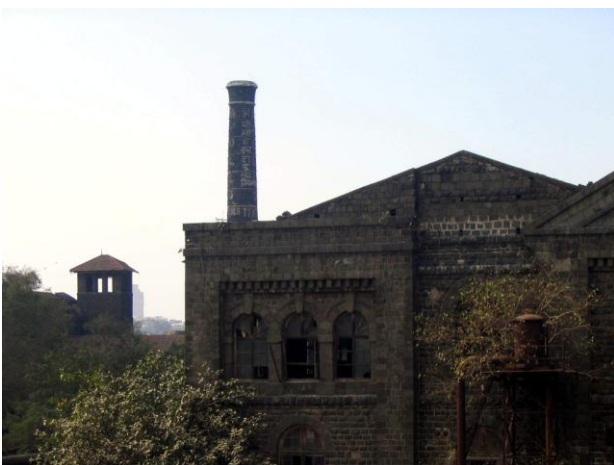
Ornamental stone façade with dentiled band, triangular pediments, fine detailing
