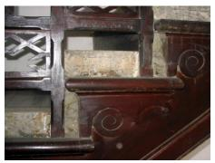
Marble cladding on the existing wooden staircase increase the dead load on staircase
