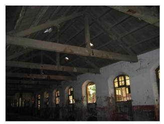
Segmental arched windows at equal intervals and detail of wooden roof trusses
