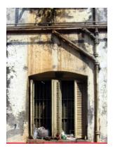
Leakage from the downtake pipes damage the plaster
