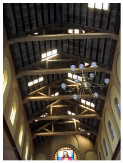
Original timber boardings removed and acrelyic skylight along with asbestos sheet roof is an add-on
