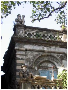
Detail of alternate courses in sand stone and Black basalt with idols of Sadhus and jails on the parapet
