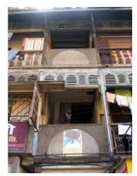
Part of the C.I. railing replaced by plastered brick parapet wall
