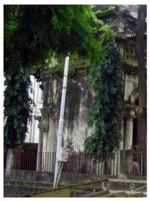
Front arch of the porch has been enclosed by plastered brick work
