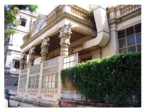
Duct projecting from the front wall disturb the composition of front façade
