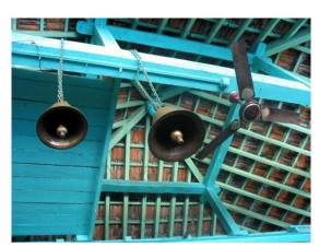
Roof detail with tiles laid directly over purlins on the truss
