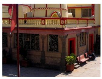
Façade with original carved stone pillars with newly constructed brick walls plastered & painted like Malad stone
