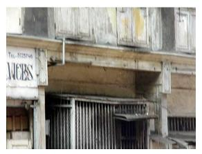
Detail of the load bearing wooden structural members on ground floor
