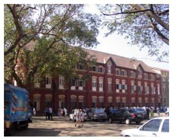
Elongated façade with exposed brick construction, segmental arched windows and Mangalore tiled sloping roof
