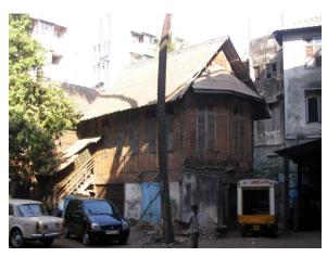
View of the Vernacular style structure in exposed brick masonry and timber frame
