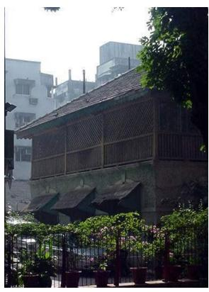
Detail of wooden jail on first floor with chajjas added to the ground floor arched openings
