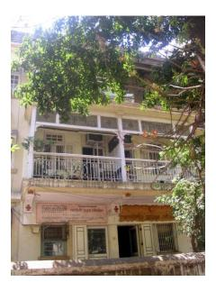
Front balcony supported with decorative bracket with cast iron railing fixed in wooden post supporting stained glass pannel.
