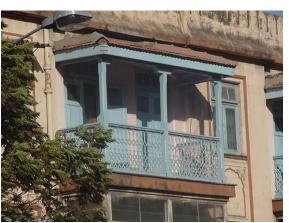
Detail of balcony on south side showing decorative railing, posts supporting sloping roof
