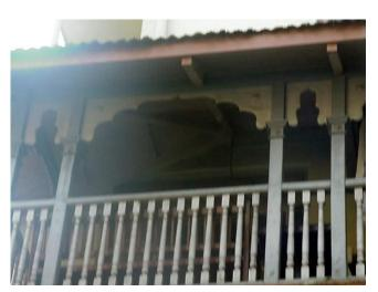
Detail of wooden railing pitched between wooden post supporting slopping roof.
