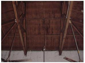
Wooden truss supporting sloping roof above showing purlins and wooden boarding.
