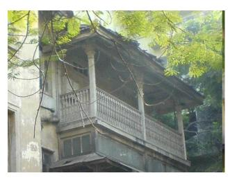
Detail of balcony on second floor with ornamented railing fixed wooden post supporting sloping roof.
