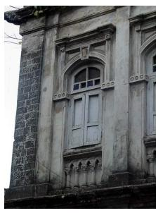
Corner of Block A highlighted in coarsed black basalt masonary.
