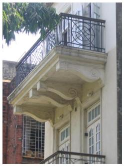
Balcony detail showing decorative brackets, cornice band and cast iron railing.
