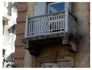
Detail of balcony showing cast iron railing fixed in between wooden posts.
