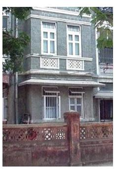
Detail of chajjah, concrete jali, pediments, cornice bands on north façade of building with compound wall.
