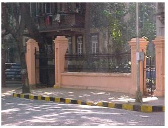
Detail of low height compound wall having cast iron railing in between along with decorative entrance gate.
