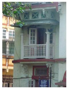
Detail of balcony on 1<sup>st</sup> floor showing decorative wooden bracket, railing, post supporting roof.
