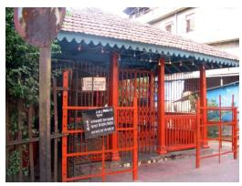
Detail of entrance to temple showing wooden columns supporting sloping roof along with wooden railing.
