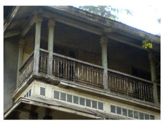
Detail of balcony on second floor with ornamented railing fixed wooden post supporting sloping roof.
