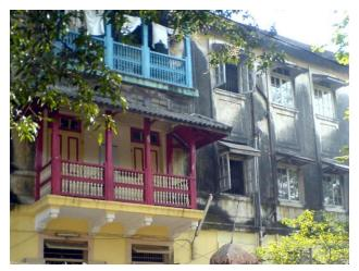
Detail of second floor balcony showing decorative wooden railing fixed in wooden post with ornamented arch supporting sloping roof.
