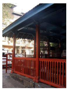
Detail of wooden railing and wooden column resting on stone pad.
