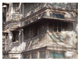
Corner of building with hexagonal block stand out in elevation. Decorative stained glass pannels above window opening.
