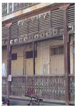
Steel staunction supporting common passage alongwith cast iron railing. Wooden louvers on upperside of common passage.
