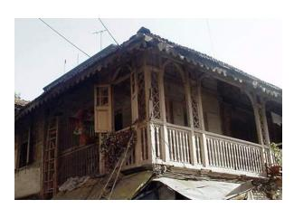
Corner of Block B showing bressed wooden post supporting sloping roof.
