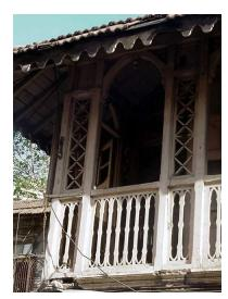
Corner detail of block B showing decorative facia, cast iron railing and wooden post.
