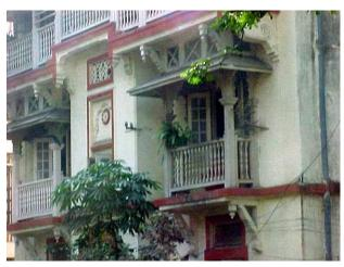
Detail of balcony on 1<sup>st</sup> floor showing decorative wooden bracket, railing, post supporting roof.
