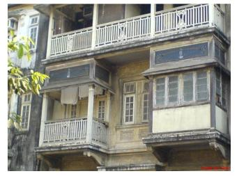
Details of balconies showing wooden railing.
