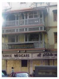
Decorative balcony on first & second floor supported with brackets, stained glass pannels on first floor.
