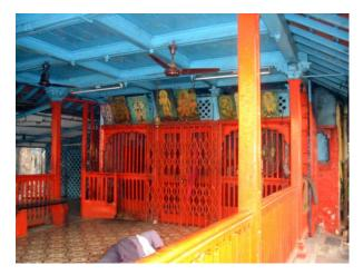
Internal view of temple showing wooden beam resting on column supported by decorative bracket.Door is made up of old mosaic tiles.
