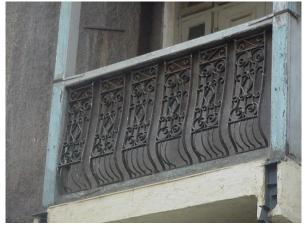
Detail of cast iron railing to balcony
