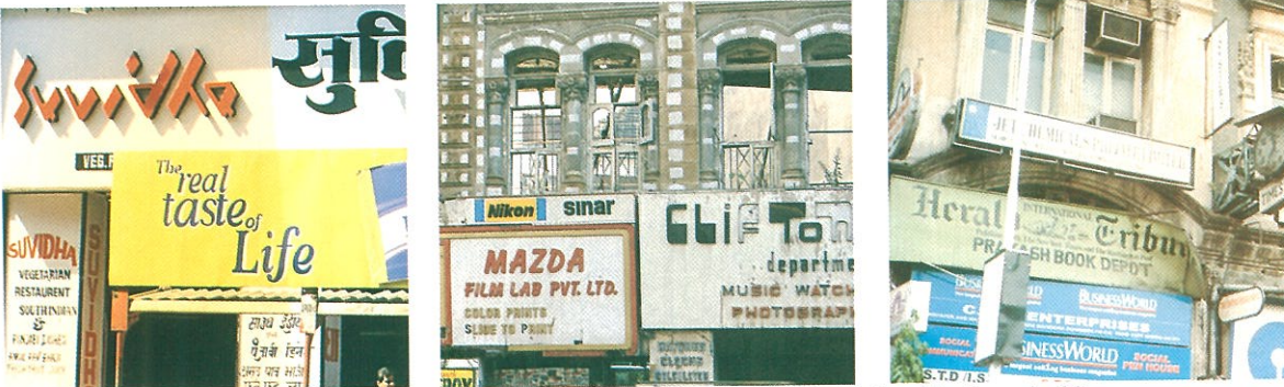
Views of incongruous shopfronts and signboards that obliterated architectural details of heritage buildings
