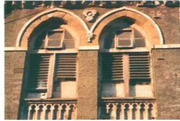
Arched windows of the Times of India Building
