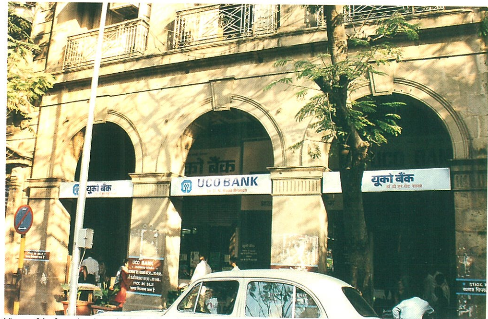
View of before (top) and after (above) images of signboard re-location implemented after the preparation of the guidelines.
