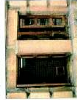
Rectangular openings in the rooms before restoration.
