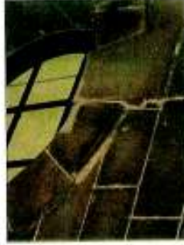
Voussoirs of the Ox eye window restored with lime mortar. The structural cracks were slotted with SS pins.
