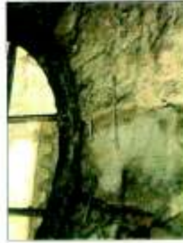
Composite stone walls with brick inner leaf along three sides of the ante-rooms. Note the north wall devoid of the brick leaf, constructed in massive stones, stacked up in a single pile
