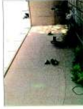
Malad creta plaster with textured finish for the security wall with the surface area broken into joints of uniform width.
