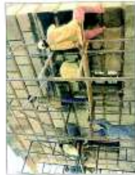
Facade cleaning in progress
