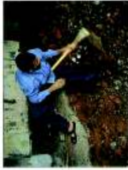
P.C.C. floor and filling within the structure being removed
