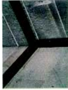
Capping casing in polished wood specially designed to mark the electrical wiring.
