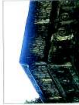
Cornice and frieze bands soiled by tar stains and weathering
