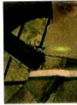
Inclusion of 45 degree angle through the Ox eye window caused damage to the voussoirs and lead to vertical structural cracks.
