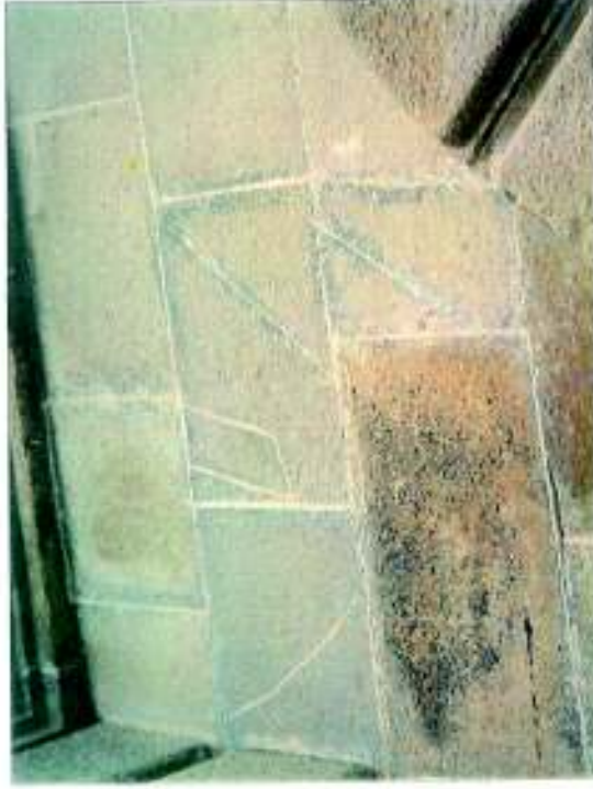
JOINTS AND CRACKS AFTER LIME POINTING
