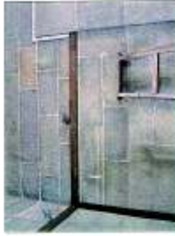
Masking of electrical wiring with polished wood capping casing.
