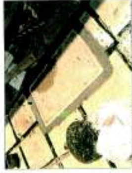
Inspection chambers and service chambers integrated with paving pattern.
