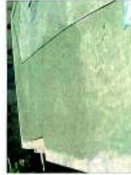
Leveled roof surface before application of IPS layer.
