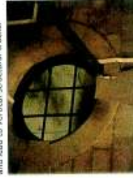
Inclusion of 45 degree angle through the Ox eye window caused damage to the voussoirs and lead to vertical structural cracks.
