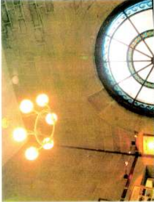
NEW ELECTRICAL WIRING AND FIXTURES IN HARMONY WITH THE HISTORIC STRUCTURE - AFTER RESTORATION.
