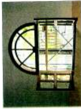
Window during execution stage. Pattern of original direction of openings retained.
