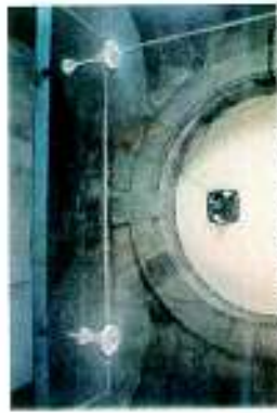
ARCHED OPENING (FRONT) BLOCKED BY MASONRY WALL BEFORE RESTORATION
