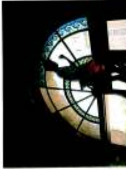
Stained glass panels being placed in position.
