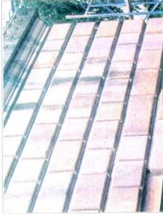
FACADE AFTER RESTORATION
