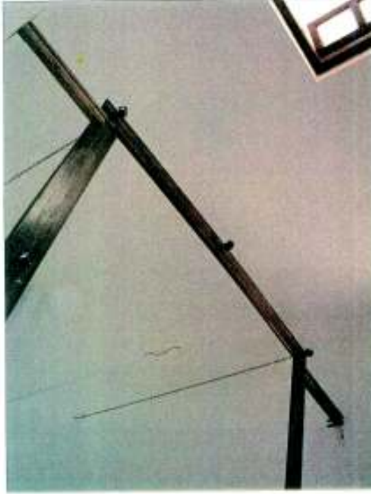
CEILING IN ROOM AFTER RESTORATION
