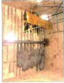
ISMB 250 introduced to strengthen the existing slab and prevent further sagging.
