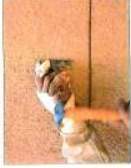
Malad creta plaster being hacked manually to form serrations on the surface. Its color complements the yellow basalt stone facade of the Gatehouse.
