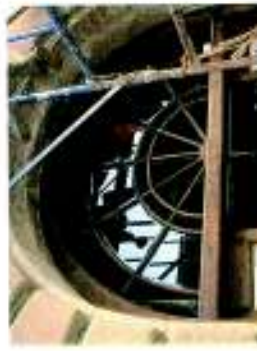
Front door during the execution stage.
