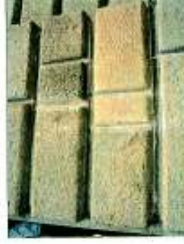
Stone masonry after removal of cement accretions and cleaning.
