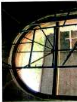
Installation of timber frame
