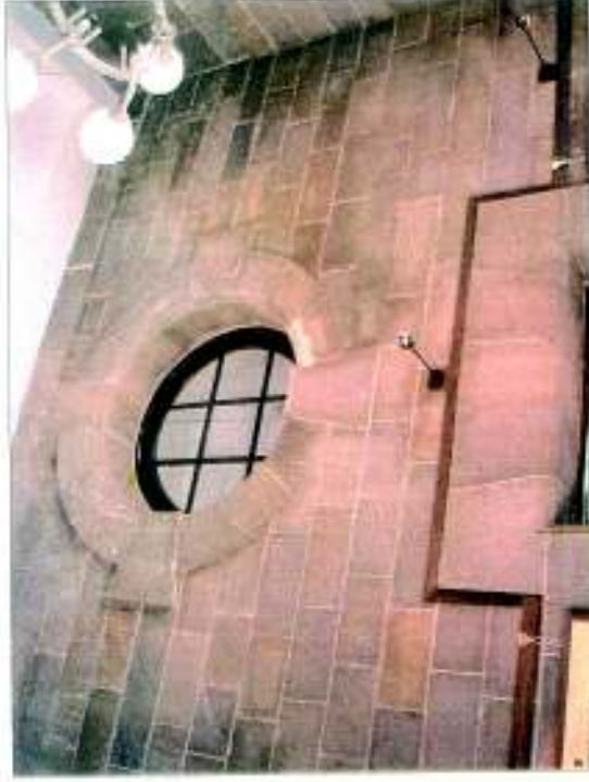
RESTORED OPENINGS IN THE CENTRAL HALL
