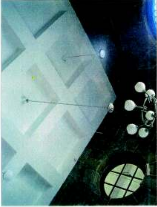
COFFERED CEILING AFTER RESTORATION
