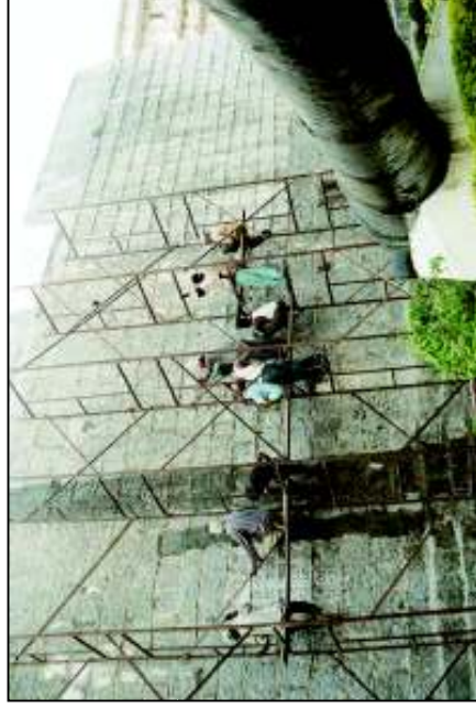
Gentle tapping to remove paint accretions
