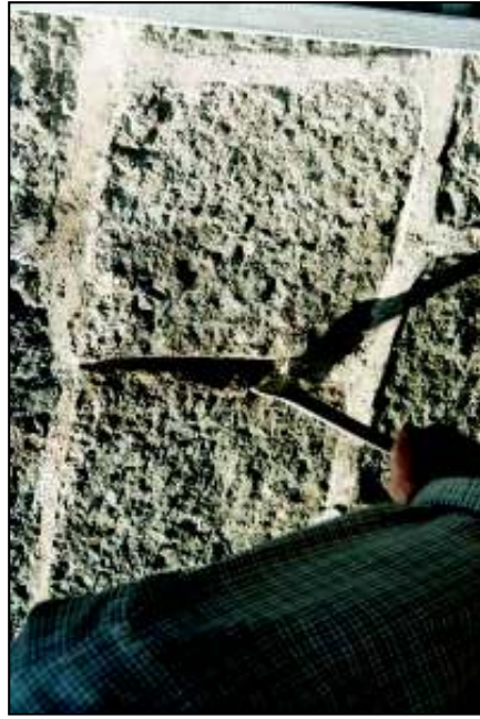
Raking out weakened jointing mortar and flushing out loose mortar
