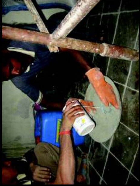
Polymer Aided repair of the damaged and spalled concrete beams was undertaken under the supervision of Structural Rehab Advisor Mr. Arup Sarbadhikary.
