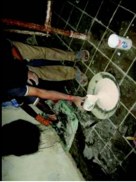
Polymer Aided repair of the damaged and spalled concrete beams was undertaken under the supervision of Structural Rehab Advisor Mr. Arup Sarbadhikary.
