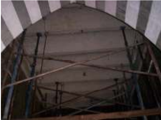
Repair of Jack Arch below flat terrace – First Floor Verandah
