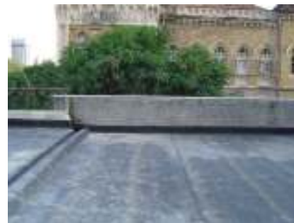
Polymer Mortar Double coat plaster Lead flashing above skirting
