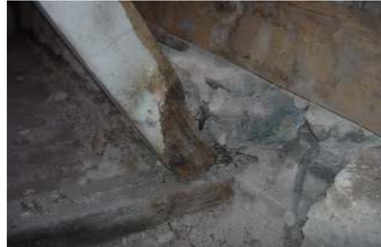
Deteriorated end condition of timber truss
