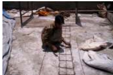
Reinforcement - Structural Steel & Applying Rusticide on Steel reinforcement
