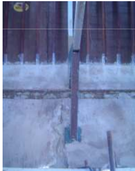
Strengthening of the truss member
