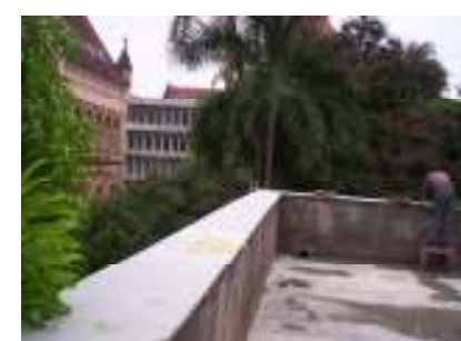
Kottah Stone fixing
