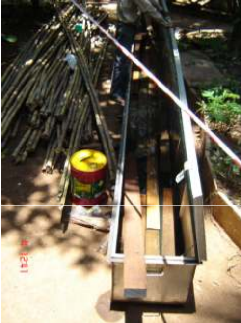
All timber was treated for termites
