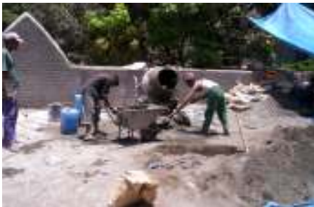
M25 Grade Concrete for terrace
