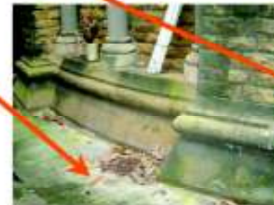
Stone Staining & Damaged Mouldings
