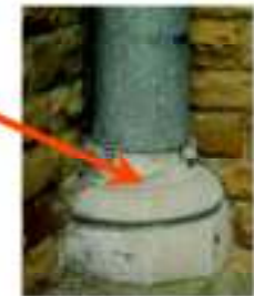
Stone Staining & Damaged Mouldings
