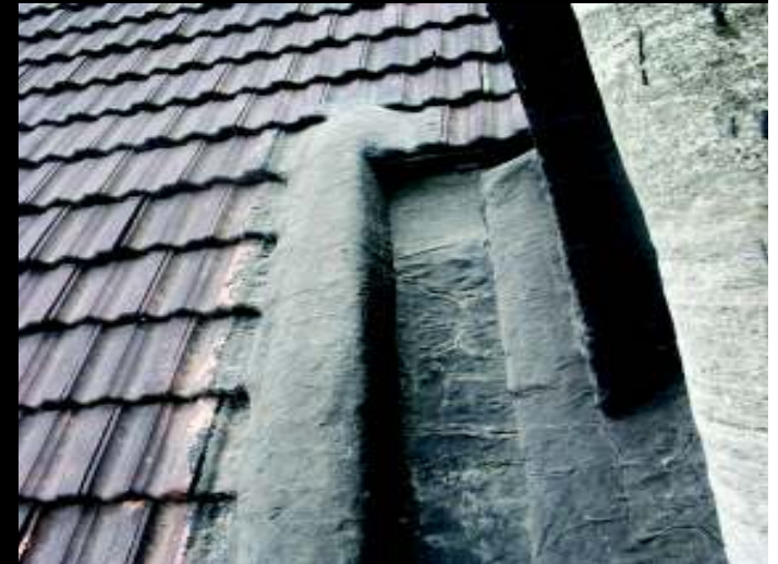
Gutter along Gable end
