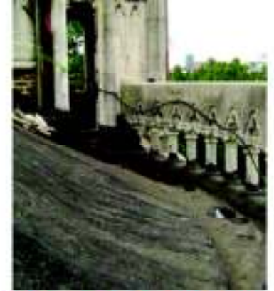
Stairwell masonry in need of pointing
