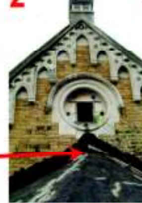
Stairwell masonry in need of pointing
