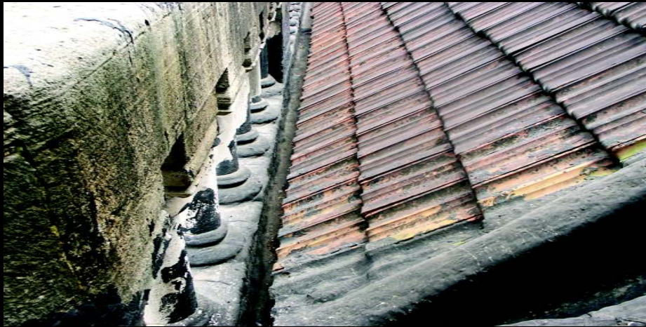
Upper Level Gutter
