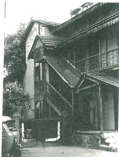
Above Porch Detail Below External Staircase Source – Joshi (1995)
