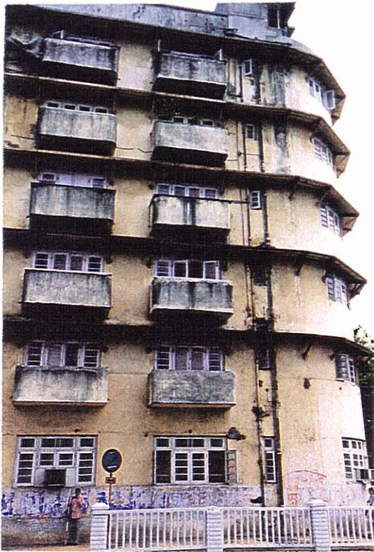
Chhajjas Replaced, Moonlight Building Source www.geocities.com
