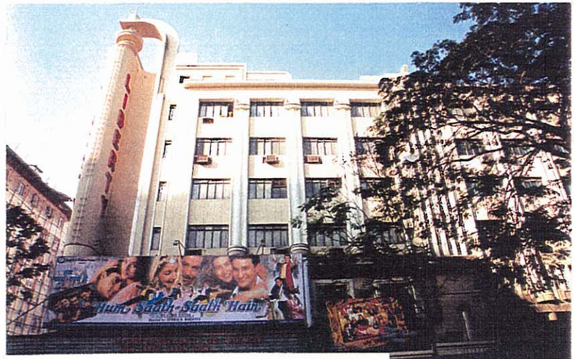
Significant Art Deco Building, Liberty Cinema Source RCACC 1999/2000
