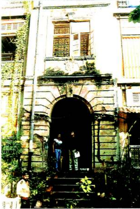
"Govind Niwas" along S.K.Barodawalla Marg - facing demolition and New High rise
