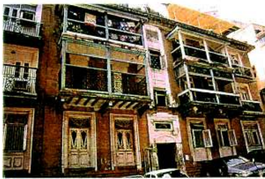
Tulsi Mahal - Raghavji Road
