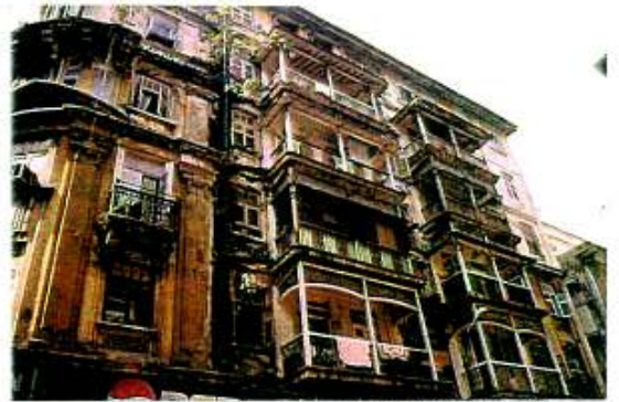
Old Botawalla Building- Junction of August Kranti Marg & Raghavji Road
