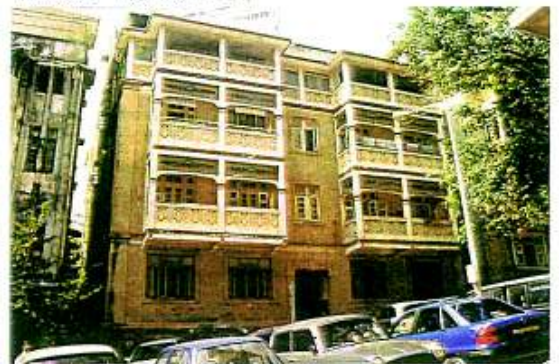
Hill View - Raghavji Road
