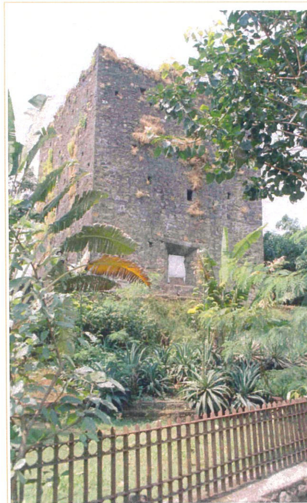
Remains of the North gateway of the fort.
