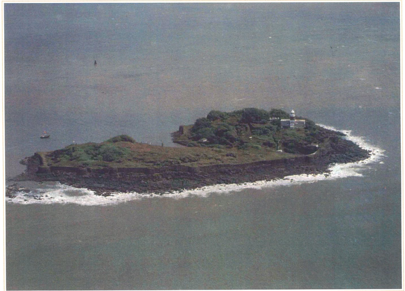
Aerial view of Khanderi fort
