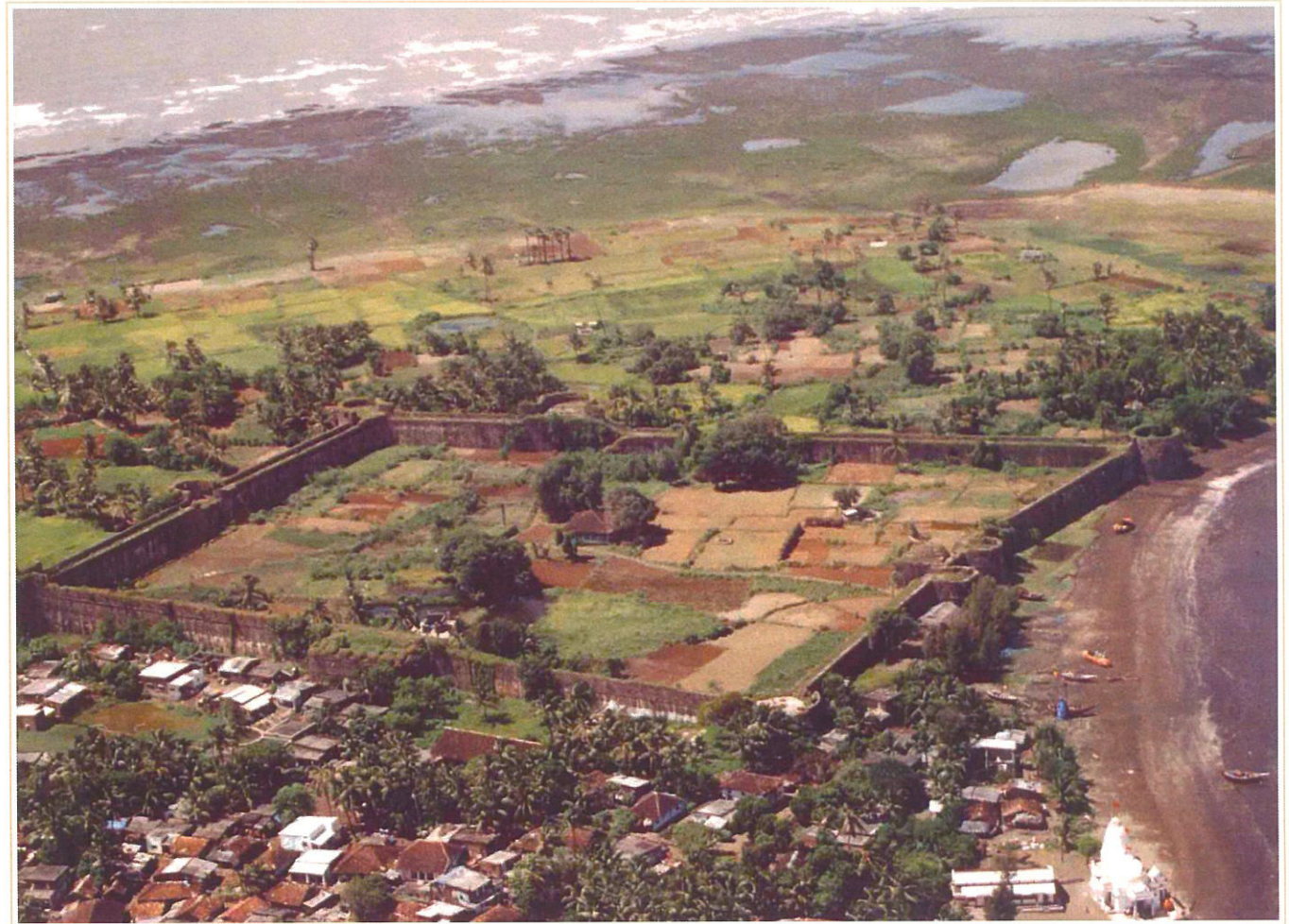
Aerial view of Arnala fort
