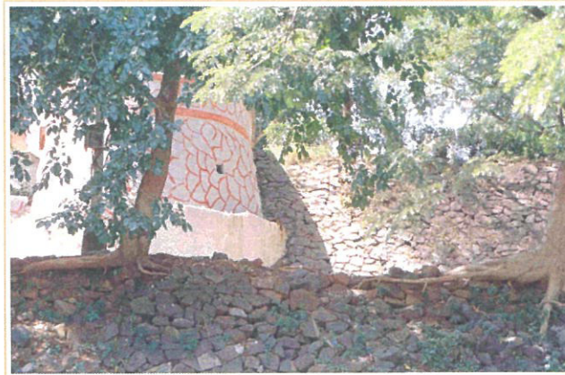
A view of newly painted bastion with the original ramparts.
