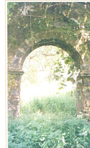
the semi-circular arch observed in surrounding arcade.
