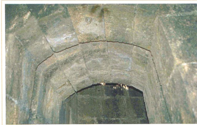
The niche along the jamb of the bastion entrance.
