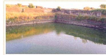
View of the Fresh water tank within the fort
