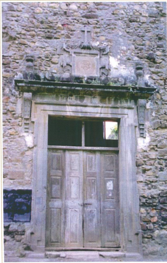
The Matrix of St. Joseph displaying the use of a variety of stones
