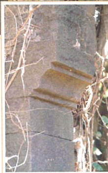
Column cornice detail at the entrance gateway
