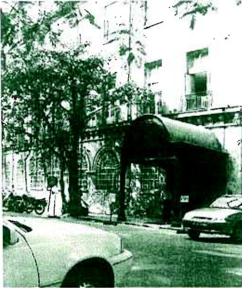
Garishly painted porches ruins the character of this building and its environs. Such colour schemes should not be allowed.
