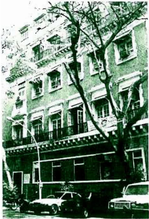
Inappropriate placement of AC's, sealing of opening, changing of original teakwood door and window details is to be stopped so as to retain the Edwardian character of this precinct.
