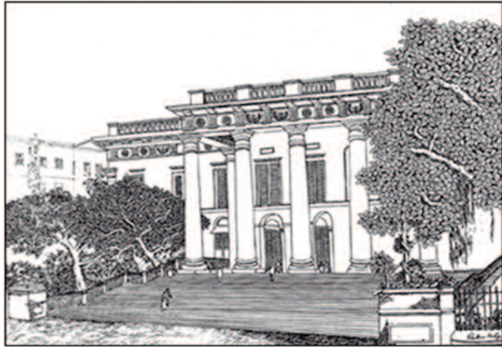
Town Hall – Front view
