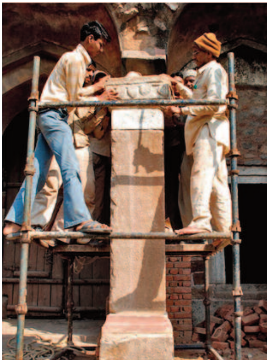
Reinstalling capitals collected from the site
