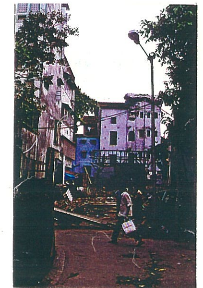
STAGE III: EMPTY PLOT ON COMPLETE DEMOLITION
