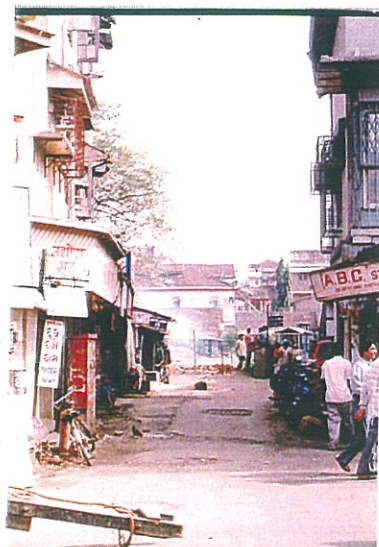
PHOTOGRAPH SHOWING VACANT PLOT AFTER DEMOLITION
