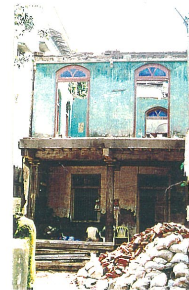
STAGE II: DEMOLITION UNDERWAY
