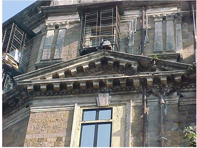
Window opening is refilled and the dentils of the pediment are broken
