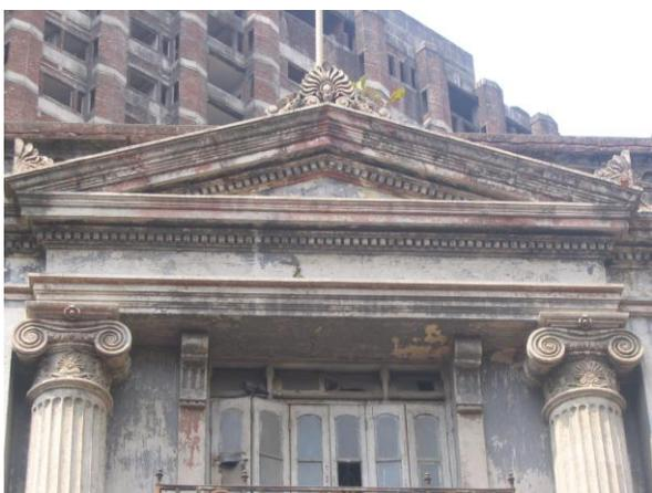
Triangular pediment with dentils and ionic columns below
