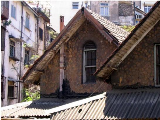
Detail of sloping roof with the downtake pipe puncturing it
