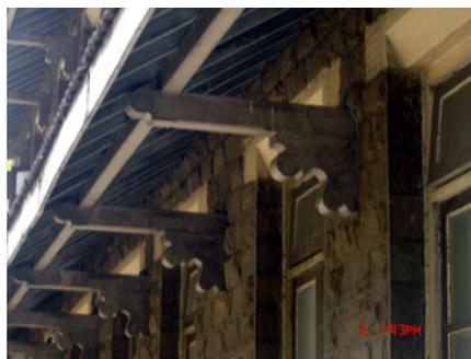
Wooden brackets to support the sloping roof
