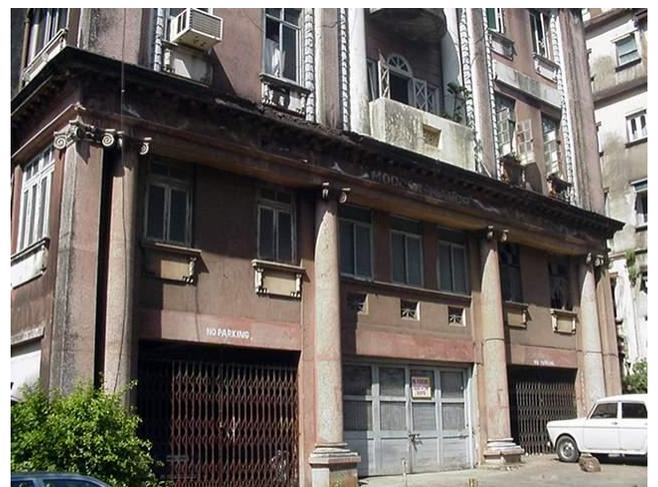
Projecting cornice band at 2<sup>nd</sup> floor level supported by Ionic columns
