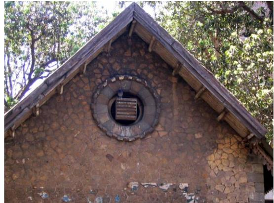
Random rubble masonry wall with a circular ventilator
