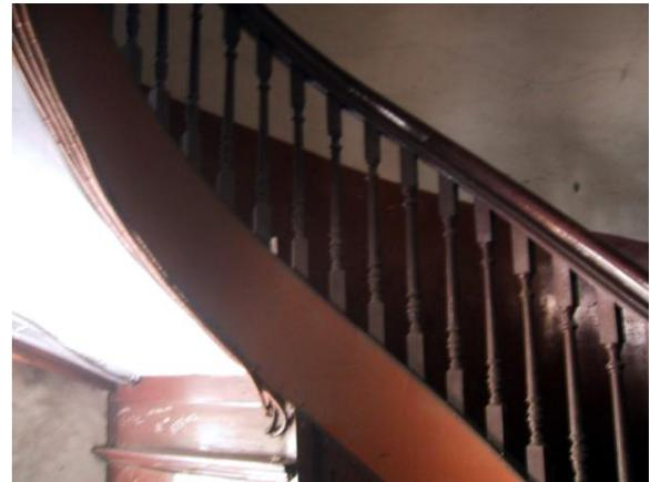
Open well, winding wooden staircase
