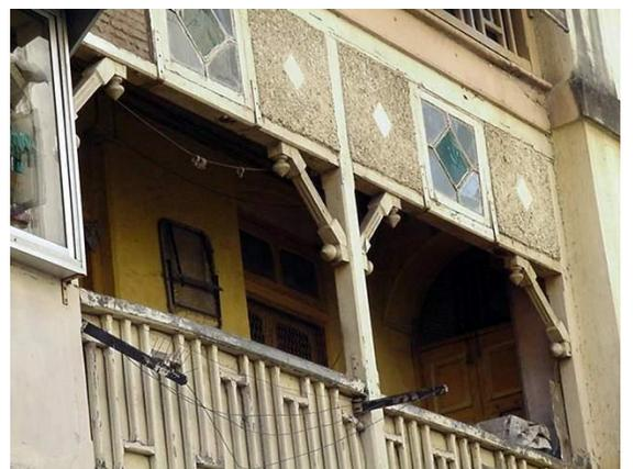
Opaque weather shed supported by wooden brackets
