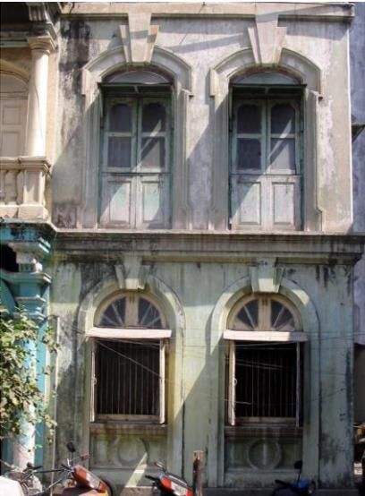
Semicircular openings on the ground floor and segmental openings on the 1<sup>st</sup> floor
