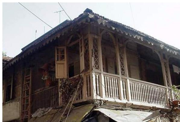
Corner of Block B showing bressed wooden post supporting sloping roof.
