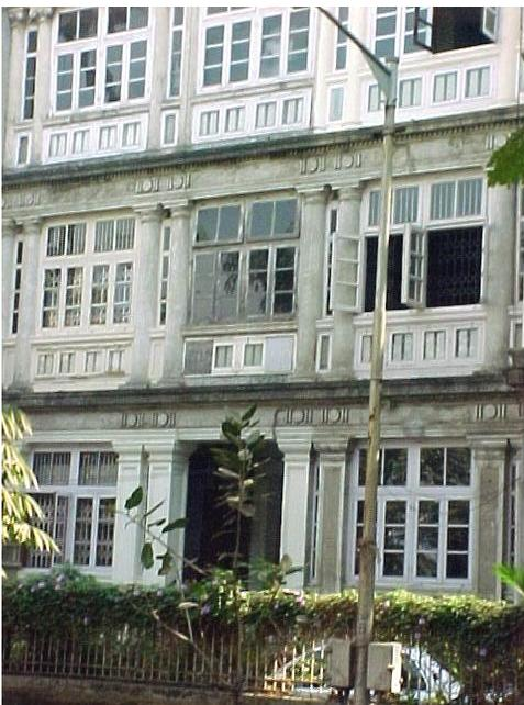
Detail of front façade showing different styles of columns on each floor with decorative motifs and concrete band.
