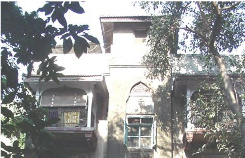
Detail of balcony having decorative cast iron railing, Moorish arch and staircase block with sloping roof.
