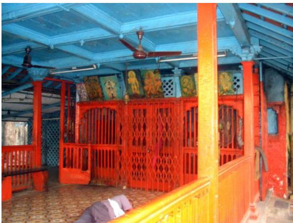
Internal view of temple showing wooden beam resting on column supported by decorative bracket. Door is made up of old mosaic tiles.
