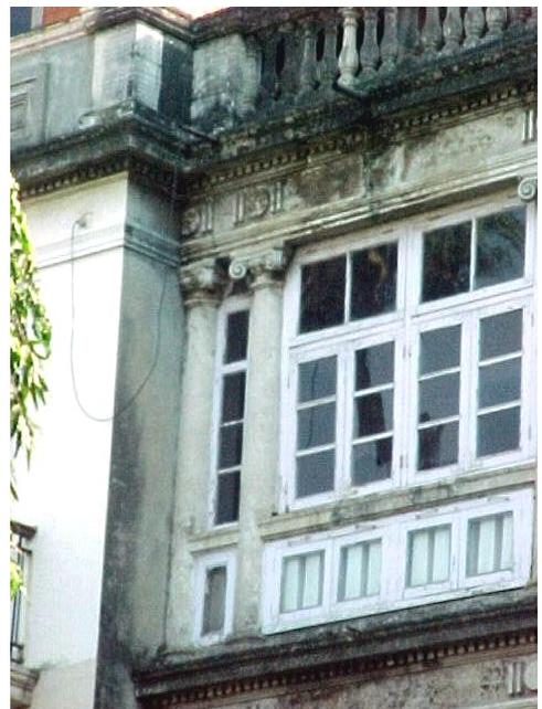
Second floor showing Doric columns with cornice band, motifs along with concrete railing.
