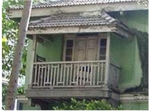
Detail of projecting balcony with wooden railing and cornice band at floor level.
