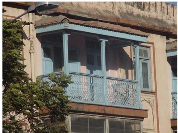
Detail of balcony on south side showing decorative railing, posts supporting sloping roof
