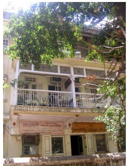
Front balcony supported with decorative bracket with cast iron railing fixed in wooden post supporting stained glass panel.
