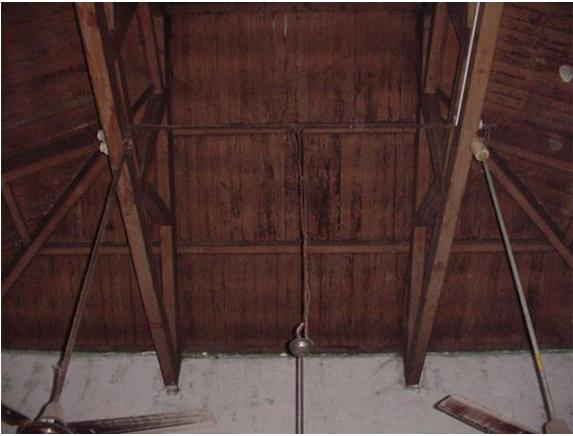
Wooden truss supporting sloping roof above showing purlins and wooden boarding.
