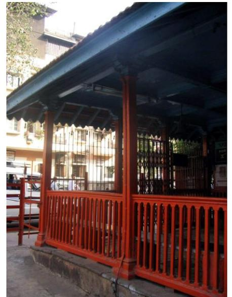
Detail of wooden railing and wooden column resting on stone pad.
