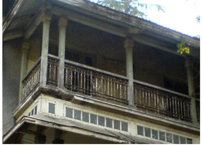
Detail of balcony on second floor with ornamented railing fixed wooden post supporting sloping roof.
