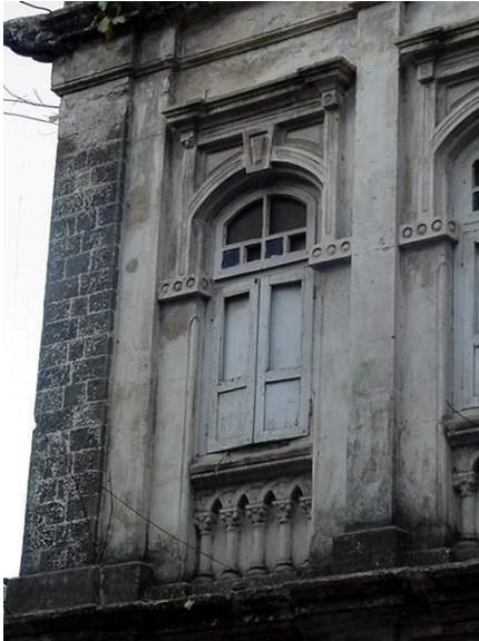
Corner of Block A highlighted in coarsed black basalt masonry.
