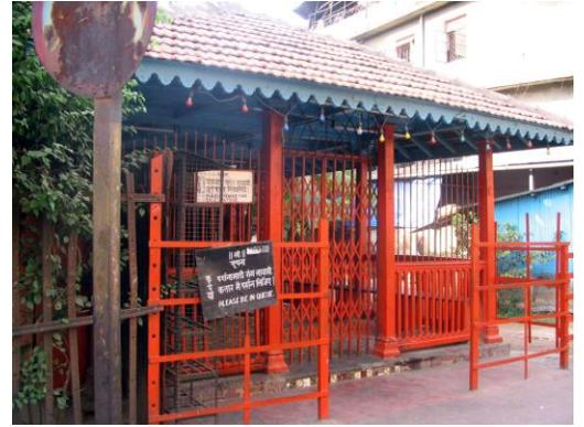
Detail of entrance to temple showing wooden columns supporting sloping roof along with wooden railing.
