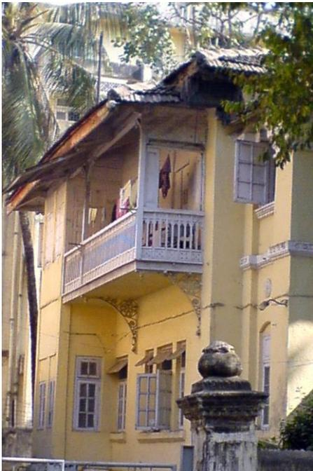
Decorative cast iron brackets supporting balcony on north side having wooden railing, post supports sloping roof
