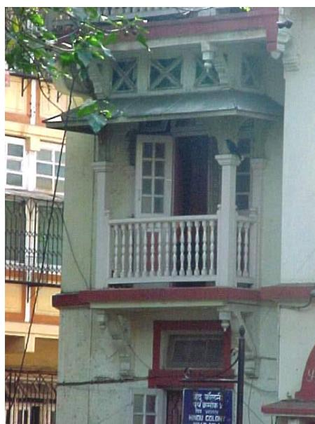
Detail of balcony on 1<sup>st</sup> floor showing decorative wooden bracket, railing, post supporting roof.
