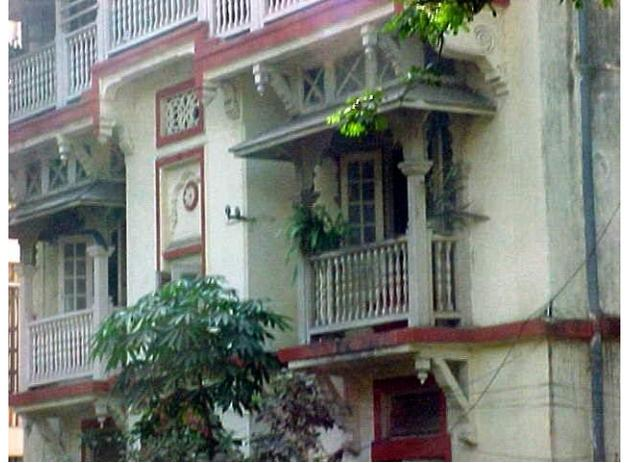
Detail of balcony on 1<sup>st</sup> floor showing decorative wooden bracket, railing, post supporting roof.
