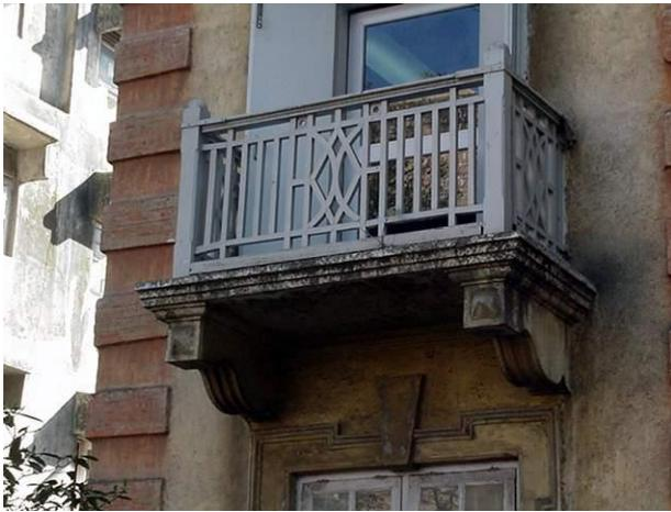
Detail of balcony showing cast iron railing fixed in between wooden posts.
