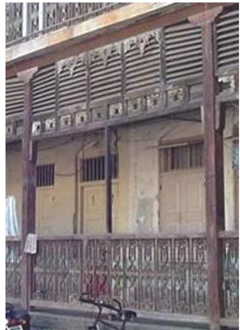
Steel stanchion supporting common passage alongwith cast iron railing. Wooden louvers on upperside of common passage.
