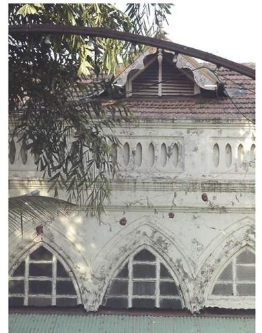
Arched opening and concrete parapet wall, roof levels with louvers.
