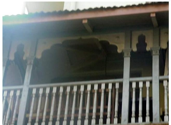
Detail of wooden railing pitched between wooden post supporting slopping roof.
