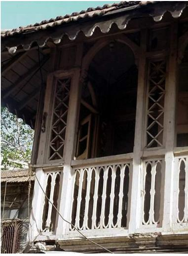
Corner detail of block B showing decorative fascia, cast iron railing and wooden post.
