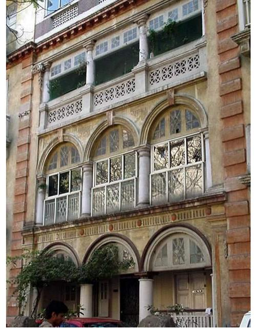
Detail of front façade showing semicircular arches resting on circular columns, stucco work at ends and stained glass panel.
