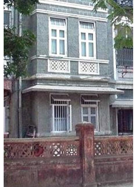
Detail of chajjah, concrete jali, pediments, cornice bands on north façade of building with compound wall.
