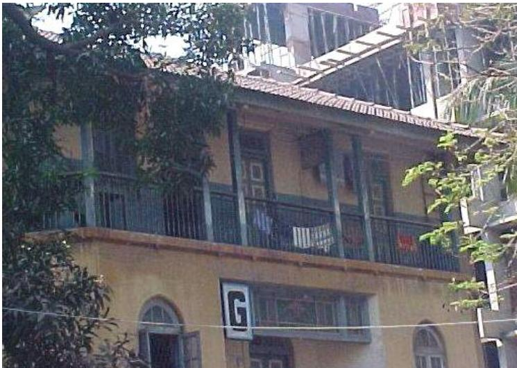
Top floor with recessed balcony with wooden railing and wooden posts supporting the mangalore tile roof above. Stained glass pannels on first floor balcony.
