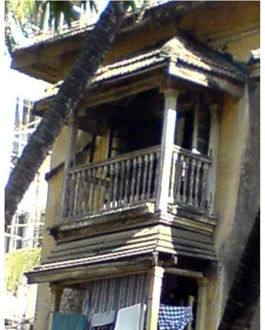
Detail of balcony on second floor with cast iron railing fixed in wooden post.
