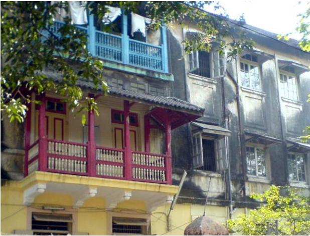
Detail of second floor balcony showing decorative wooden railing fixed in wooden post with ornamented arch supporting sloping roof.
