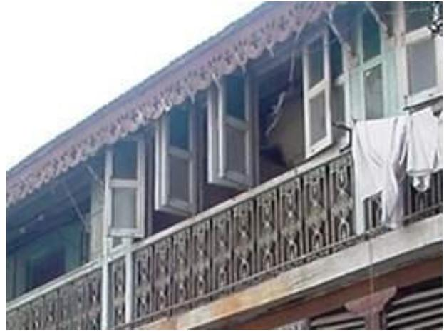
Decorative cast iron railing on first floor having common passage supported with wooden post. Decorative wooden facia is supported with small brackets.
