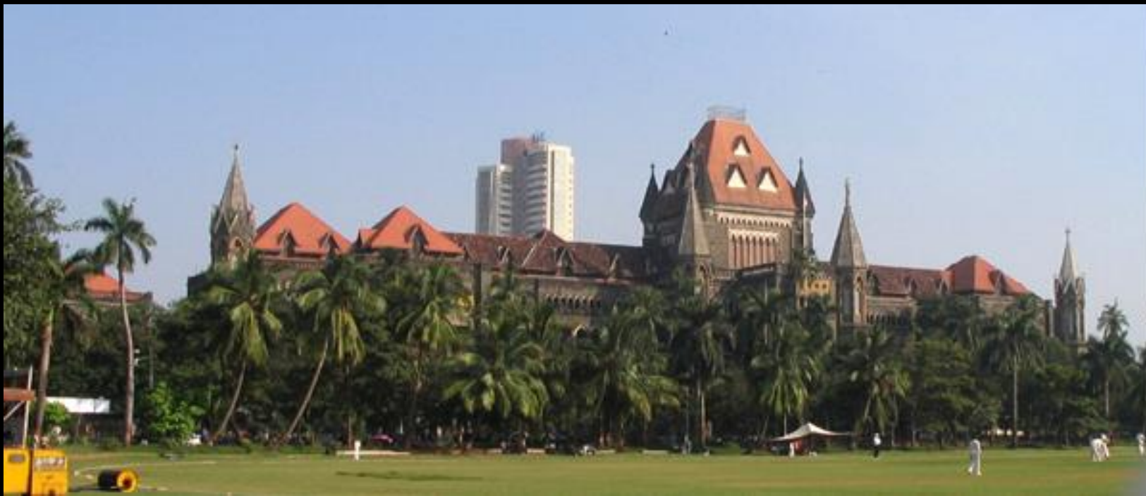
Front View of High Court
