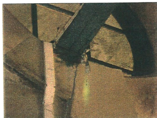
Insertion of MS angle through the ox eye window caused damage to the voussoirs and lead to vertical structural cracks.
