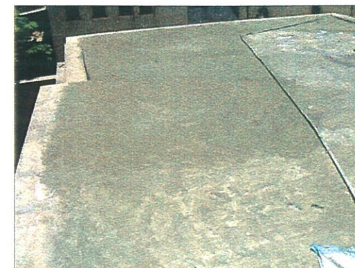
Leveled roof surface before application of IPS layer.
