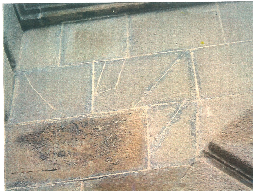
JOINTS AND CRACKS AFTER LIME POINTING
