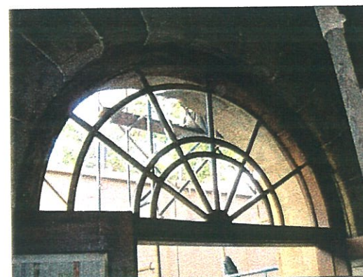
Sash bars in the semicircular portion of the arched opening placed in position.
