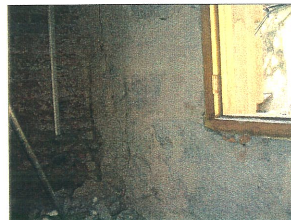
Composite stone walls with brick inner leaf along three sides of the ante-rooms. Note the north wall devoid of the brick leaf, constructed in massive stones, stacked up in a single pile
