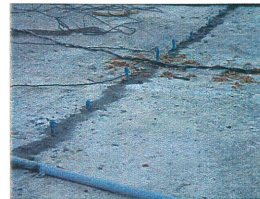
Roof slab prepared for polymer grouting
