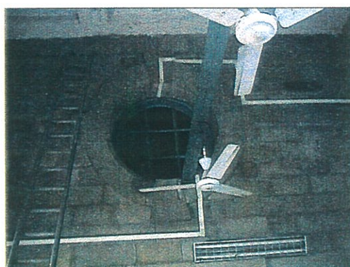
Fans suspended on steel beams, taking support on the voussoir of the intrados of the Bulls eye
