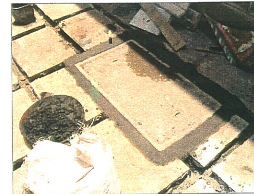
Inspection chambers and service chambers integrated with paving pattern.
