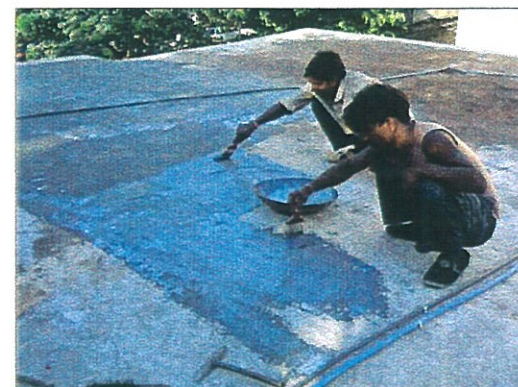
Application of polymer modified cement layer over prepared roof surface
