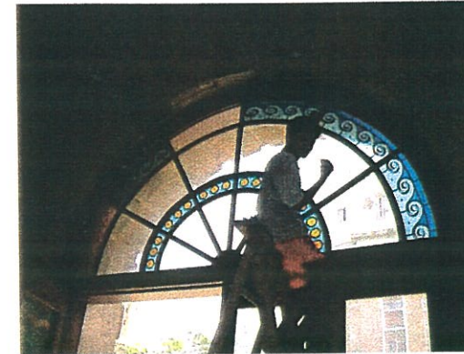
Stained glass panels being placed in position.
