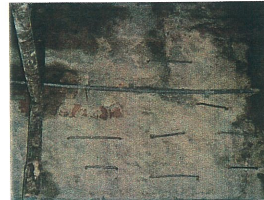
Vertical structural crack in the partition wall between the central hall and the rooms stitched with SS pins.
