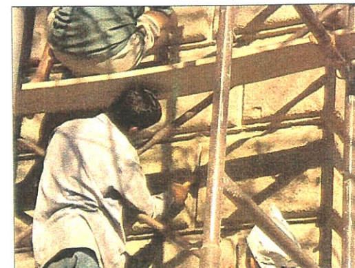
Removal of cement from recessed joints and dressed stone surfaces
