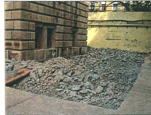
Layer of P.C.C. and murram around the structure was much deeper than estimated.
