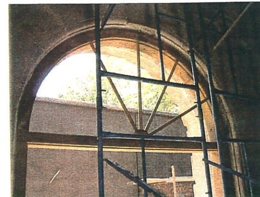
Installation of timber frame
