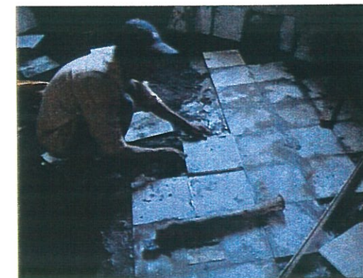
Laying of Kotah stone flooring in diagonal pattern (in the rooms).
