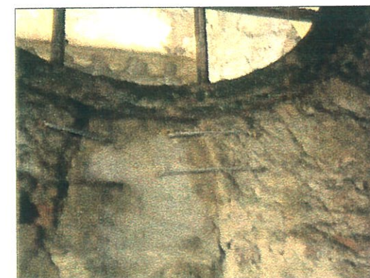
SS pins placed across opened joints of voussoirs of the ox-eye window.
