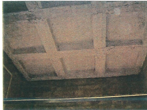
COFFERED SLAB OF CENTRAL HALL BEFORE RESTORATION
