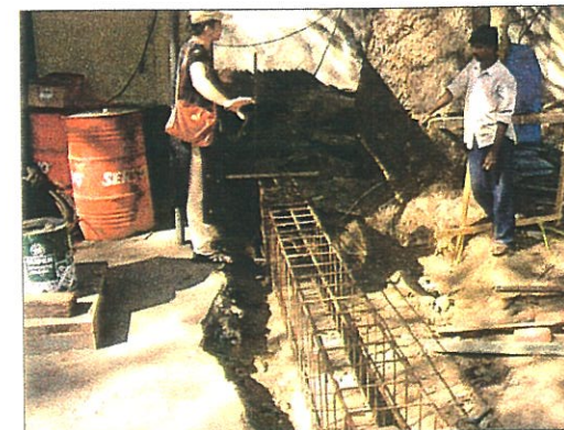
R.C. Beams laid across the massive tree roots to support the masonry above
