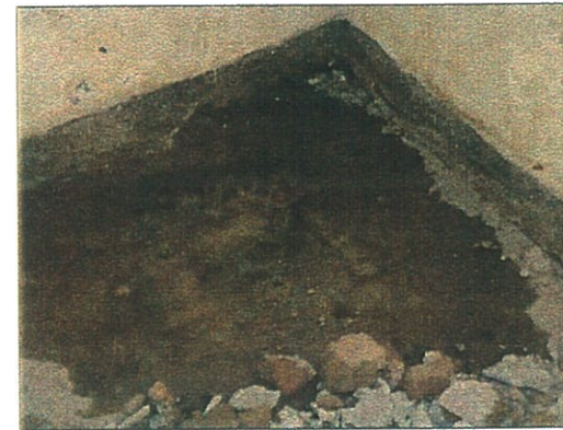
Shahbad stone flooring explored in the rooms was fairly damaged and uneven.
