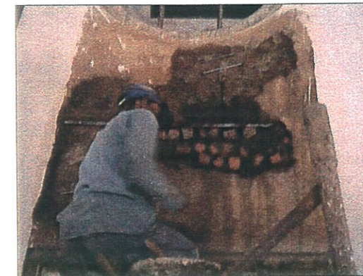
Consolidation / Leveling of masonry surface with brick bats in lime mortar.
