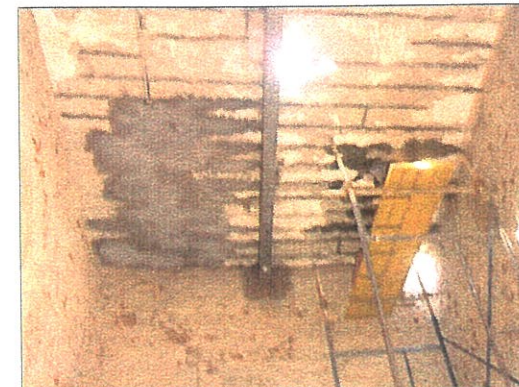
ISMB 250 introduced to strengthen the existing slab and prevent further sagging.
