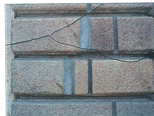
Deep recessed joints in stone masonry filled with cement mortar (before restoration)
