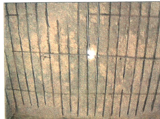
Reinforcement of slab exposed after removal of loose concrete cover
