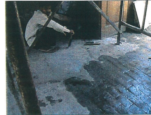
Cleaning the cementitious layers off the cobbled floor was a painstaking task.
