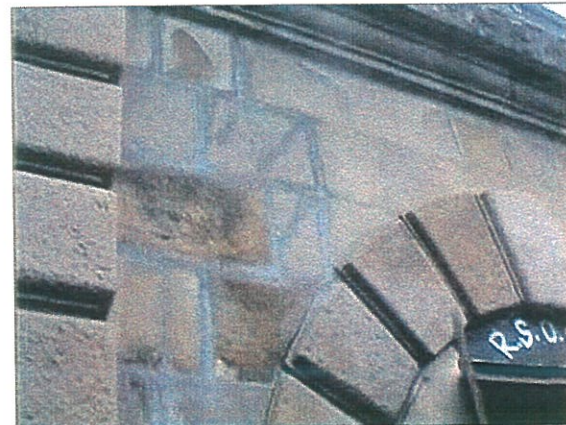
JOINTS AND CRACKS IN ASHLAR MASONRY SEALED WITH CEMENT
