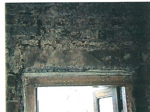
Stone lintels above square headed openings in the rooms.
