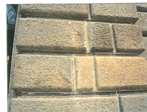
Stone masonry after removal of cement accretions and cleaning.
