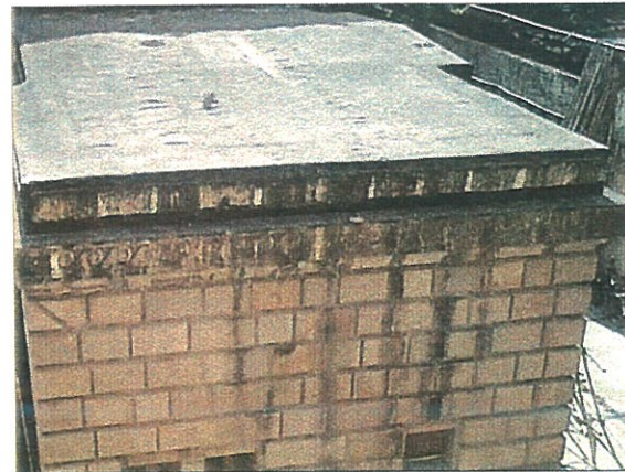
FACADE SOILED WITH STAINS (DUE TO WEATHERING AND TAR FROM THE TAR FELT ROOF PROTECTION) BEFORE RESTORATION
