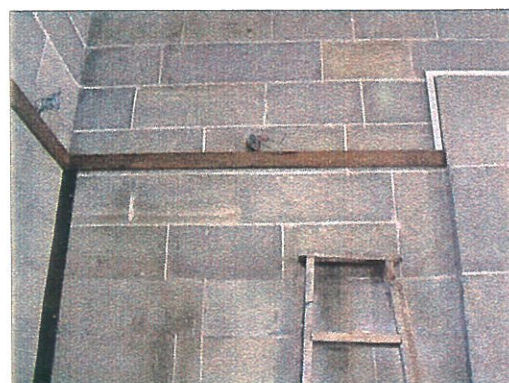
Masking of electrical wiring with polished wood capping casing.
