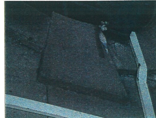
Structural crack in partition wall between the hall and the rooms caused due to insertion of steel beam. Note the disintegration of the stone voussoir at the beam.
