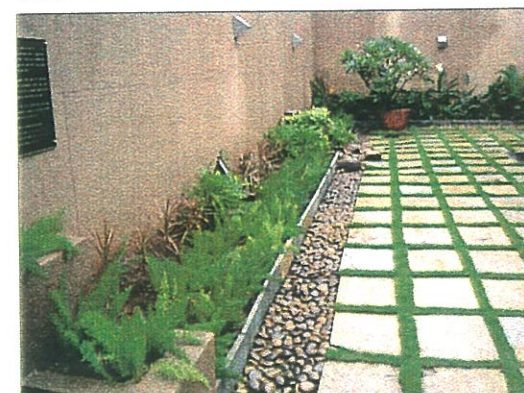
Grass jointed shahbad tile paving edged by the French drain topped with a layer of pebbles
