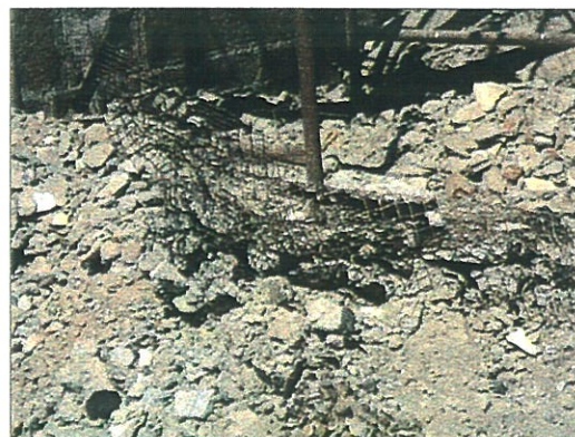
Layers of concrete (with wire mesh reinforcement) removed from roof slab
