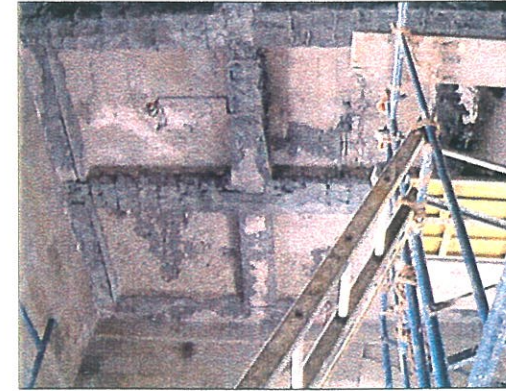
Strengthened coffered slab before application of Polymer modified mortar
