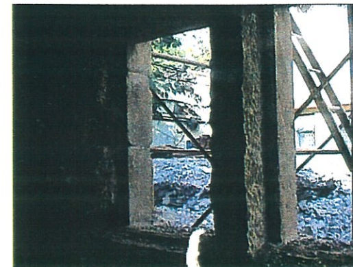
Window frames and shutters dismantled – the dressed stone surrounds exposed.
