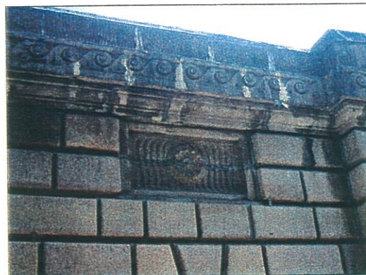
Decorative façade features damaged by soiling / tar stains and cement application (before restoration)
