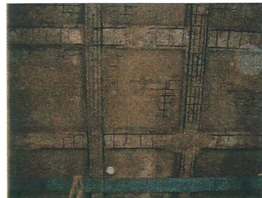
Reinforcement of coffered slab exposed after removal of Loose concrete cover.
