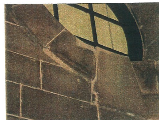
Voussoirs of the ox eye window restored with lime mortar. The structural cracks were stitched with SS pins.
