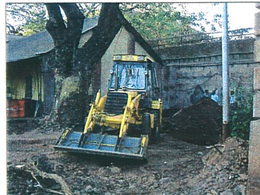
Removal of debris between the structure and the tree after demolition of the shed
