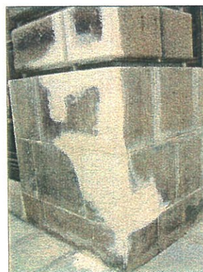
Plastic Repairs using lime mortar in locations where part stones had spalled
