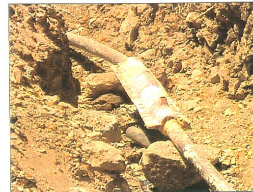
Junction at LT cable after it was realigned with an extension.
