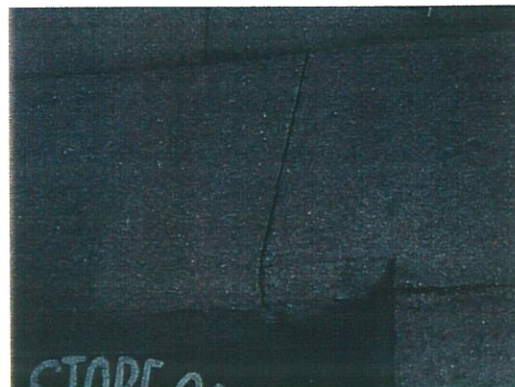
Structural crack in partition wall between the hall and the rooms caused due to insertion of steel beam. Note the disintegration of the stone voussoir at the beam.
