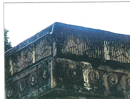
Cornice and frieze bands soiled by tar stains and weathering
