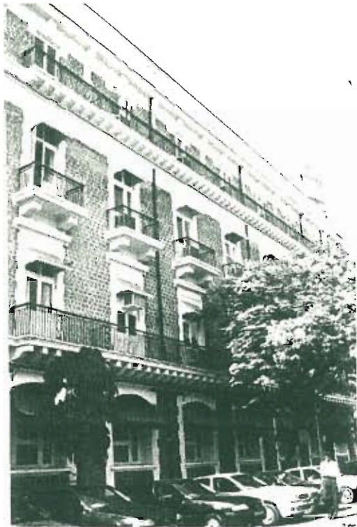
The grand hotel has painted some of its stone, given a protective coat to stone and done re-pointing using epoxy/m seal which is detrimental to fabric.
