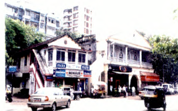
Structures of the Buffer Zone
