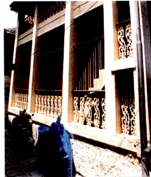
Stonework plinth covered over in plaster
