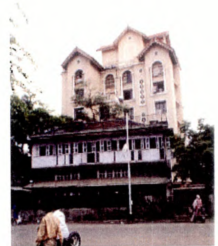
Peripheral Zone along Hill Road
