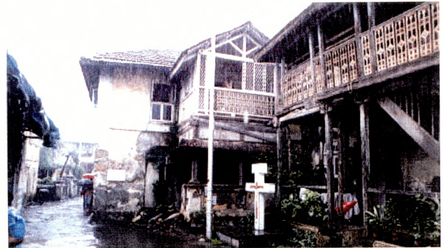
Typical meandering street
