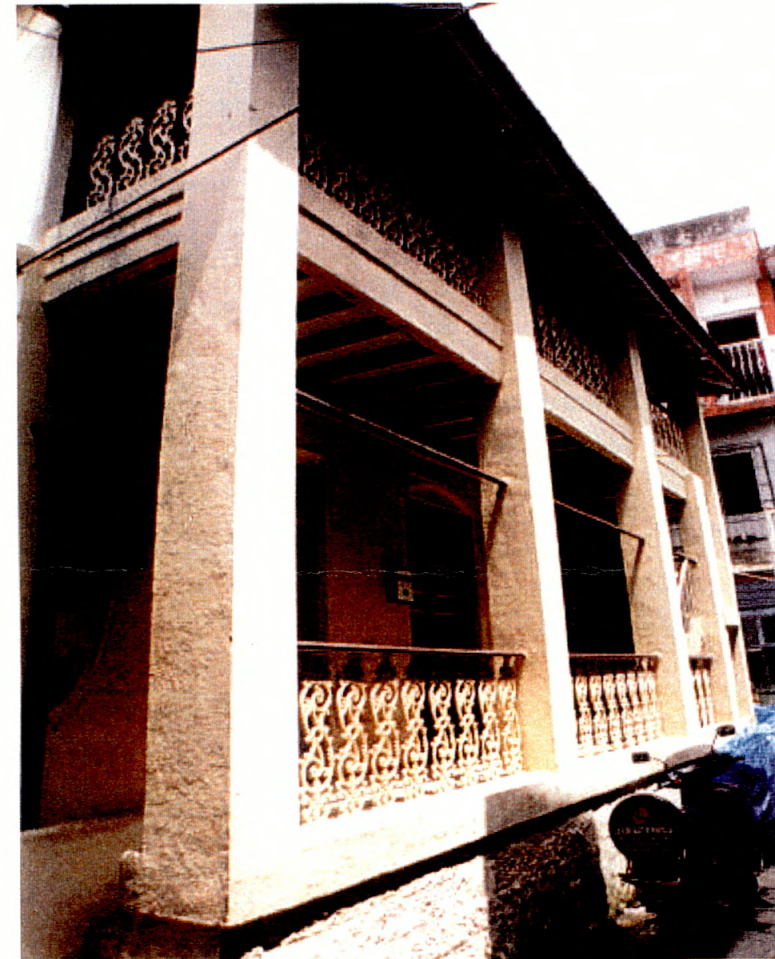
Sensitive structural alterations in concrete
