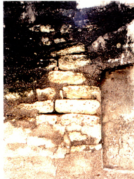
Effect of cement plaster on limestone
