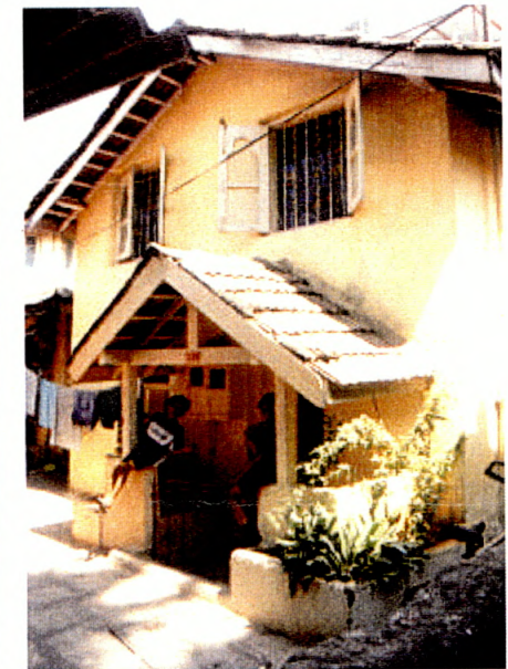
Traditional tiled roofing on wooden batters
