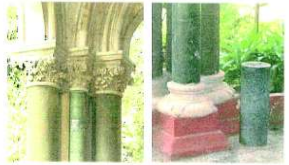
Restoration of the Convocation Hall: Dutchman Repair
