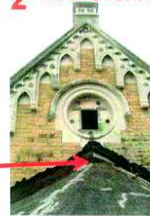
Stairwell masonry in need of pointing
