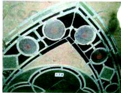
Above From Left: Panel with lead came eaten by squirrel; During Bench Repair; Panel After repair of lead came
