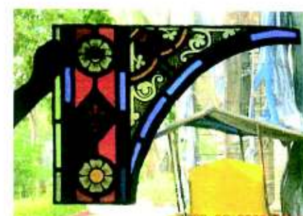
Above From Left: Panel with lead came eaten by squirrel; During Bench Repair; Panel After repair of lead came
