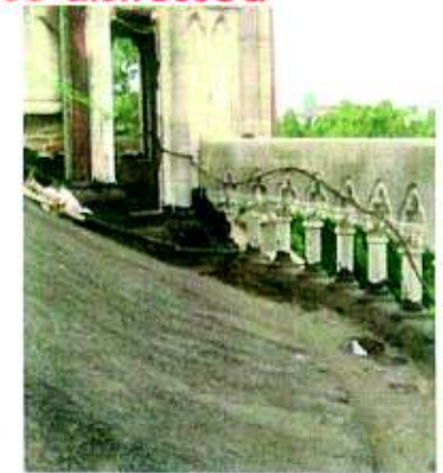
Stairwell masonry in need of pointing
