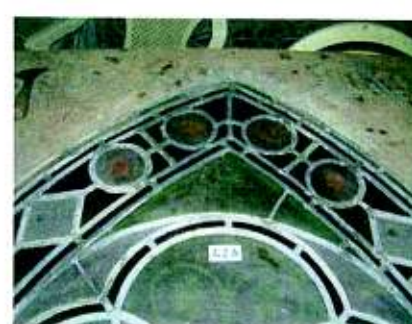
Above From Left: Panel with lead came eaten by squirrel; During Bench Repair; Panel After repair of lead came
