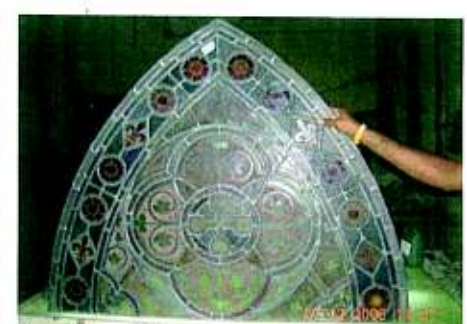
Above From Left: Panel with lead came eaten by squirrel; During Bench Repair; Panel After repair of lead came
