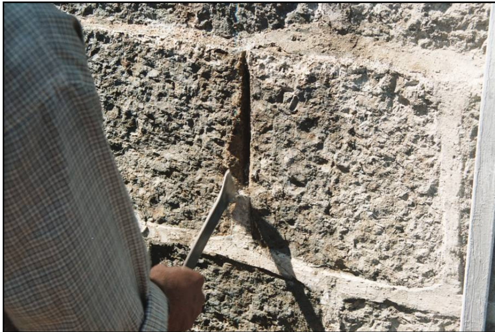
Raking out weakened jointing mortar and flushing out loose mortar
