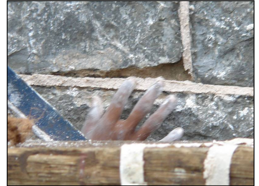
Re-jointing and re-pointing with lime mortar
