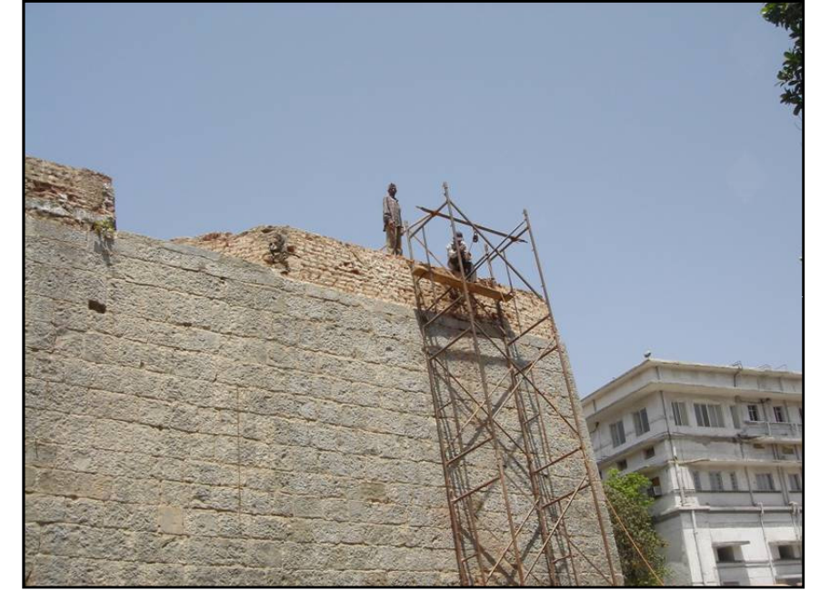
Battlements on the Bastion 3 in brick work
