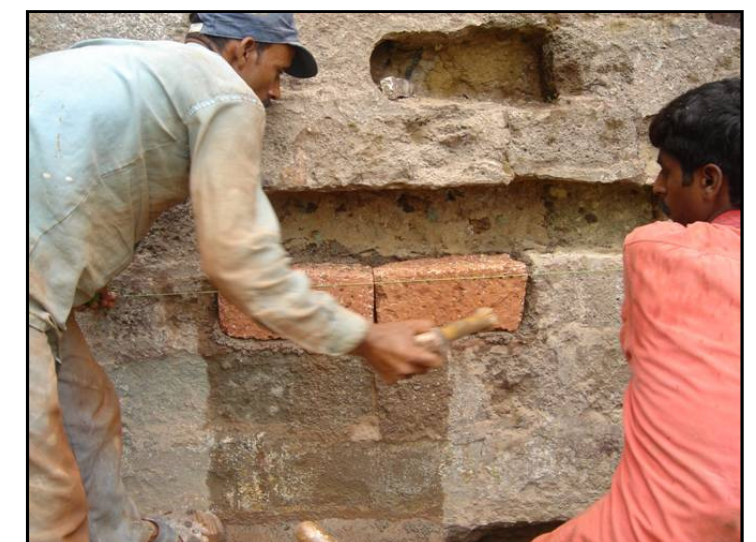
Stone replacement in process
