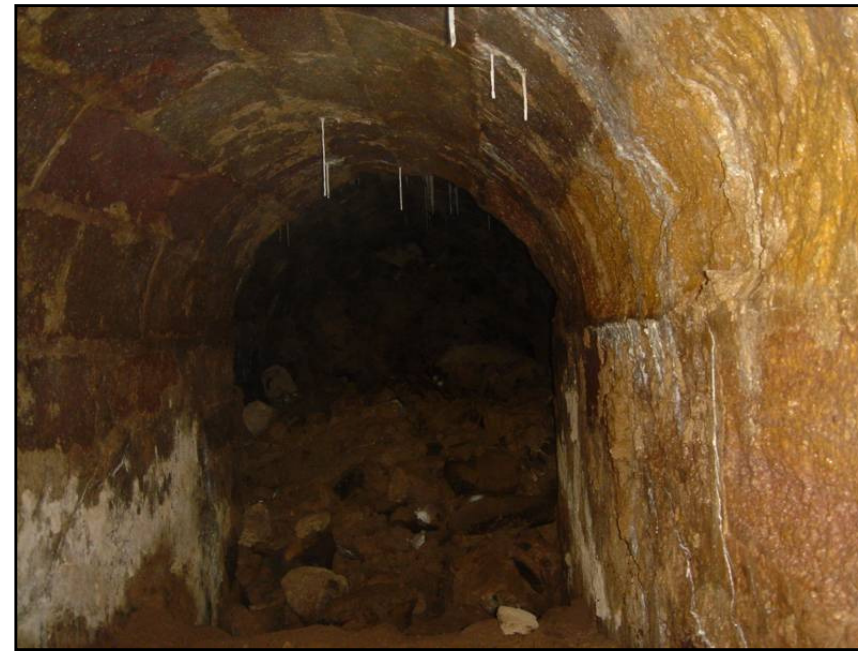
During carrying out the process of stone replacement in Curtain B, this passage tunnel (1.5m wide & 1.2m tall) has been unearthed. It has been decided to undertake further research subsequent to which further excavation and restoration work may be carried out.
