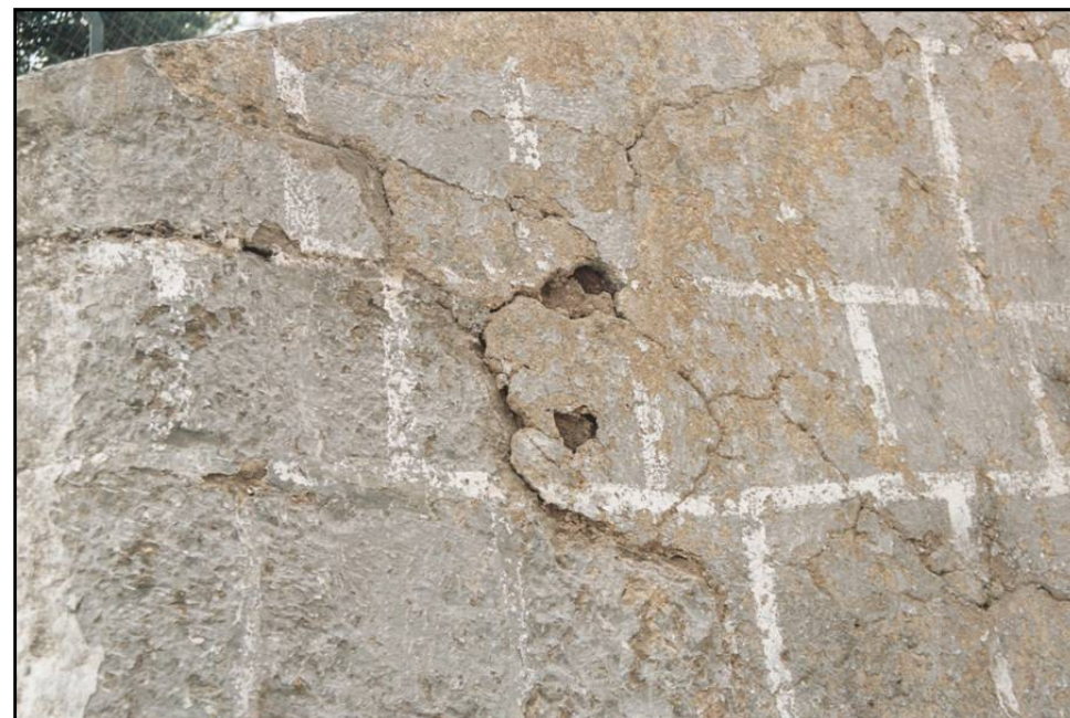
Condition prior restoration – accretions of cement plaster
