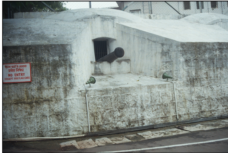
Condition prior restoration – accretions of cement paint
