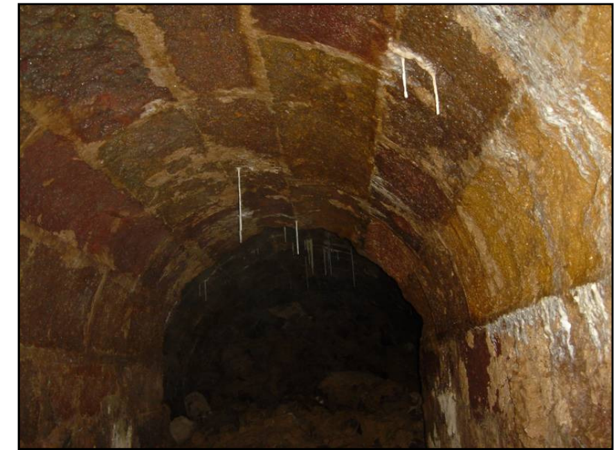
During carrying out the process of stone replacement in Curtain B, this passage tunnel (1.5m wide & 1.2m tall) has been unearthed. It has been decided to undertake further research subsequent to which further excavation and restoration work may be carried out.
