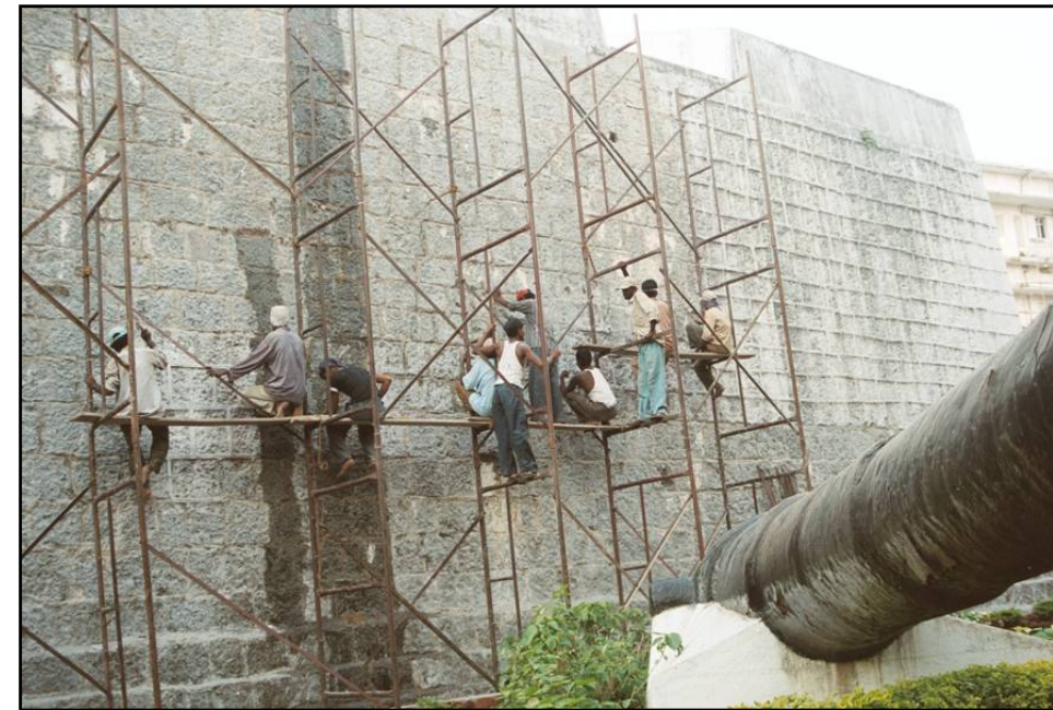
Gentle tapping to remove paint accretions
