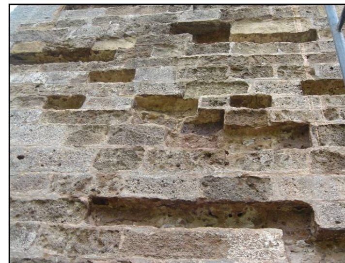
Stone replacement in process
