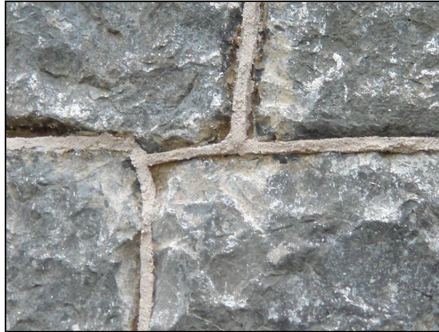
Re-jointing and re-pointing with lime mortar
