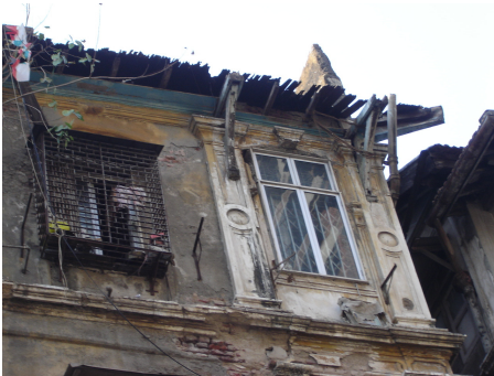
CONDITION OF OPENINGS
