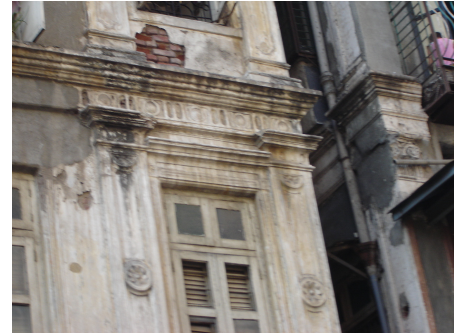
DETERIORATED ARTICULATIONS
