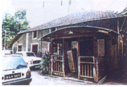
BUILDING NO. 47 E
