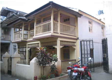
DIAS HOUSE / BUILDING NUMBER 35
