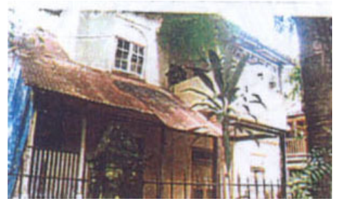
BUILDING NUMBER: 33 / ASSISI MANSION
