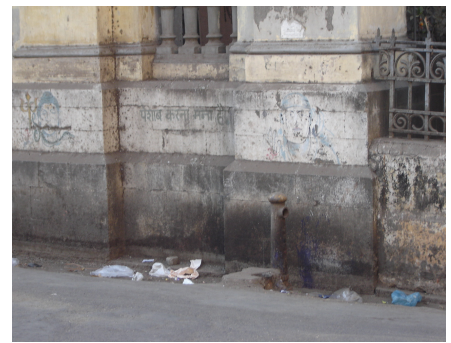
VIEW OF A PLINTH
