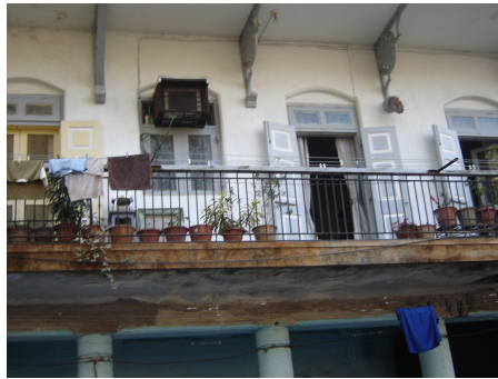
VIEW OF AN OPENINGS & BALCONY
