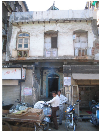
BRICK MASONRY STRUCTURE
