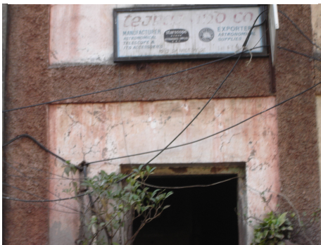
CONDITION OF WALLS
