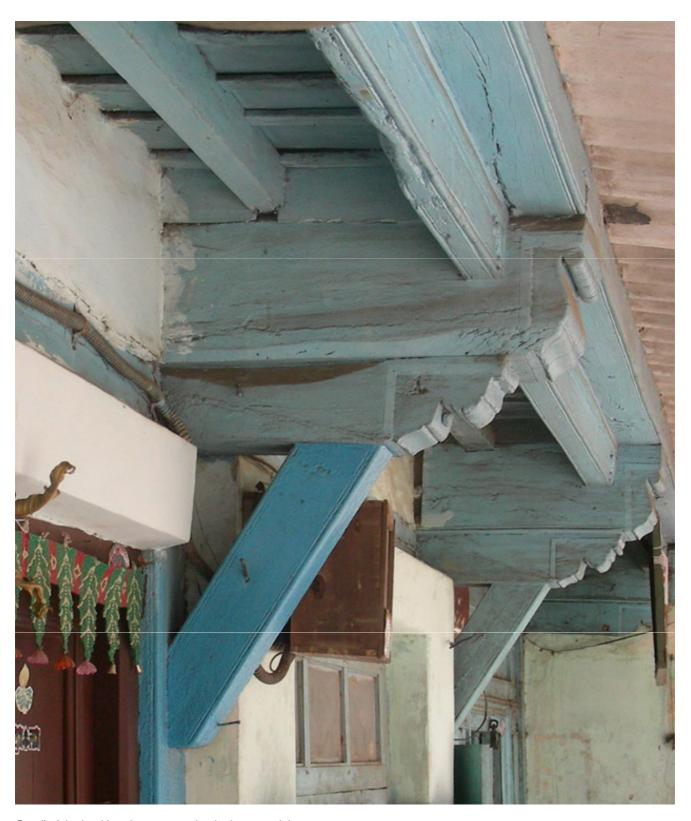
Detail of the load bearing construction in the verandah
