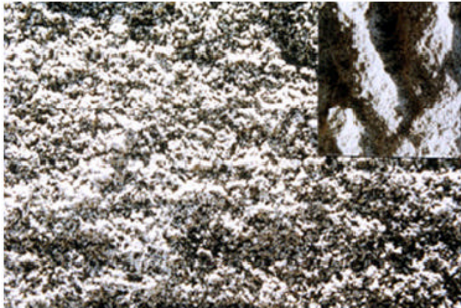
Figure 11: Erosion of limestone from wind, aerosol effect of sea water, leading to growth of microbiological activity.
