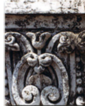
Figure 16: Calcareous stones have a hard crust on the surface. The physical and the chemical properties of the crust and the stone are different. The crust has higher density, lower permeability to water and total or partial substitution of calcium carbonate by gypsum. Variations in volume and thermal expansion of the layer and stone lead to exfoliation of the crust.
