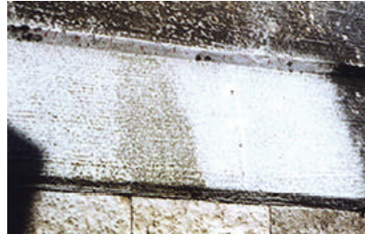
Figure 30: On site cleaning to test the appropriate method
