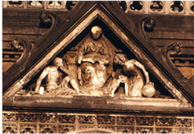
Figure 12: Loss of detail as a consequence of erosion of limestone.
