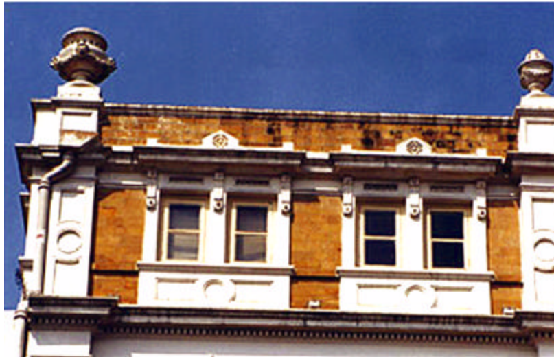
Figure 38: Recurrence of soiling after cleaning
