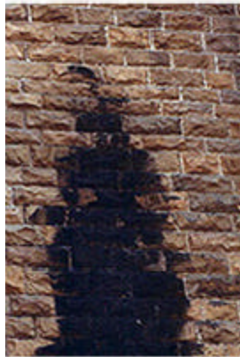
Figure 14: Soiling pattern governed by the architectural detail. The darker masonry surface is due to the water thrown out of the spout.
