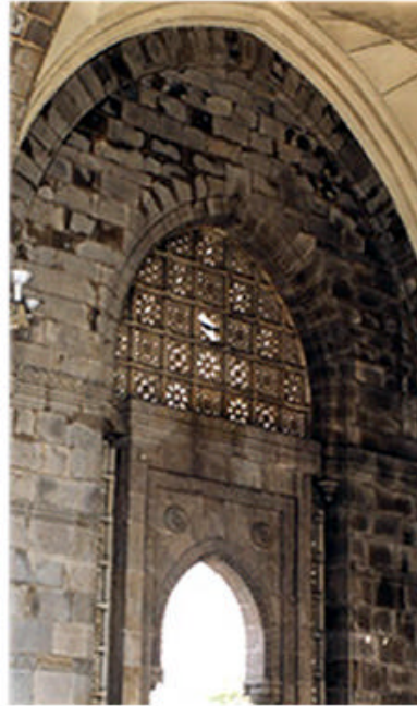
Figure 6: Water is involved in most types of stone decay. Here the penetrating damp is trapped in the masonry as can be seen by.... Hard pointing causes the moisture to evaporate from the stone surface causing deposition of salt and consequently its decay. Soft pointing is recommended to minimize decay of stone as the pointing can be periodically renewed
