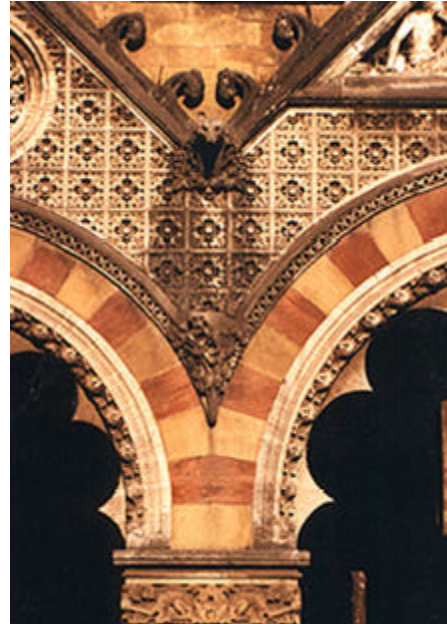
Figure 21 : The use of limestone in buildings is primarily decorative element, as a carved and lending richness, opulence and affluence to the facades of the building. Limestone remains clean but gets roughened wherever rain washing is regular. The sheltered zones collect dirt and often a sulphate crust is formed. Maintenance could significant overcome this problem in sheltered zones.
