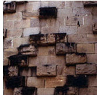
Figure 15: Texture location and properties of individual stone contributes to differential soiling. Rough surfaces facilitate deposition.
