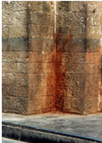
Figure 23: Pan staining of masonry
