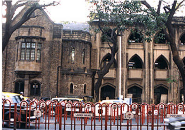
Figure 27: The differential soiling is due to different material. The portion of the building on the left is Kurla basalt and on the right is cast stone. Soiling can add substantially to the structure and architectural value of the building. A case for not cleaning.
