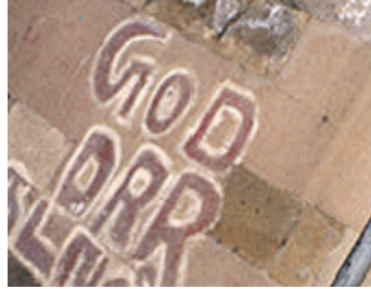
Figure 24: (b) In the case of paints, the pigment solvent which is absorbed in the pores is very difficult to remove.
