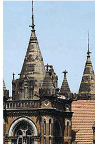
Figure 7: The lighter side of the conical limestone roof indicates the direction of wind and rain, the leeward side left being soiled and infected with \text{CaSO}_4 encrustations
