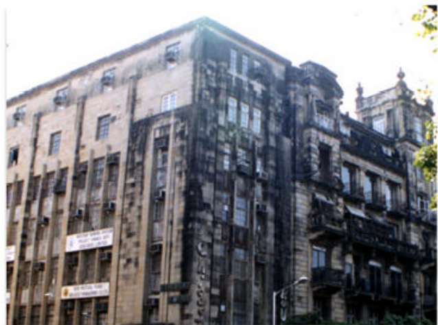
Figure 13: Facades abutting major traffic arteries tend to be more soiled than sheltered facades.
