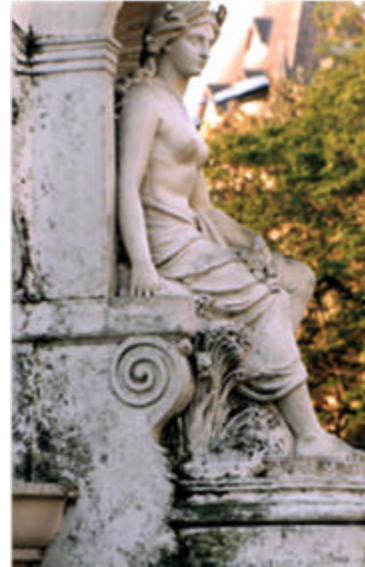
Figure 18: Algal growth on lime washed stone work
