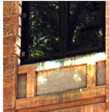
Figure 22: Metal staining the masonry (a) iron stains (b) copper stains
