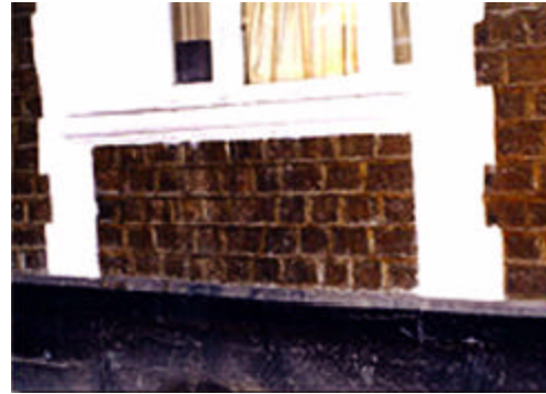
Figure 34: Application of improper surface protective systems which prevent breathing of the masonry.
