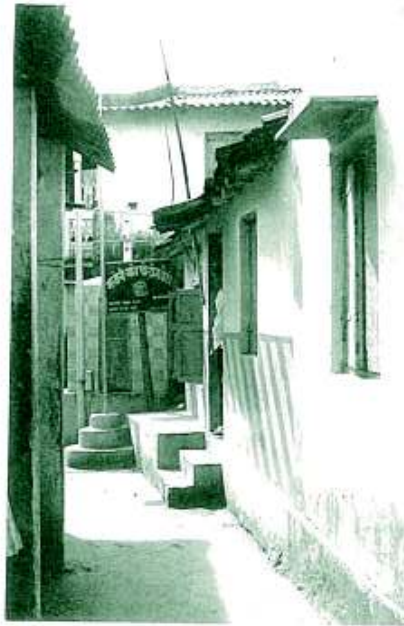
Manori Police Station Source: RCACC (2002)
