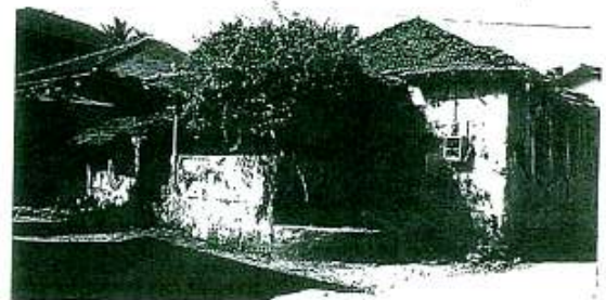
Dilapidated house, Gorai Source: RCACC (2002)
