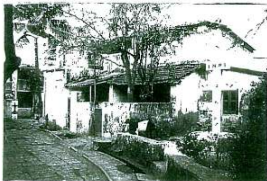
Structure with minor transformation Source: RCACC
