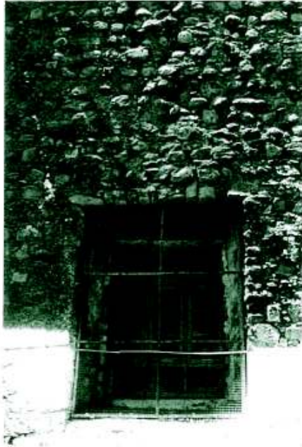
Lintel in coursed rubble masonry, Erangal Source: RCACC (2002)
