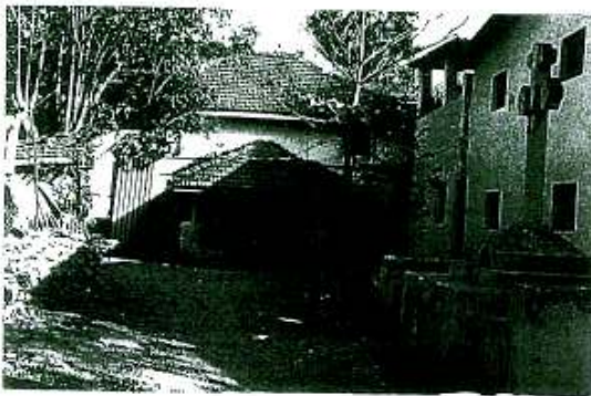
Retained building in Culvem Source: RCACC (2002)
