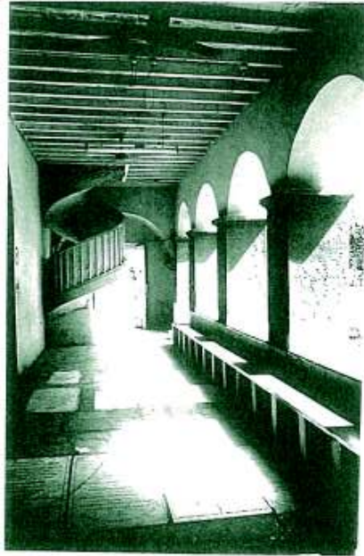
Timber spiral staircase and timber Flooring in Manori Church Source: RCACC (2002)
