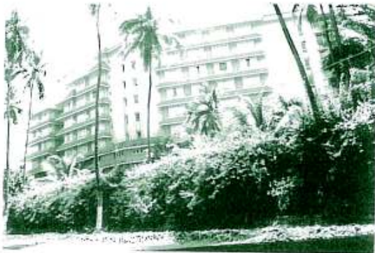
Hotel in the designated NDZ area, violating height controls Source: RCACC (2002)
