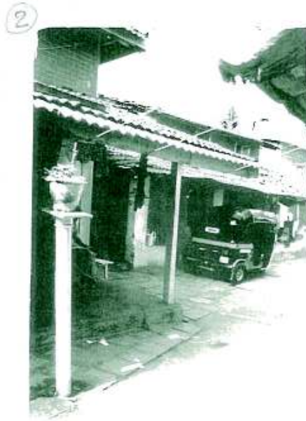
Bhandari house cluster, Aksa Source: RCACC (2002)
