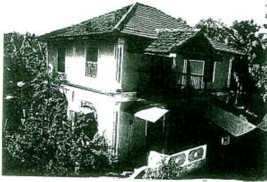
Retained building in Culvem Source: RCACC (2002)
