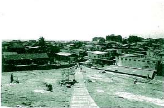
Haphazard Gaothan expansion, leading to environmental degradation in Manori Source: RCACC (2002)
