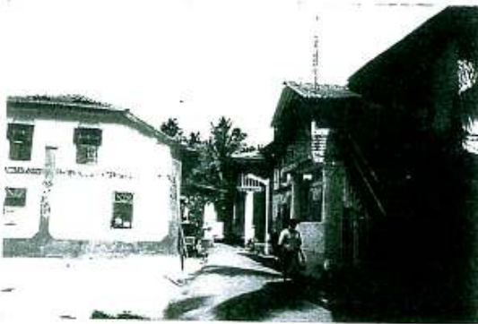
Structure with Minor Transformation Source: RCACC
