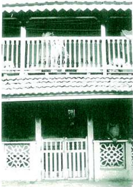
Timber turned wooden railing in verandah, Madh Source: RCACC (2002)
