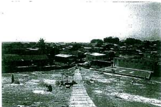
View of South Gaothan Madh Source: RCACC
