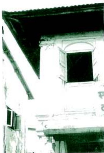
Window and plaster details, Manori Source: RCACC (2002)
