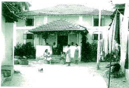
East Indian house, Manori Source: RCACC (2002)
