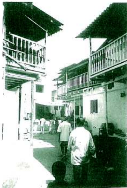
Koli Housing Block, Manori Source: RCACC (2002)
