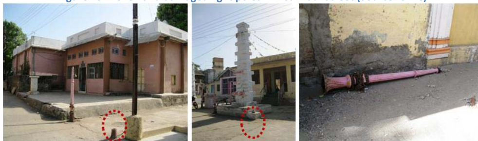
Figure 25 Broken and damaged light poles in Deulwadi Street (Source: UMC)
