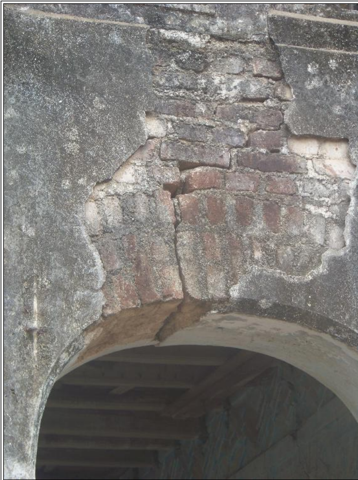
Image Title: Raigad Jilha Macchimar Sangha Ltd. Image Type: Top-View Reference: Cracked arches in need of structural repairs
