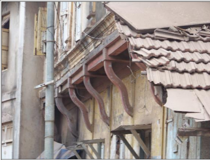
Image Title: Vajan Mape Vibhag Image Type: Front-View Reference: Brackets supporting first floor Lanticevar
