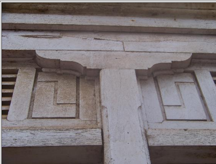
Image Title: Dali House Image Type: Top-View Reference: Wooden column with brackets
