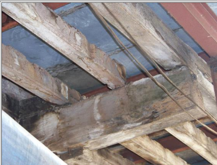
Image Title: Modi Wada Image Type: Top-View Reference: Decayed wooden members of Balcony
