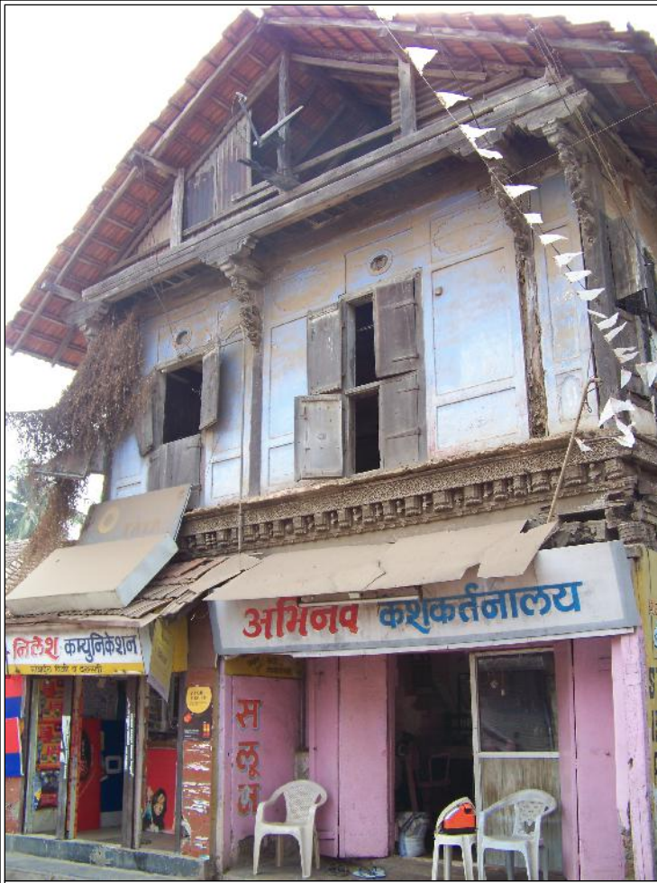
Image Title: Modi Wada Image Type: Front-View Reference: Front view showing dilapidated attic and ground level with incongruent additions
