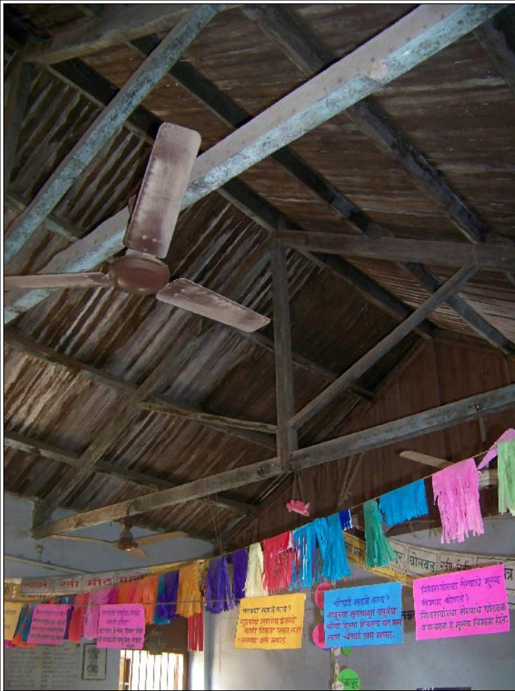
Image Title: Haldavanekar School Image Type: Top-View Reference: Wooden roofing trusses
