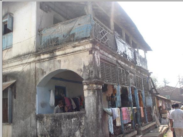
Image Title: Dabri House Image Type: Side-View1 Reference: Louvered openings acting as sun screens at ground floor of verandah
