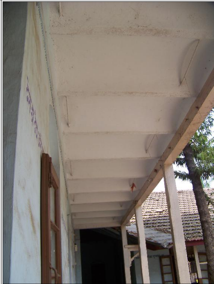
Image Title: Haldavanekar School Image Type: Top-View Reference: Projecting balcony on first floor with wooden framework
