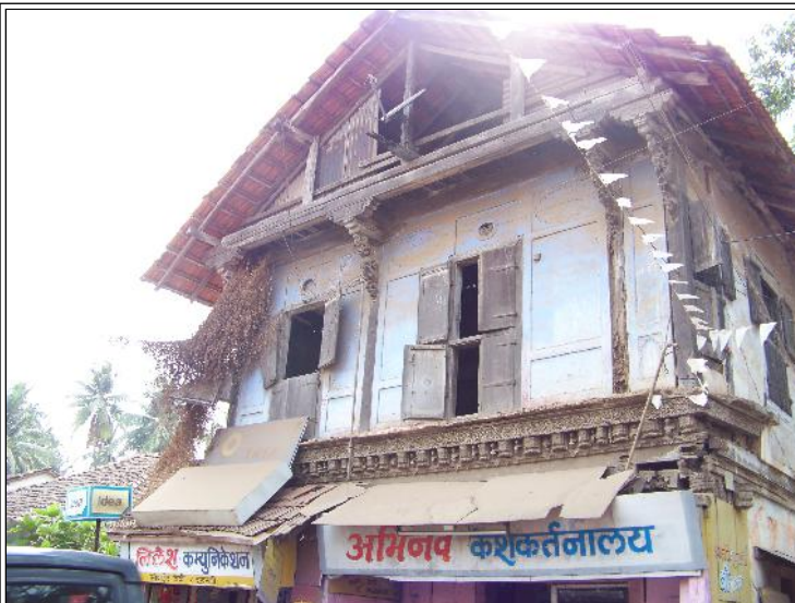
Image Title: Modi Wada Image Type: Front-View Reference: First floor showing wooden brackets and acarved cornice at junction of ground and first floor
