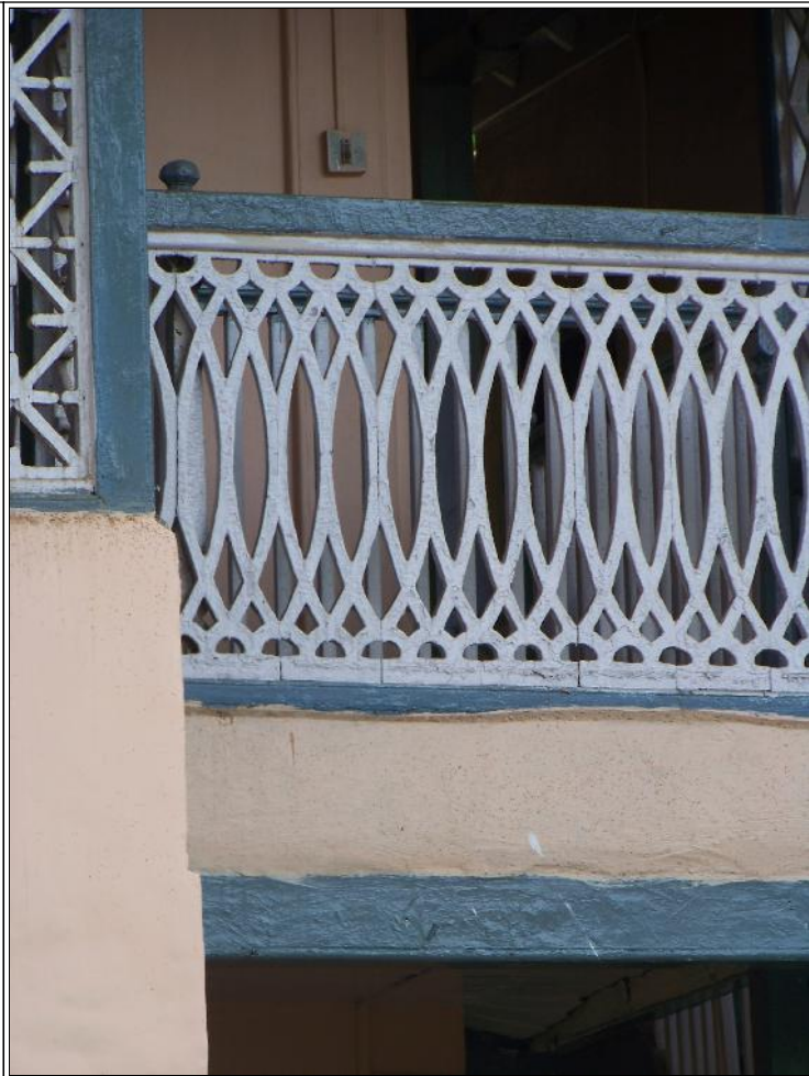
Image Title: Geomagnetic Observatory Image Type: Top-View Reference: Cast iron railing on First Floor
