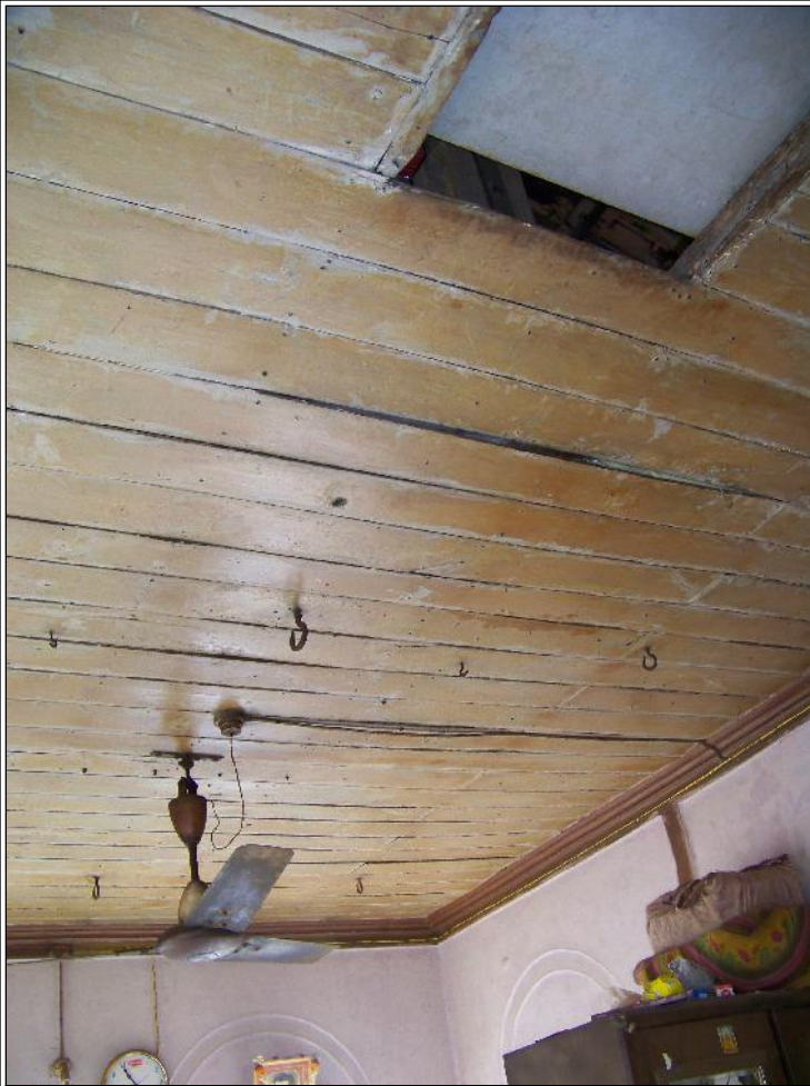
Image Title: Modi Wada Image Type: Top-View Reference: Wooden False Ceiling on First Floor
