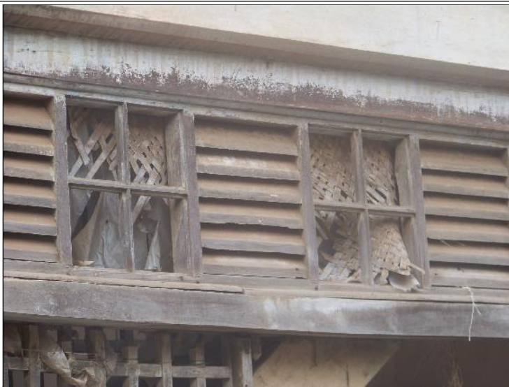
Image Title: Choule Building Image Type: Top-View Reference: Sunscreen on groundfloor verandah a feature inspired from colonial houses
