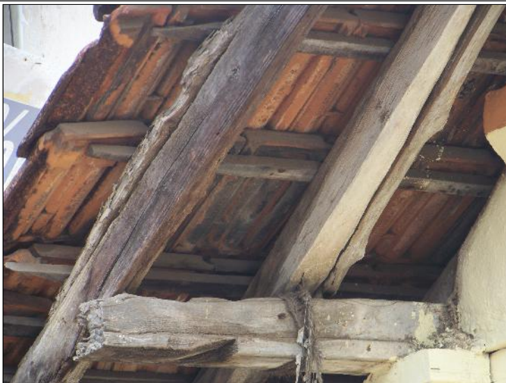
Image Title: Hanuman Mandir Image Type: Top-View Reference: Mangalore tile roofing over undressed timber members
