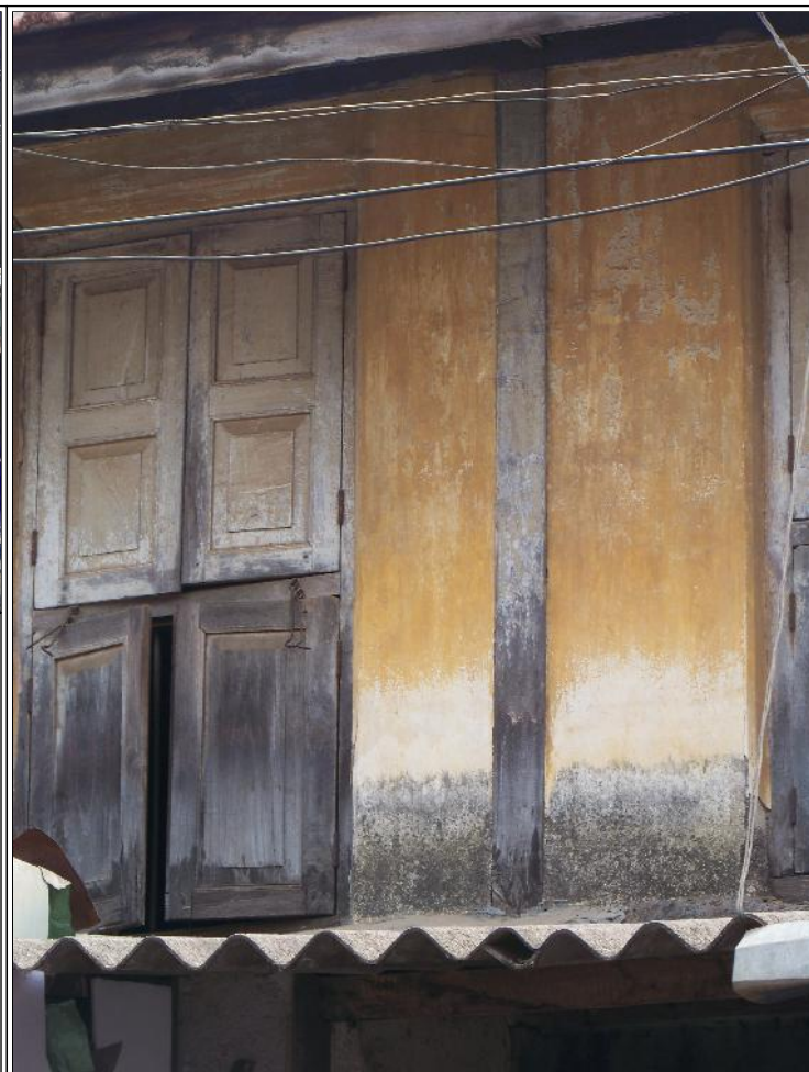
Image Title: Gujrati Mahajan House Image Type: Front-View Reference: Double shuttered windows on first floor walls show evidence of water seepage
