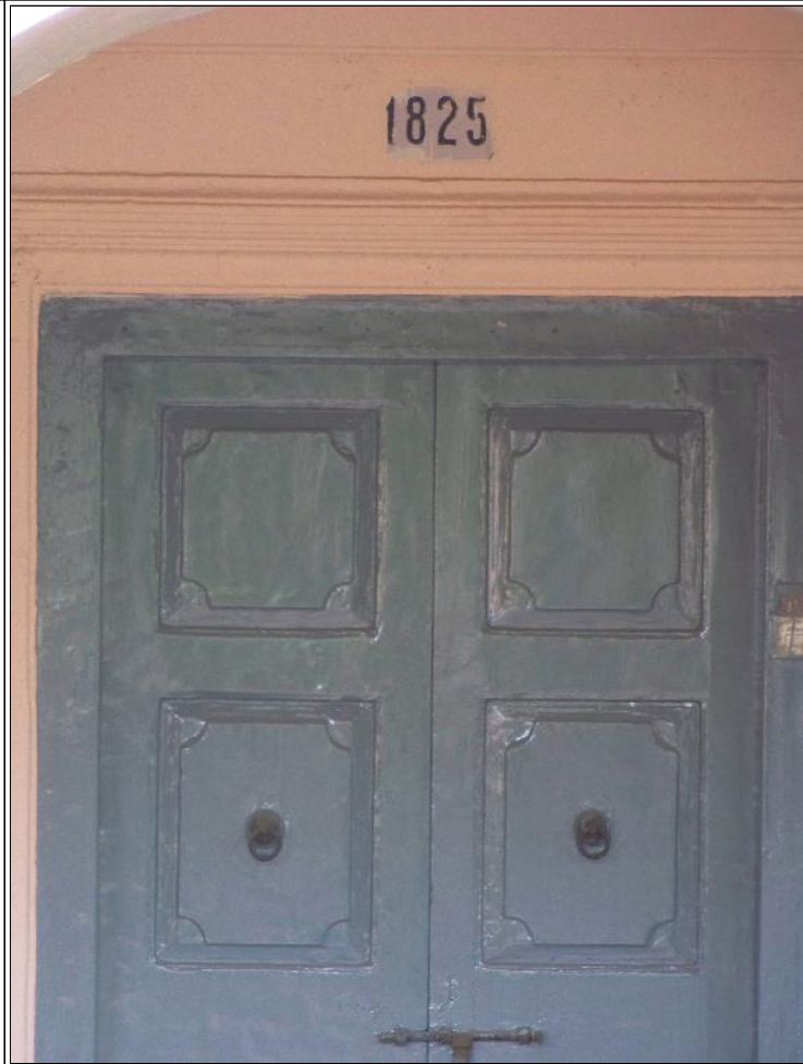
Image Title: Geomagnetic Observatory Image Type: Front-View Reference: Close up of the panelled doors with moulded jambs
