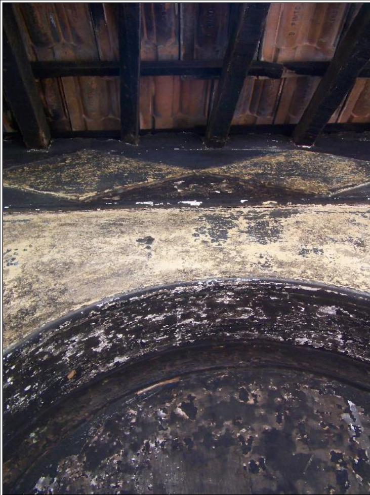
Image Title: Modi Wada Image Type: Top-View Reference: Part of wall damaged due to water
