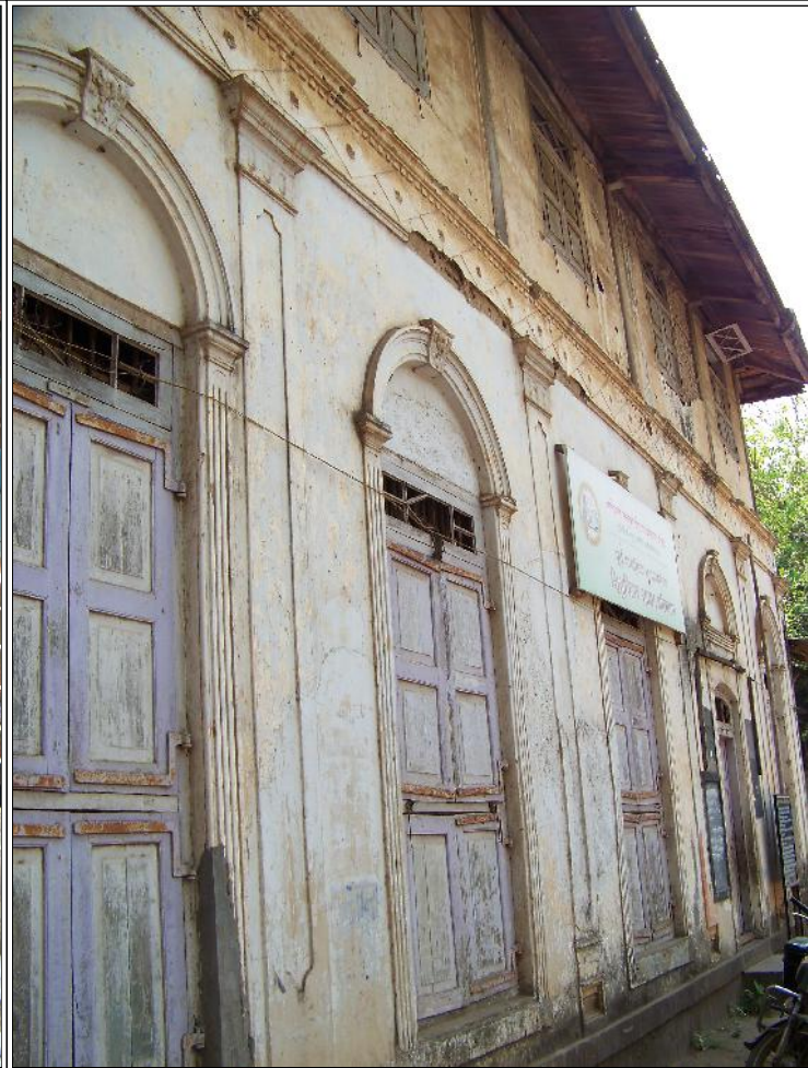
Image Title: Biwalkar Shiv Mandir Image Type: Front-View Reference: View of openings showing plaster work in cornices, Jambs and Arches
