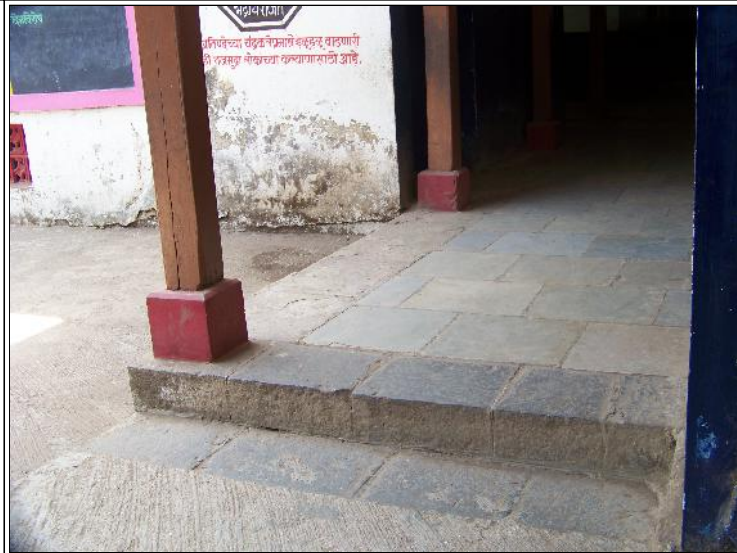
Image Title: Haldavanekar School Image Type: Front-View Reference: Columns with stone base sitting on dressed stone plinth
