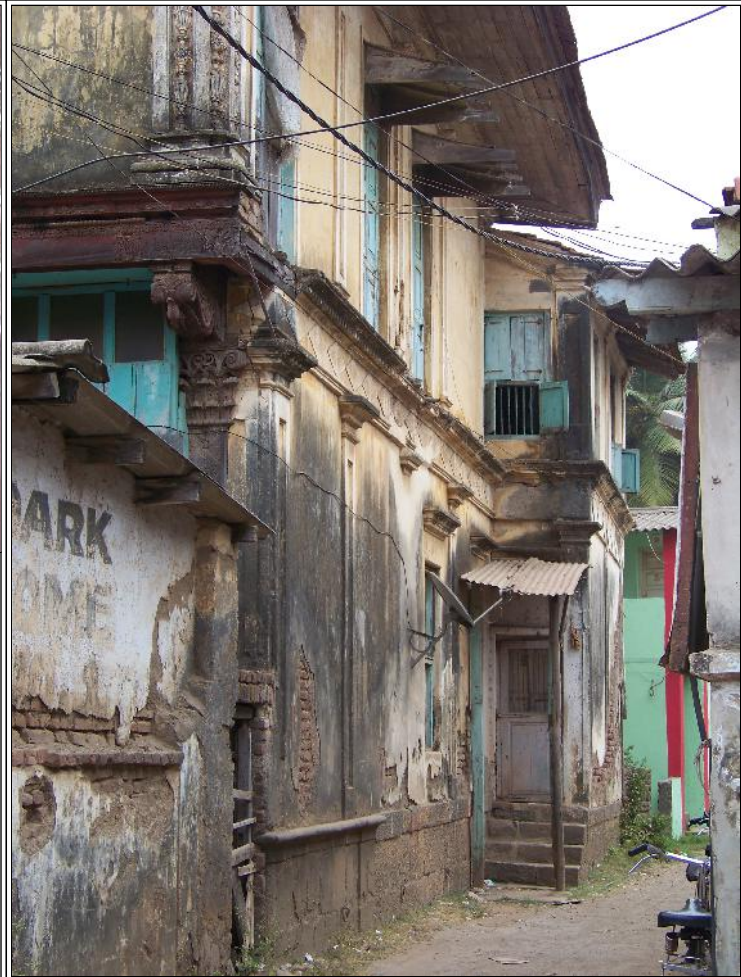
Image Title: Gurjar House Image Type: Front-View Reference: View of the sides showing plaster work and the damage caused by water
