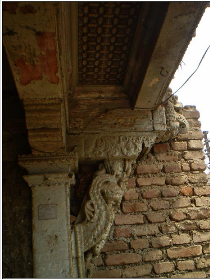
Image Title: Ganpati Mandir Image Type: Front-View Reference: Wooden column/ Bracket supporting projecting floor
