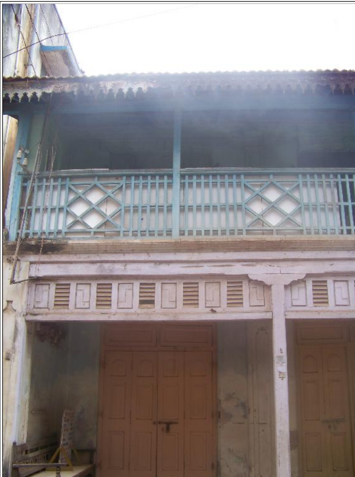
Image Title: Dali House Image Type: Front-View Reference: Front elevation of the house showing sunscreens at ground floor and the wooden railings above
