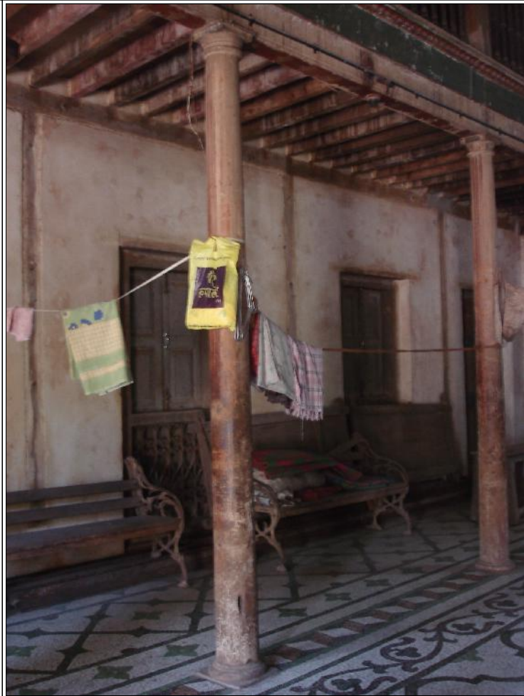
Image Title: Radha Krishna Mandir Image Type: Top-View Reference: Slender wooden Columns supporting the first floor
