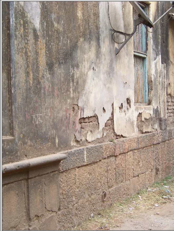
Image Title: Gurjar House Image Type: Side-View1 Reference: Detail view of plinth showing loss of plaster and damage due to water
