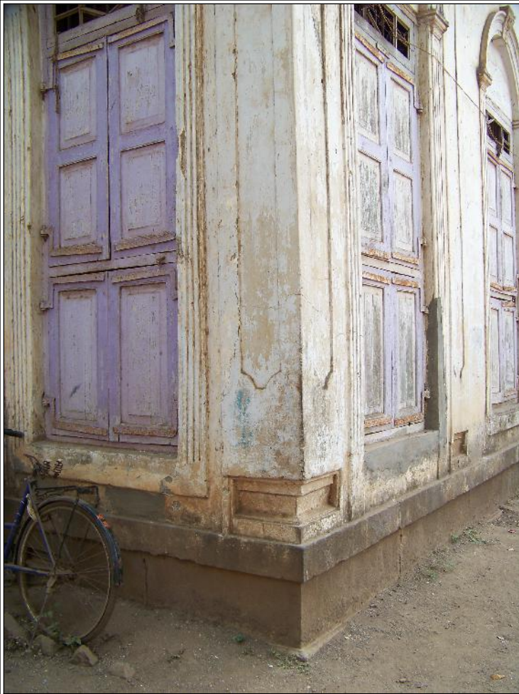
Image Title: Biwalkar Shiv Mandir Image Type: Front-View Reference: Corner view showing moulded Jambs and cornices in plaster work
