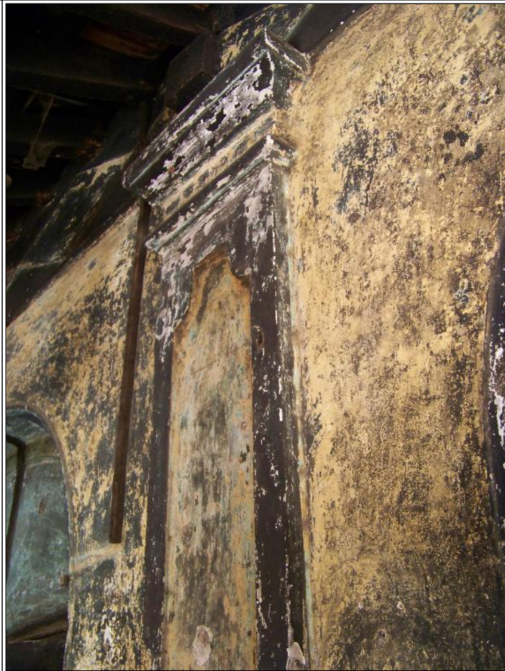
Image Title: Modi Wada Image Type: Front-View Reference: Part of wall damaged due to water
