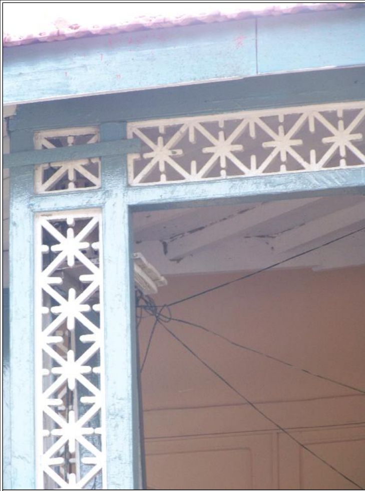
Image Title: Geomagnetic Observatory Image Type: Top-View Reference: Detail of Grill inserted within wooden columns
