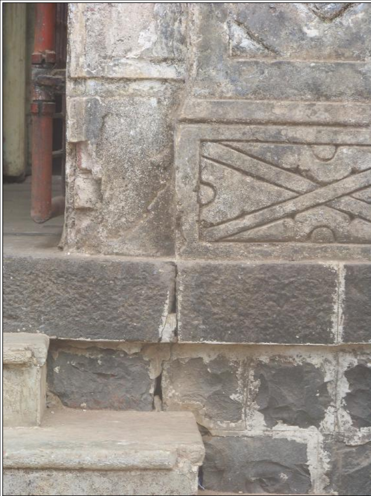
Image Title: Raigad Jilha Macchimar Sangha Ltd. Image Type: Front-View Reference: Detail view of plinth crack indicating possible differential brittleness
