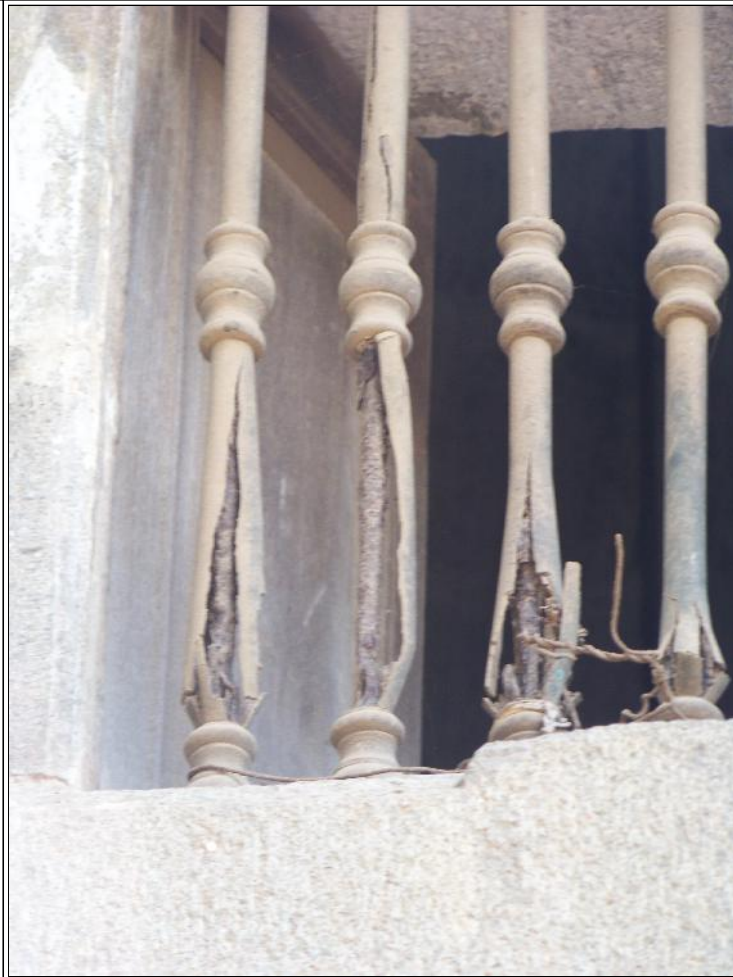
Image Title: Biwalkar Shiv Mandir Image Type: Front-View Reference: Broken Brass Grill with corroded iron core
