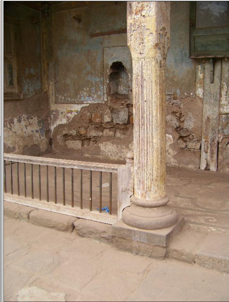
Image Title: Ganpati Mandir Image Type: Front-View Reference: Wooden column with stone base and stone floor
