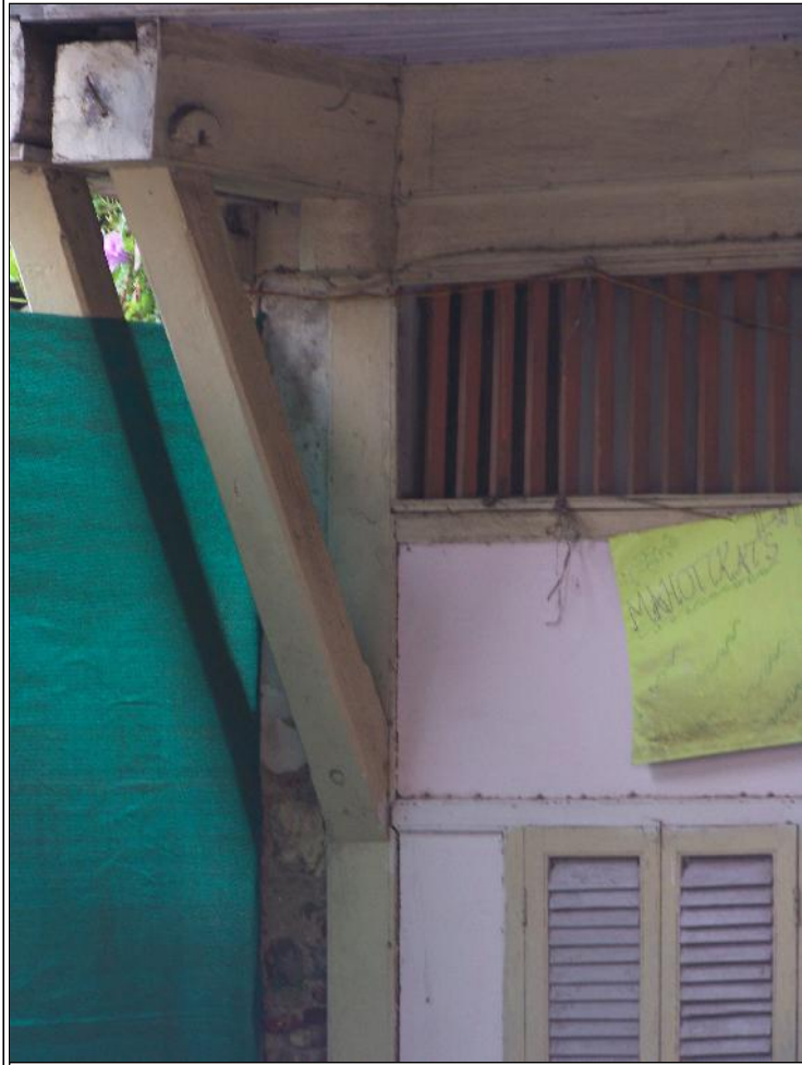
Image Title: Angre Wada Image Type: Front-View Reference: Wooden Brackets supporting balcony on the first floor
