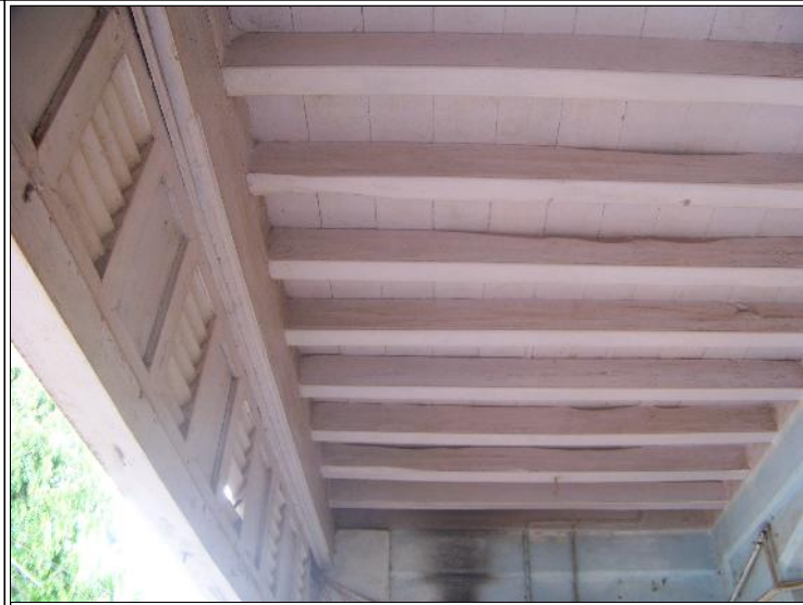
Image Title: Dali House Image Type: Top-View Reference: Wooden framework supporting the First floor
