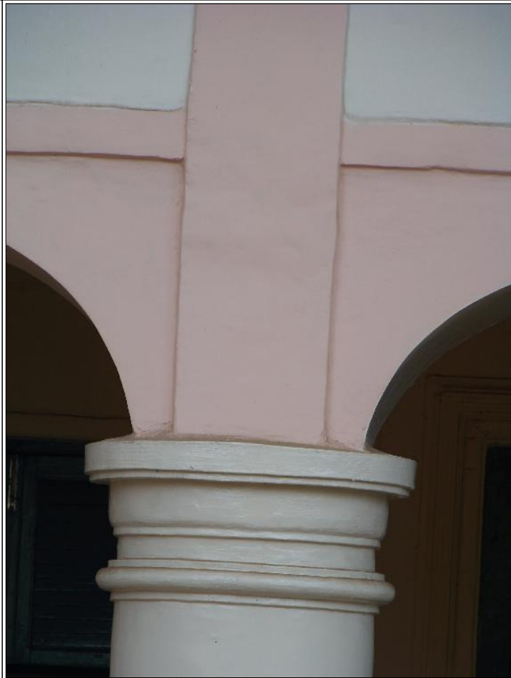
Image Title: Geomagnetic Observatory Image Type: Front-View Reference: Masonry columns with springing points of Arches
