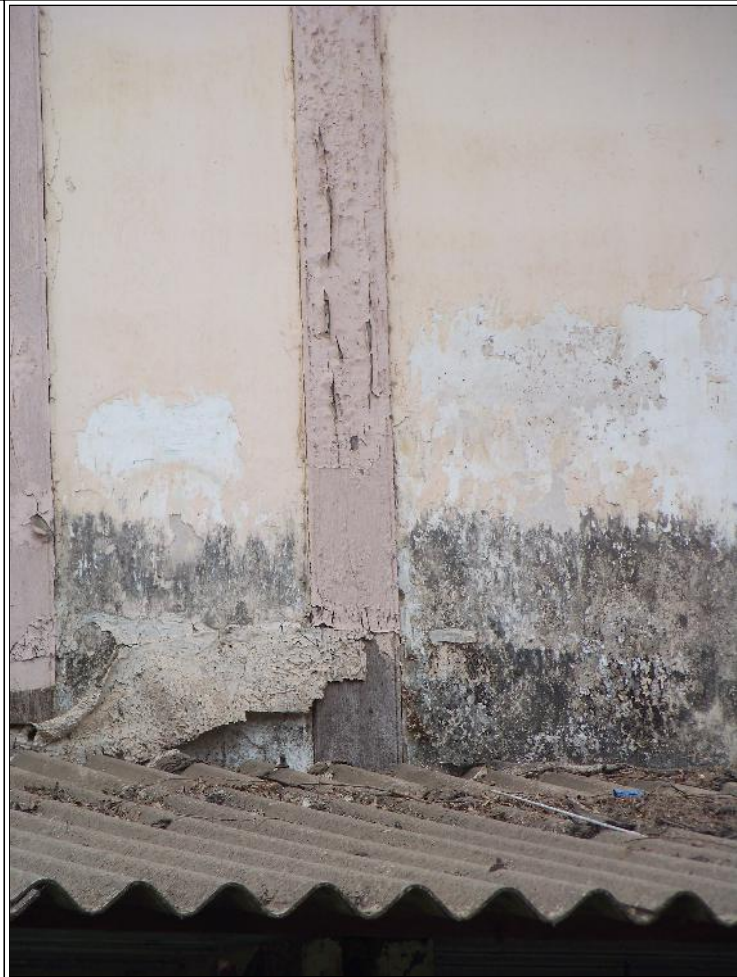
Image Title: Angre Wada Image Type: Front-View Reference: Junction of new verandah with old structure
