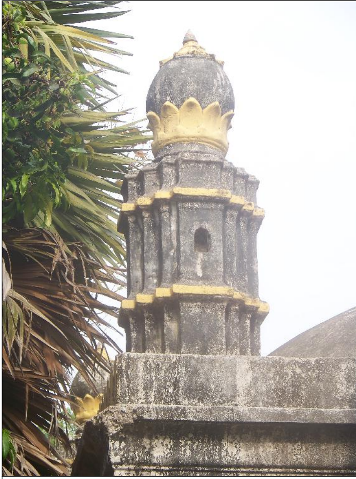
Image Title: Shriram Mandir Image Type: Front-View Reference: Brick and Lime minarets on four corners of the shikhara
