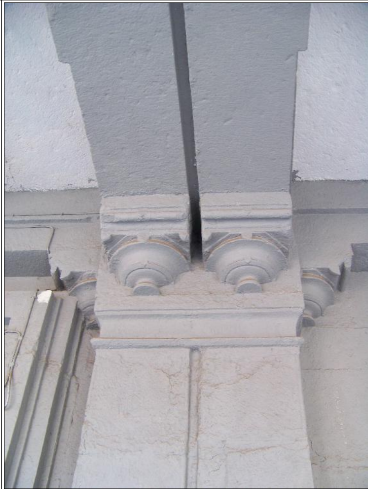
Image Title: Balaji Mandir Image Type: Top-View Reference: Inverted Bell capitals of columns in front portico
