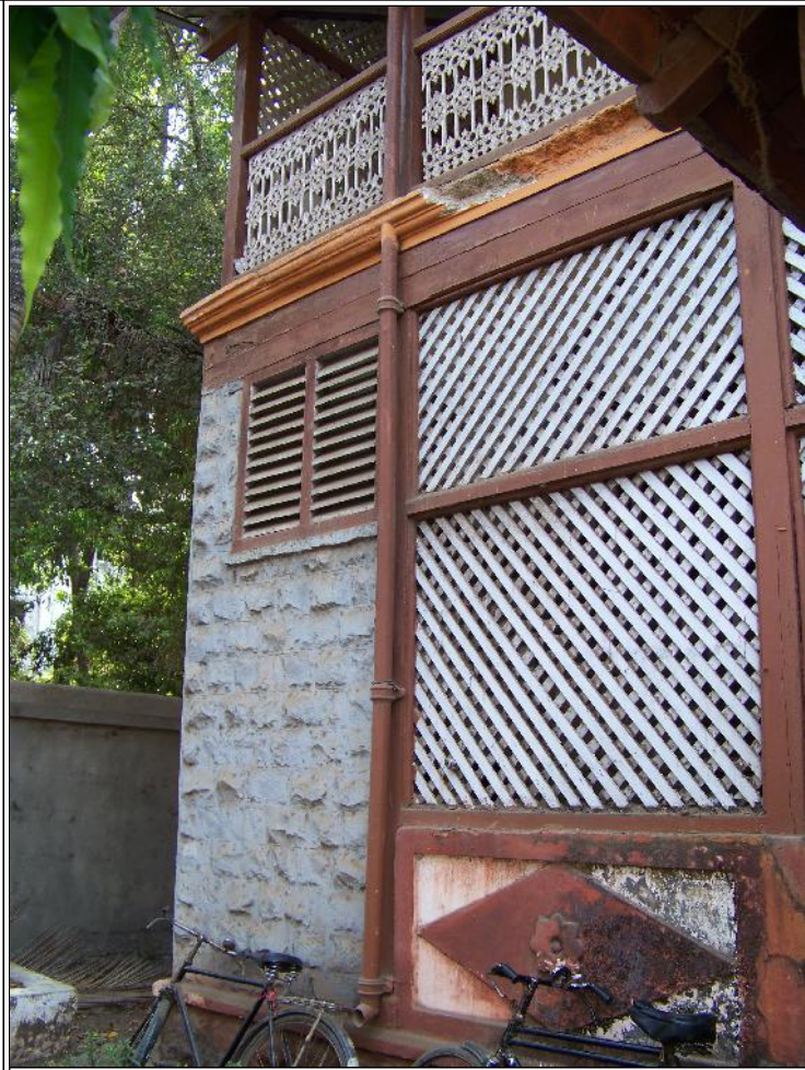
Image Title: Old Nagar Parishad Image Type: Side-View2 Reference: Wooden Jali covering Part of the Facade
