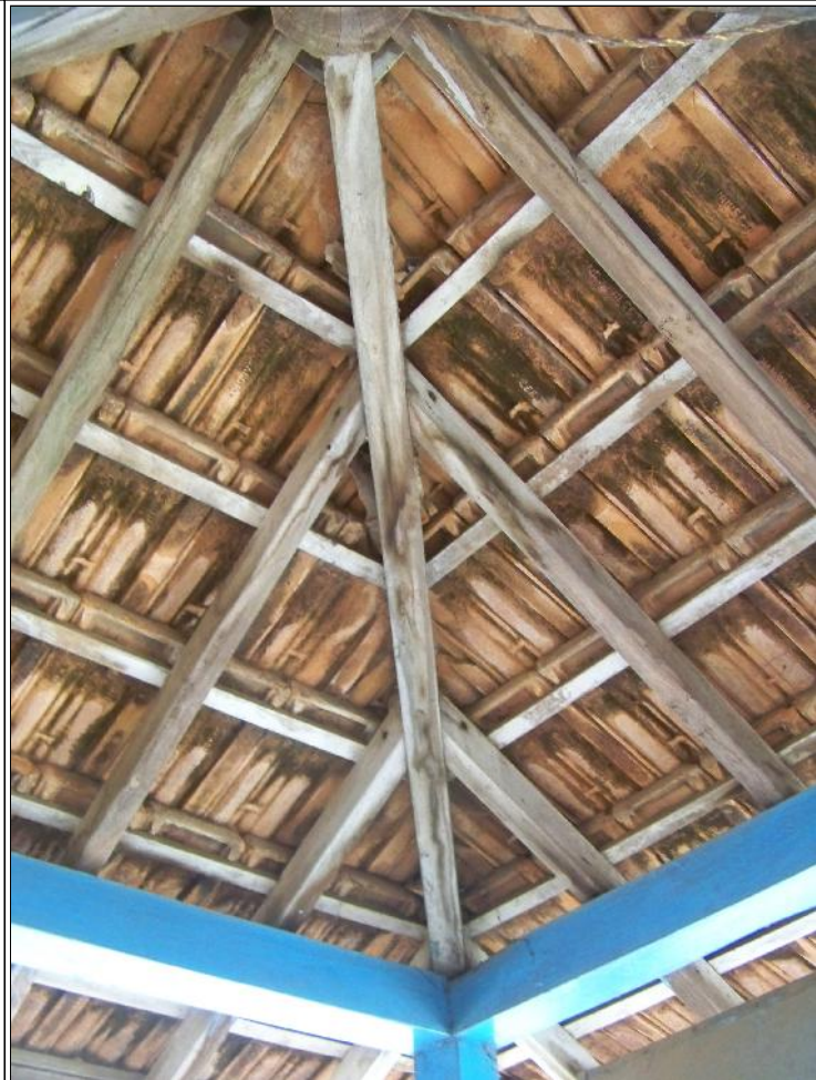
Image Title: Shree Kashivishweshwar Mandir Image Type: Top-View Reference: Wooden frames of the roof
