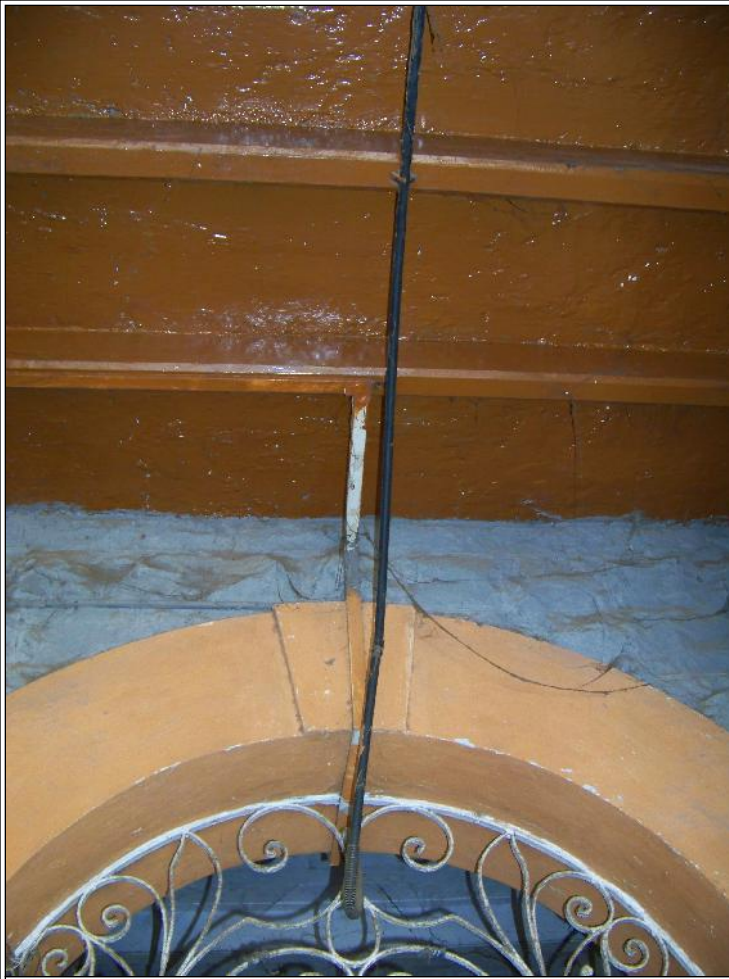
Image Title: Old Nagar Parishad Image Type: Top-View Reference: Arched opening with Psudo Structural Keystone
