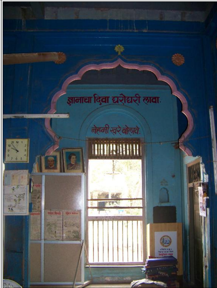
Image Title: Biwalkar Shiv Mandir Image Type: Front-View Reference: Internal view showing multifoiled arches and full height windows behind Garish oil paint is an inappropriate intervention and needs to be removed
