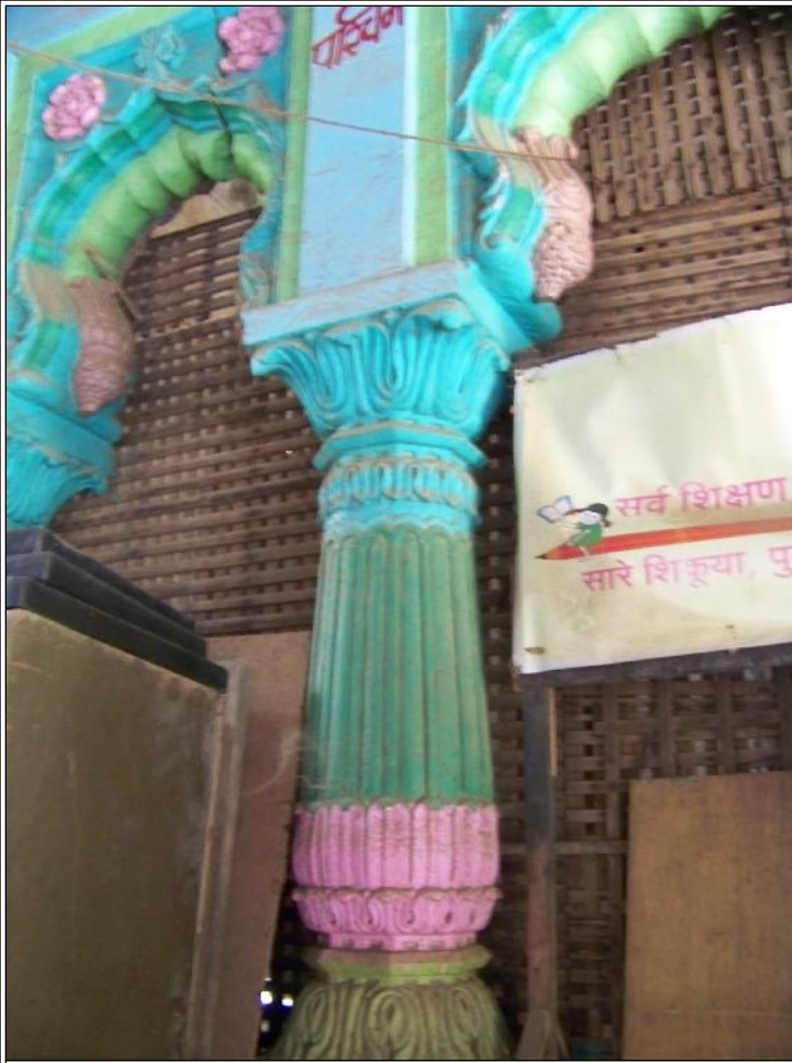
Image Title: Biwalkar Shiv Mandir Image Type: Front-View Reference: View of Baluster column with multifoiled arches with banana flower springing points
