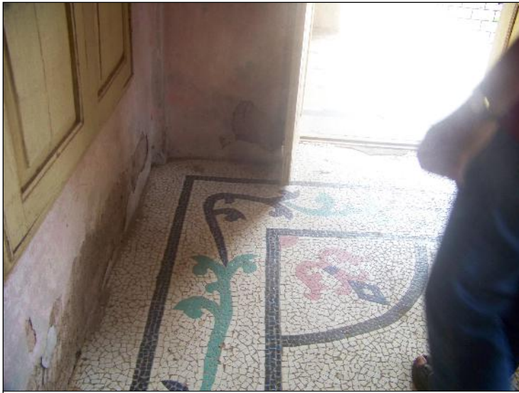
Image Title: Raigad Jilha Macchimar Sangha Ltd. Image Type: Front-View Reference: China mosaic flooring inside the structure
