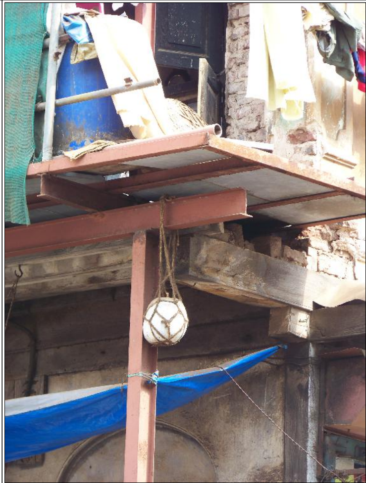
Image Title: Modi Wada Image Type: Top-View Reference: Incongruent MS Supports added to Balcony
