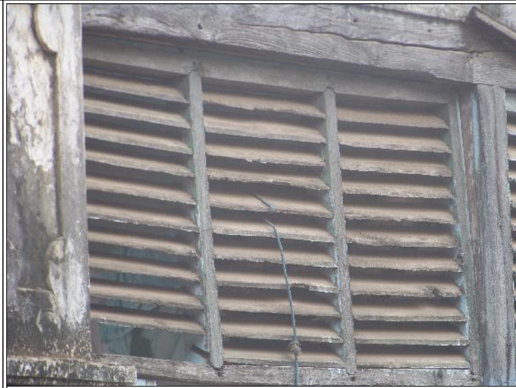
Image Title: Dabri House Image Type: Top-View Reference: Louvered openings acting as sun screens at ground floor of verandah
