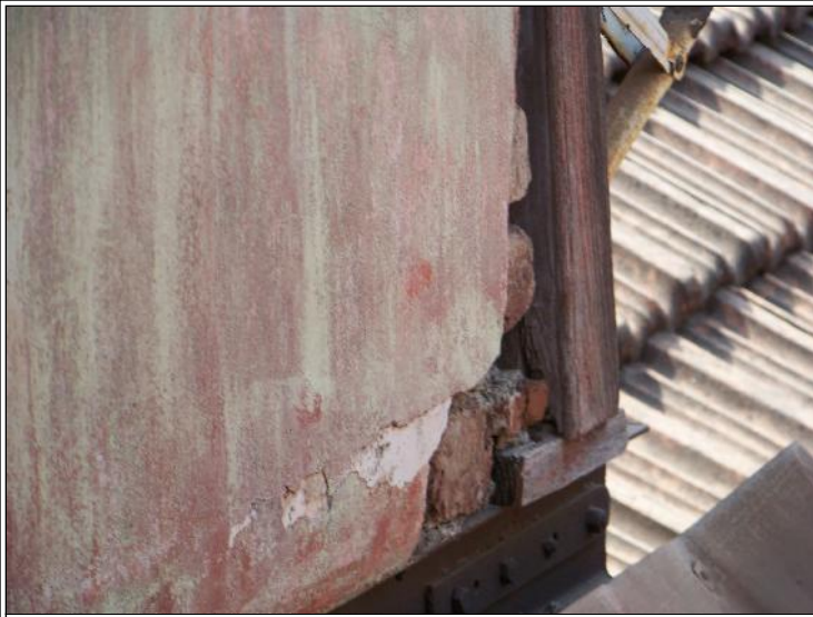
Image Title: Manohar Chawl Image Type: Front-View Reference: Deteriorating walls of timber work
