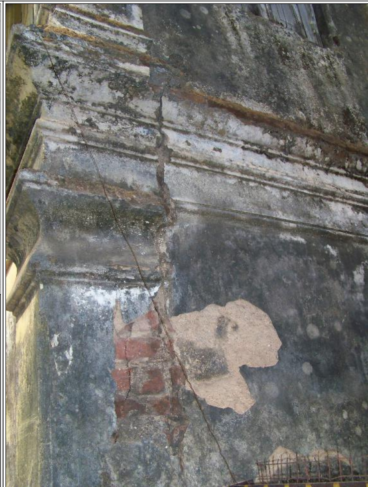
Image Title: Kelkar Wada Image Type: Side-View1 Reference: Moss growth on plaster cracking and peeling off of the plaster is apparant or the external surface
