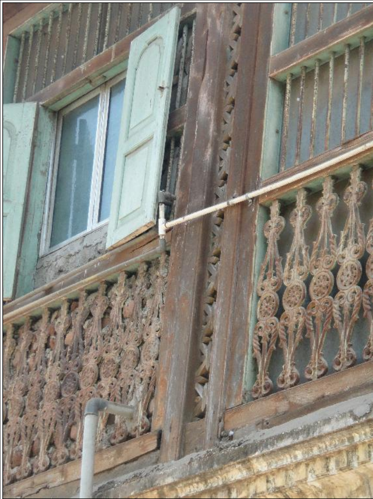
Image Title: Bhagwat Wada Image Type: Front-View Reference: Cast iron baluster and the window behind added later.
