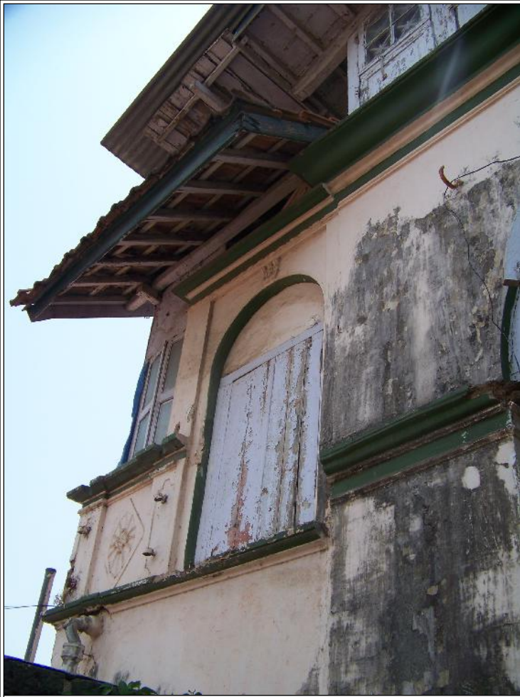
Image Title: Dharkar Wada Image Type: Rear-View Reference: Disfiguration due to dampness
