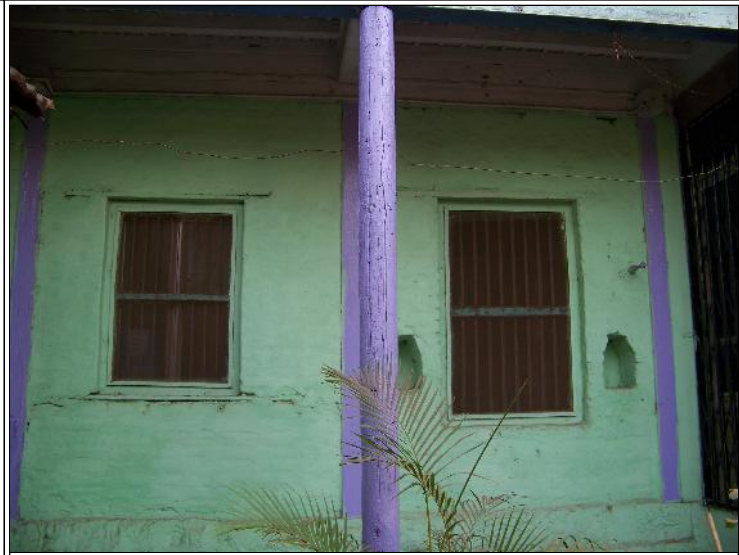
Image Title: Mandlik Wada Image Type: Top-View Reference: At Ground Floor rounded timber column and grilled windows with panelled shutters
