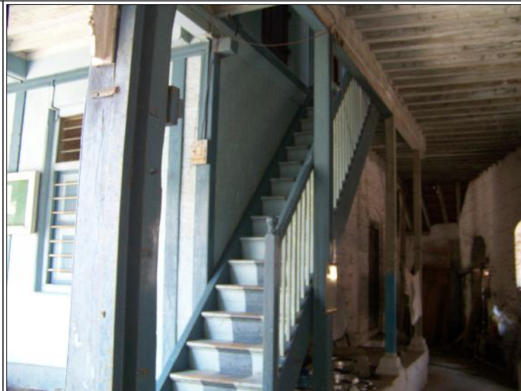
Image Title: Parmar Wada Image Type: Top-View Reference: Timber stairs and floor
