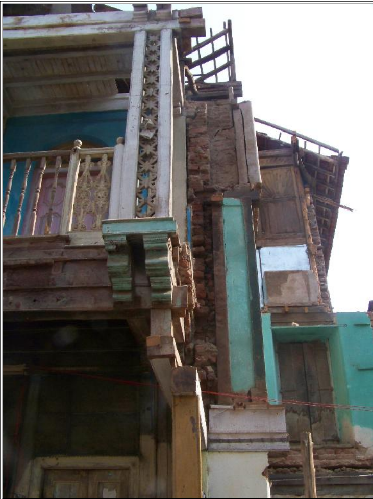
Image Title: Bhagwat Wada Image Type: Front-View Reference: Badly damaged corner of the house
