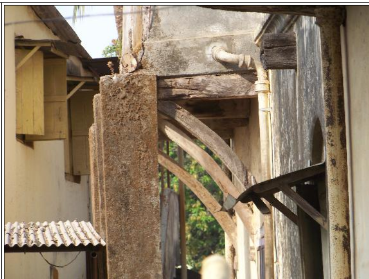
Image Title: Tilak Wada Image Type: Side-View1 Reference: temporary support to the upper floor
