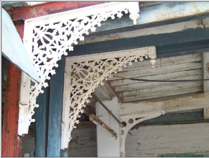
Image Title: Parmar Wada Image Type: Top-View Reference: Ornate cast iron brackets
