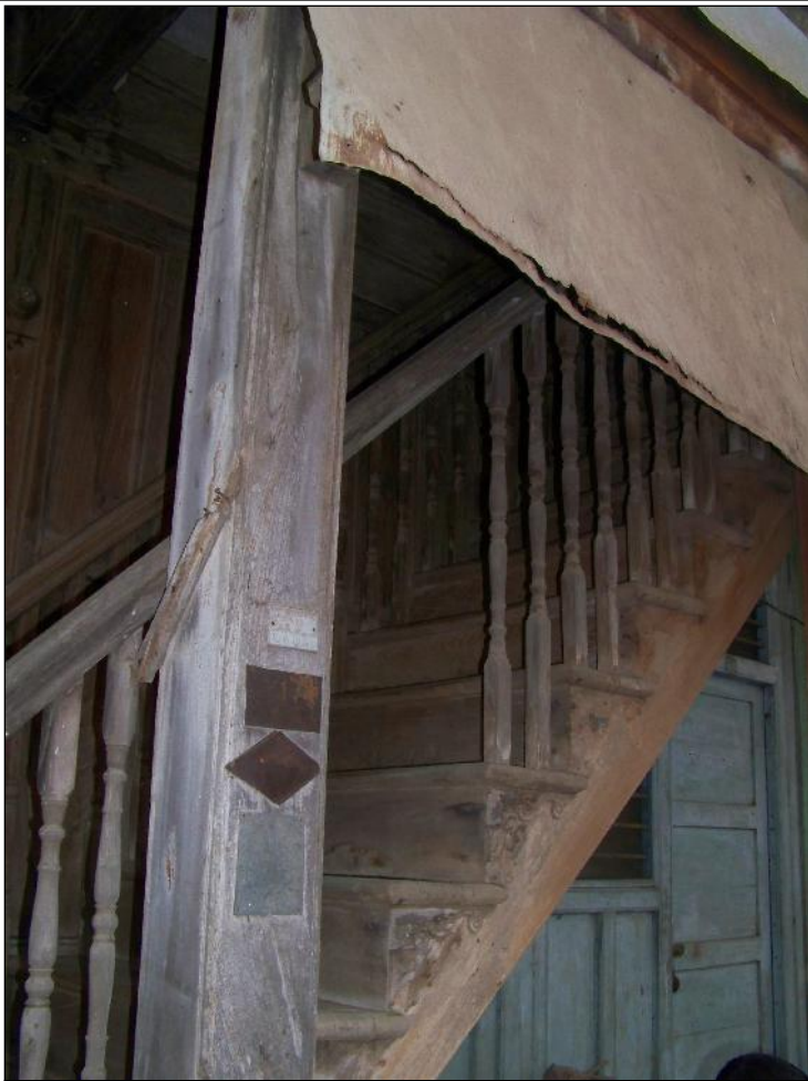
Image Title: Bhagwat Wada Image Type: Front-View Reference: Deteriorating woodwork missing balusters of the stairs
