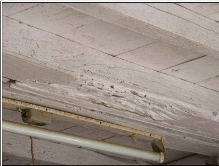
Image Title: Ahilya Mandal Image Type: Top-View Reference: A Floor beam showing damage due to dampness
