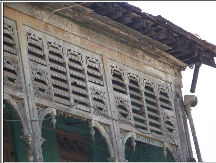
Image Title: Asha Niwas Image Type: Front-View Reference: Wooden louvered panels of the first floor balcony form a prominent character giving feature of the building. These how are not in a good shape and require urgent repairs
