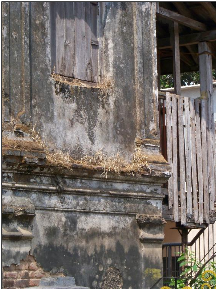
Image Title: Kelkar Wada Image Type: Side-View2 Reference: Overgrowth, Dampness, destruction of details are some of the problems of the building
