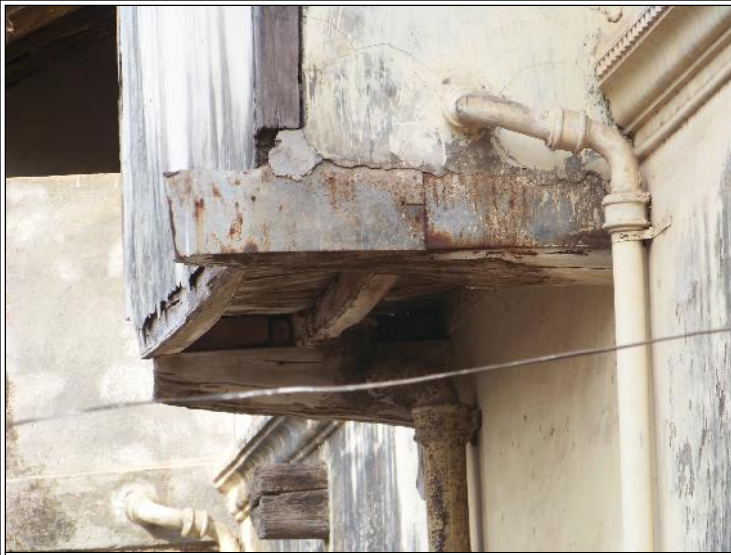
Image Title: Tilak Wada Image Type: Front-View Reference: Deterioration due to water seepage
