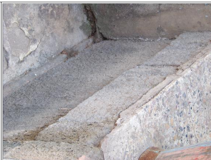
Image Title: Beth Haelohim Synagogue Image Type: Front-View Reference: Deterioration of the store on the exterior of the building
