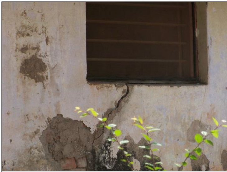
Image Title: Ghangrekar Wada Image Type: Front-View Reference: Detail of cracking of the wall on the front side
