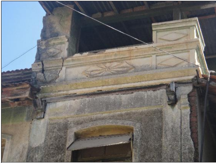
Image Title: Londhe Wada Image Type: Front-View Reference: Deterioration of the stucco work
