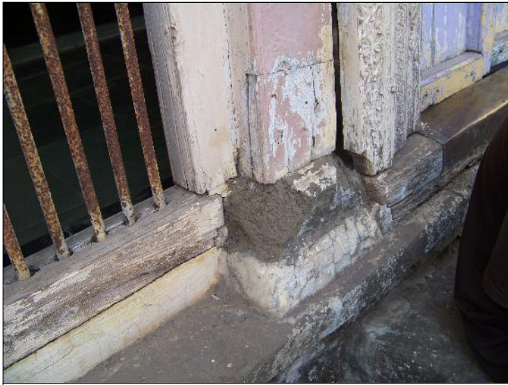
Image Title: Mahakali Mandir Image Type: Front-View Reference: Deteriorating Wood work
