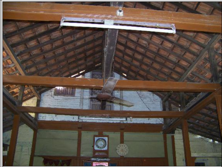
Image Title: Gosavi Datta Mandir Image Type: Top-View Reference: Timber roof of the sabhagriha
