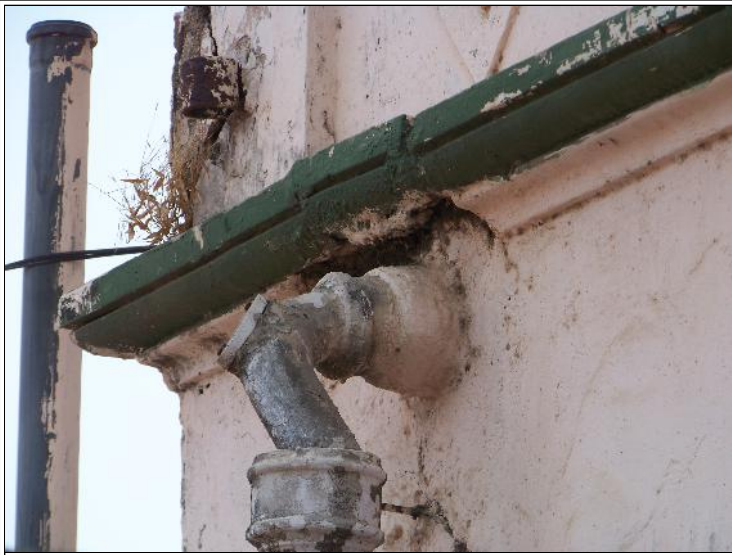
Image Title: Dharkar Wada Image Type: Front-View Reference: Drainage connection added later
