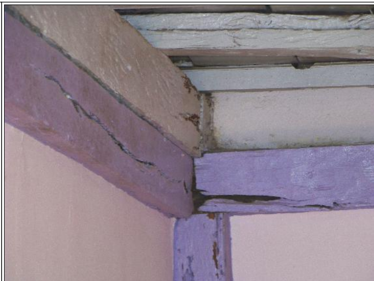
Image Title: Datar Ganpati Mandir Image Type: Top-View Reference: Deterioration of the woodwork
