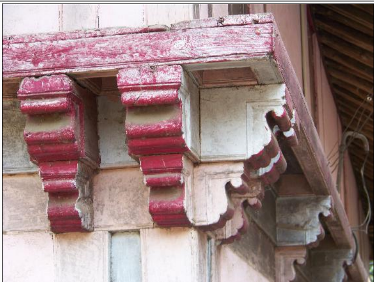
Image Title: Ziral Ali Ganpati Mandir Image Type: Top-View Reference: Corner brackets of the exterior facade of the temple
