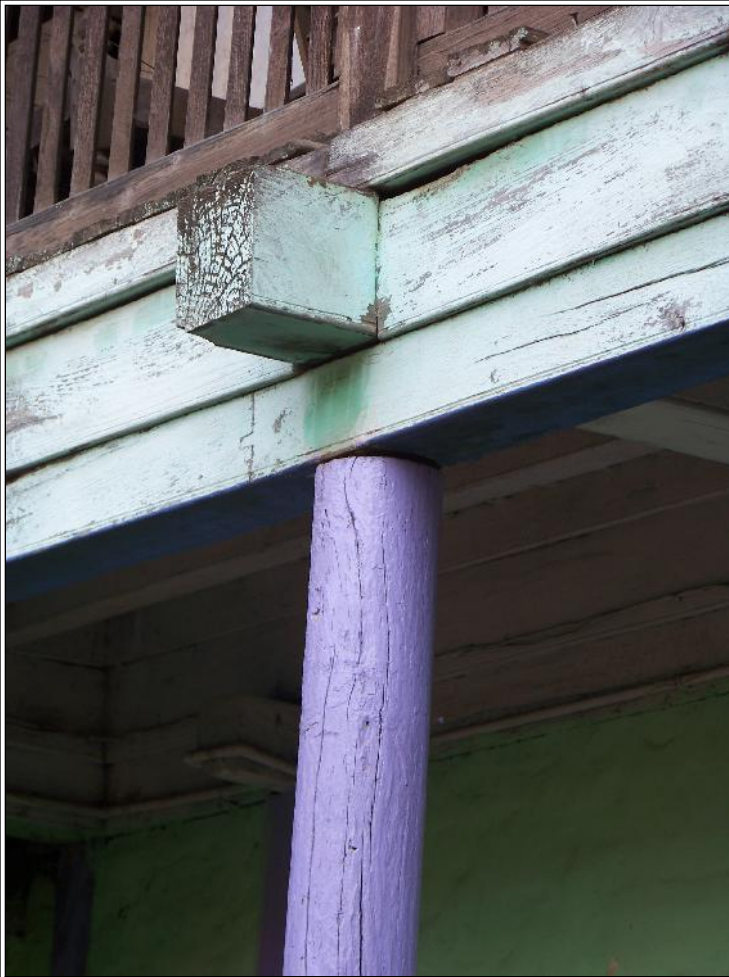
Image Title: Mandlik Wada Image Type: Top-View Reference: Detail of wooden column and beam junction
