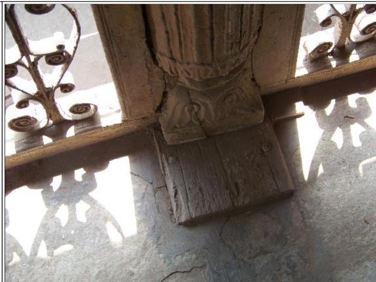
Image Title: More Wada Image Type: Front-View Reference: Deteriorating timber work on First Floor
