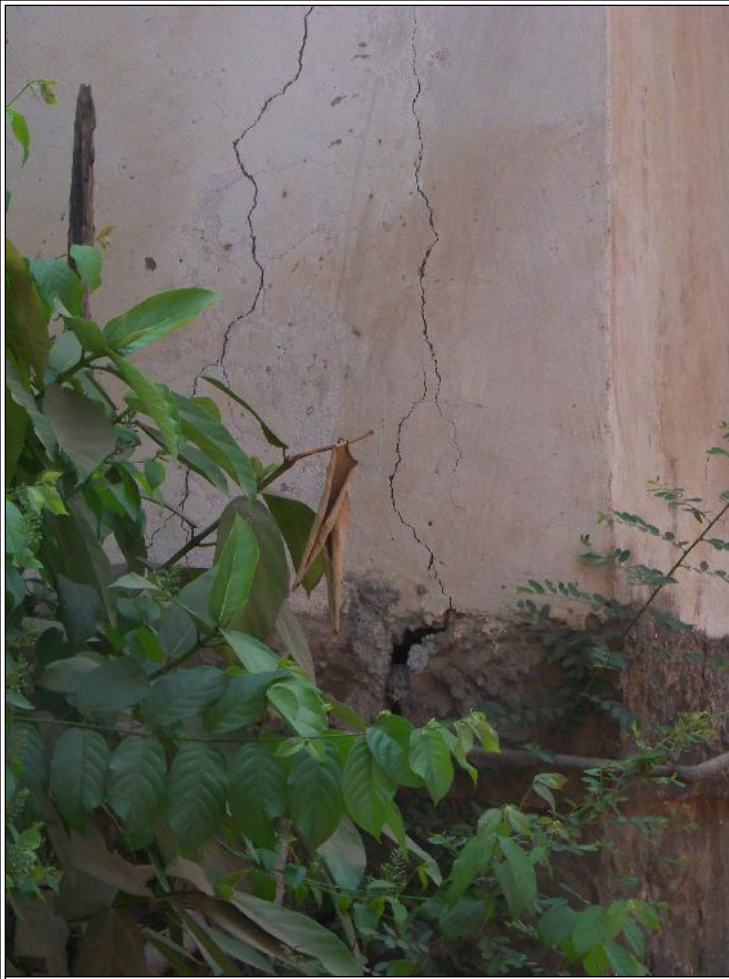
Image Title: Limaye Wada Image Type: Front-View Reference: Cracking of plaster on the exterior
