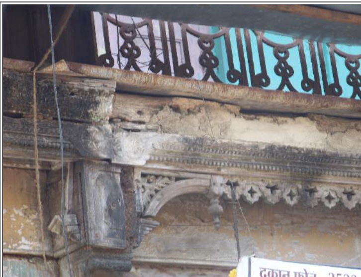
Image Title: Asha Niwas Image Type: Front-View Reference: A Deterioration of wooden elements of the building
