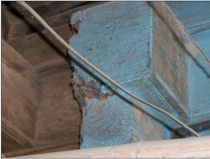
Image Title: More Wada Image Type: Top-View Reference: Weathered timber beam head
