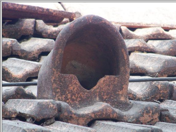
Image Title: Parmar Wada Image Type: Top-View Reference: cowl/ vent in terracota fixed in the mangalore tile roof
