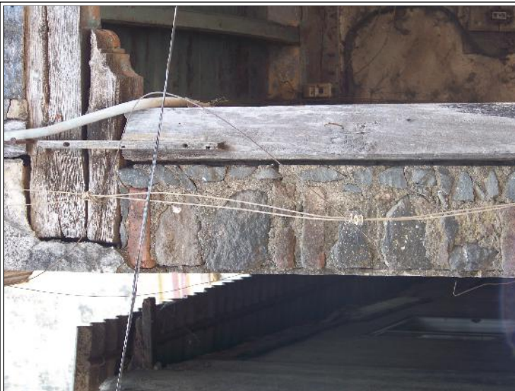
Image Title: Karmarkar Wada Image Type: Front-View Reference: Weathered timber frame cracked joints
