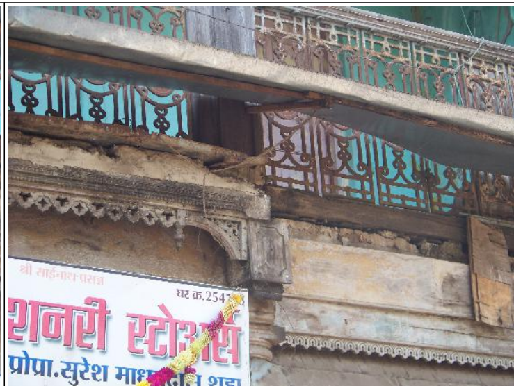
Image Title: Asha Niwas Image Type: Front-View Reference: Damaged wooden elements of the front facade of the building
