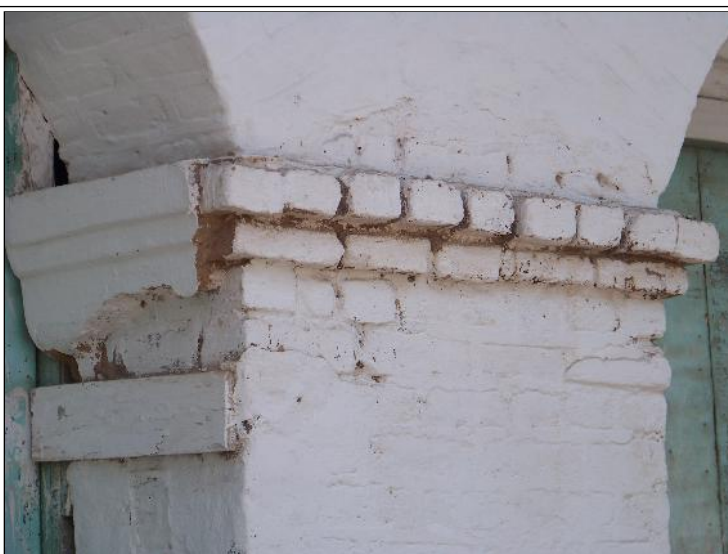
Image Title: Parmar Wada Image Type: Top-View Reference: Deteriorating Plaster
