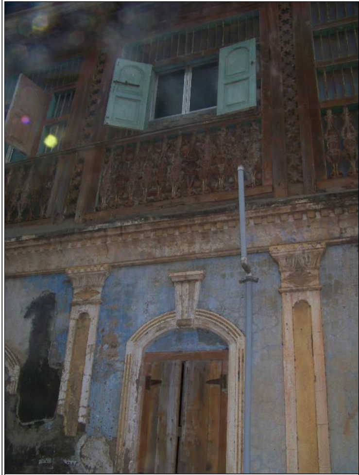
Image Title: Bhagwat Wada Image Type: Front-View Reference: Detail of the stucco work around the opening on the facade. The balcony on the first floor that is enclosed later is also seen.
