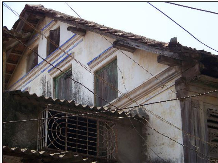
Image Title: Asha Niwas Image Type: Side-View1 Reference: Detail of the gable wall with prominent cornice bands
