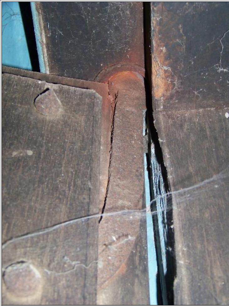
Image Title: Patil House Image Type: Front-View Reference: Detail of door pivot
