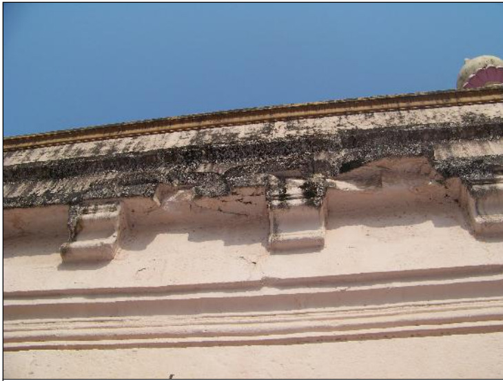
Image Title: Goteswar Mandir Image Type: Top-View Reference: Short brackets of the roof
