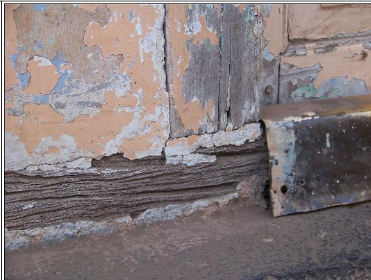
Image Title: Hanuman Mandir Image Type: Side-View1 Reference: Rotting timber of the temple structure
