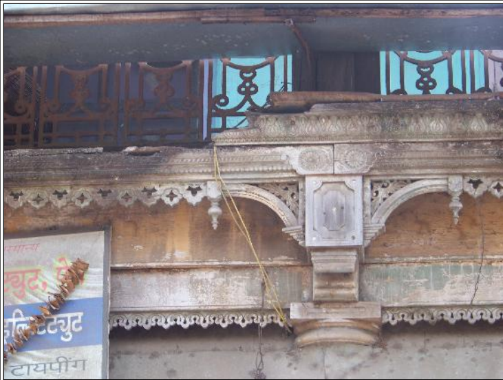
Image Title: Asha Niwas Image Type: Front-View Reference: Detail of the balcony edge showing intricate woodwork how obscured by insensitive additions
