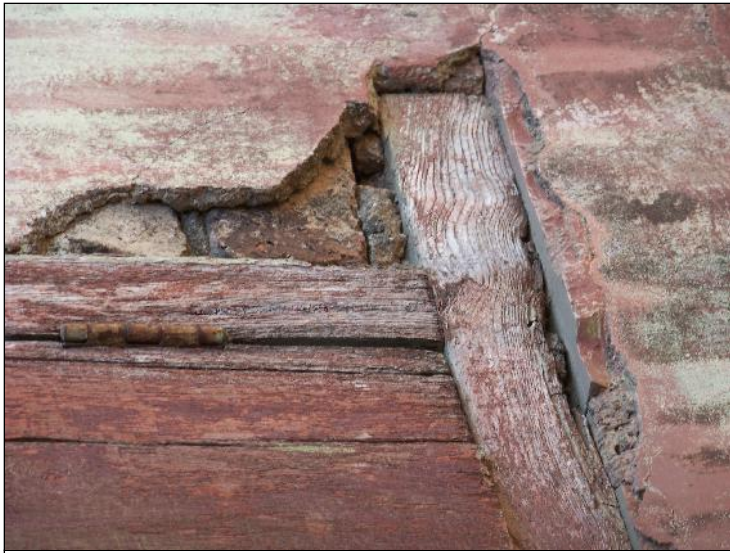
Image Title: Manohar Chawl Image Type: Top-View Reference: Deteriorating timber work
