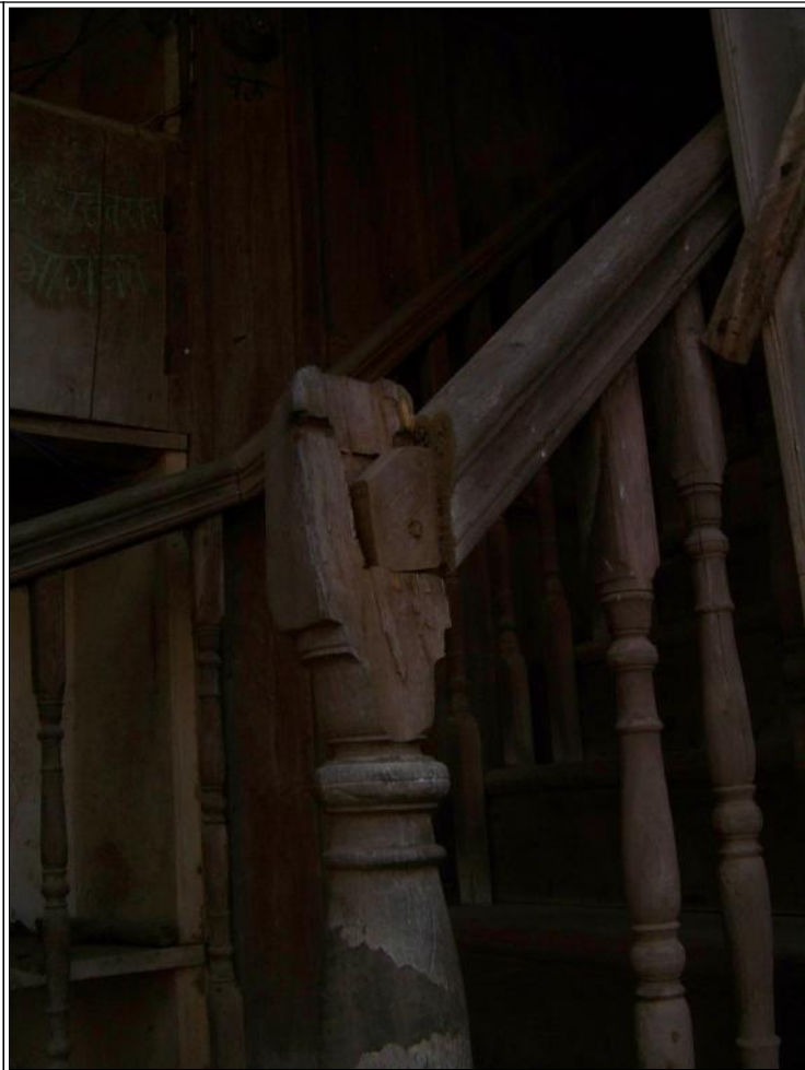
Image Title: Bhagwat Wada Image Type: Front-View Reference: Deterioration of wood work
