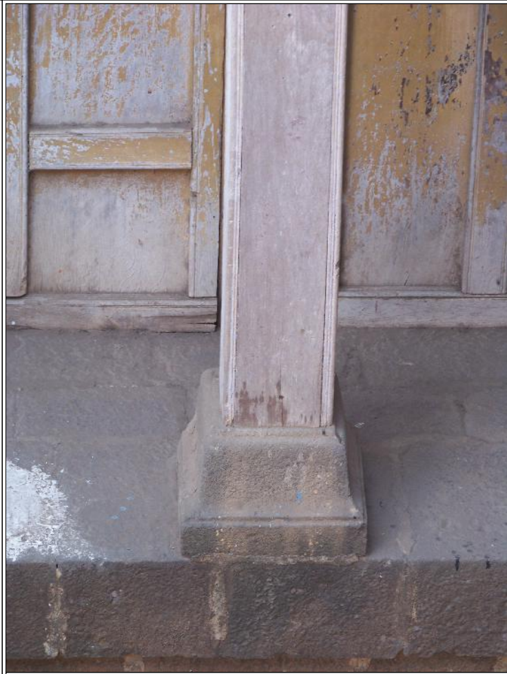
Image Title: More Wada Image Type: Front-View Reference: Stone base of timber column in verandah
