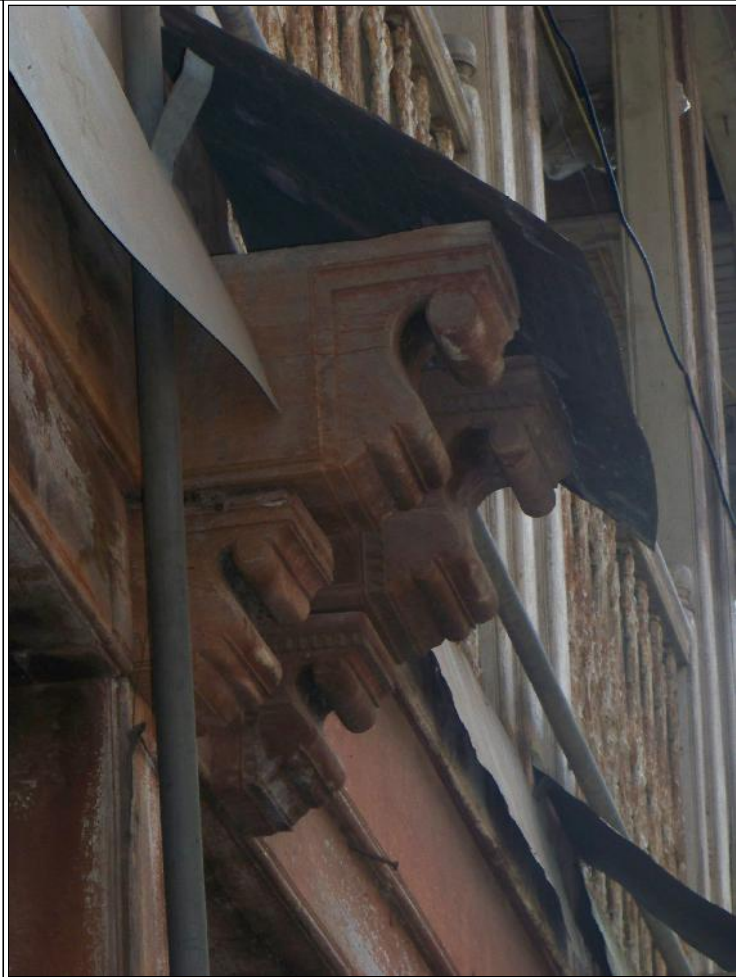
Image Title: Bhagwat Wada Image Type: Front-View Reference: Detail of the wooden medallions on the facade and the adhoc protection measures
