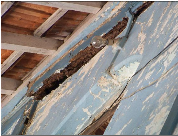
Image Title: Parmar Wada Image Type: Top-View Reference: Rain water damage to the verandah roof
