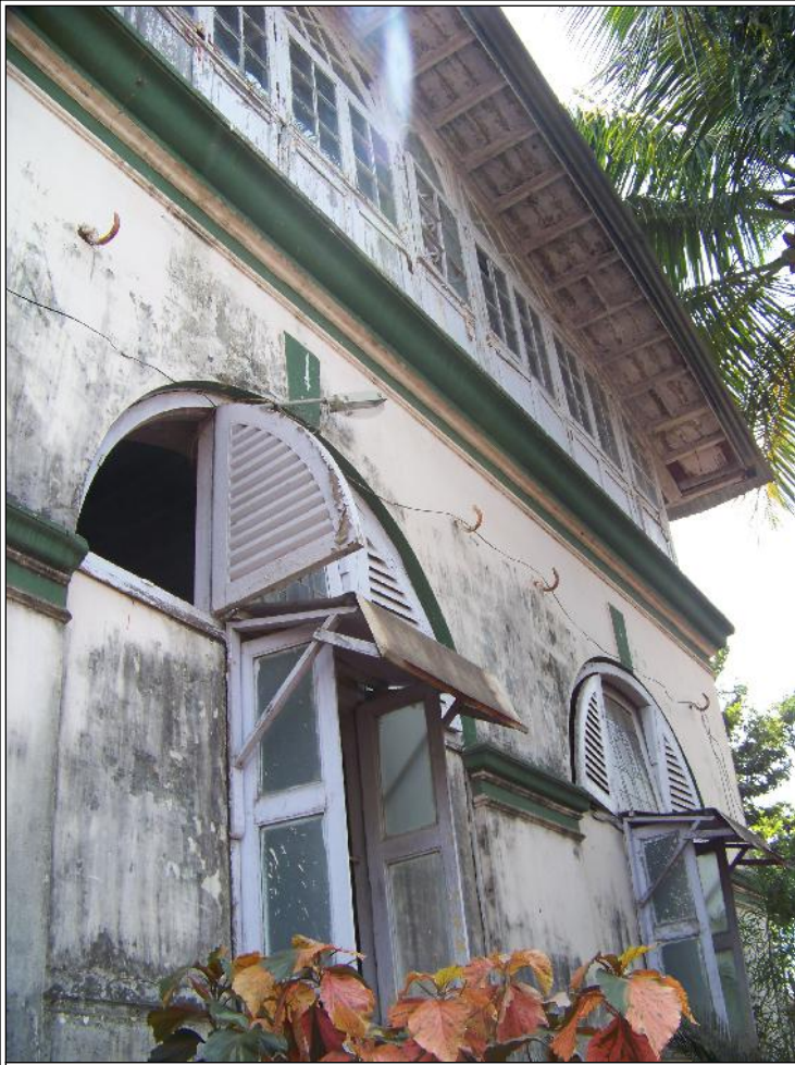
Image Title: Dharkar Wada Image Type: Side-View1 Reference: Street facing arched openings of the verandah later filled in with windows
