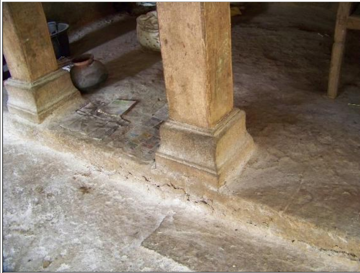
Image Title: Deshpande Wada Image Type: Front-View Reference: Detail of stone pedestal of the timber columns
