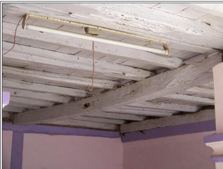
Image Title: Datar Ganpati Mandir Image Type: Top-View Reference: Deteriorating wooden ceiling of the temple
