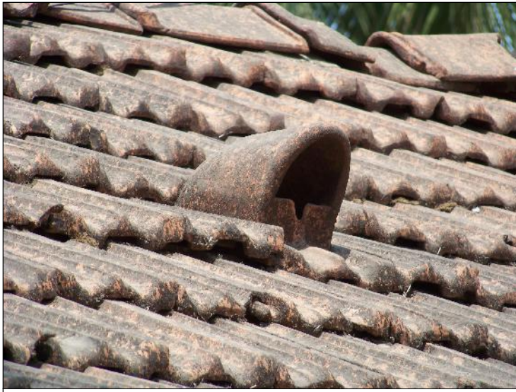
Image Title: Parmar Wada Image Type: Top-View Reference: Detail of roof showing a teracota vent.
