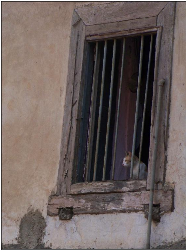
Image Title: Limaye Wada Image Type: Front-View Reference: Window detail showing the deterioration and ageing of the timber
