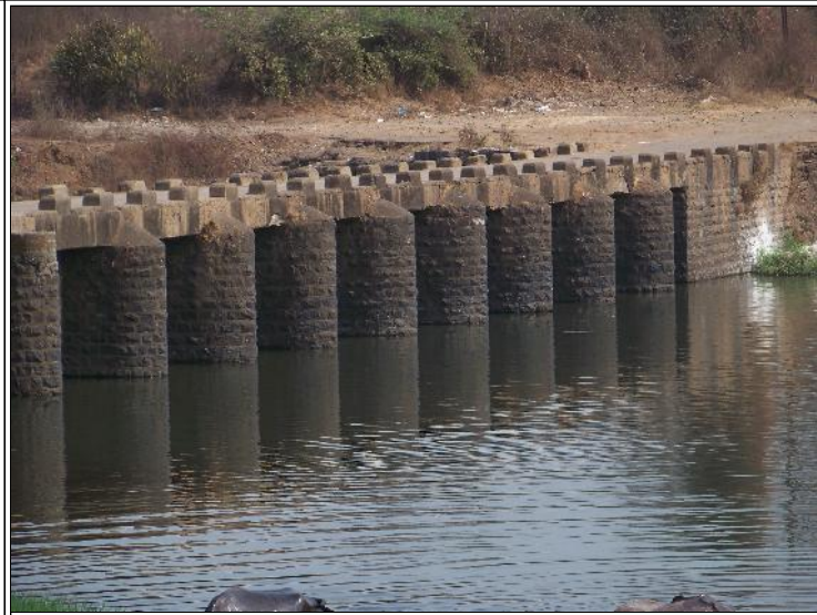
Image Title: Bridge Image Type: Side-View1 Reference: Masonary Piers on one side of the bridges. Arches are not seen from this side either
