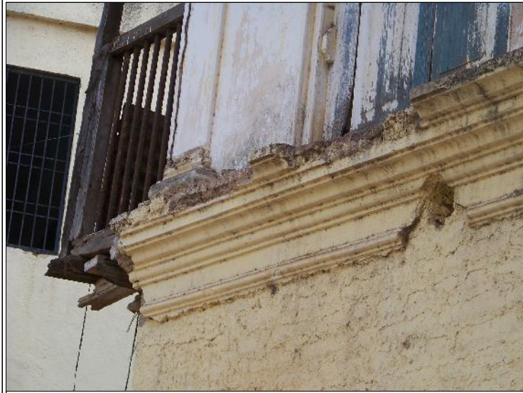
Image Title: Patil House Image Type: Front-View Reference: Damaged lime mortar cornice on the exterior of the building. Also seen is the damaged timber of the balcony
