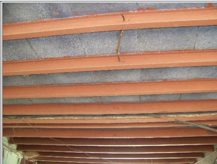
Image Title: Manohar Chawl Image Type: Top-View Reference: Ceiling of the entry to the chawl using I sections of Shahbad tiles
