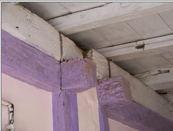
Image Title: Datar Ganpati Mandir Image Type: Top-View Reference: Deterioration to structural woodwork
