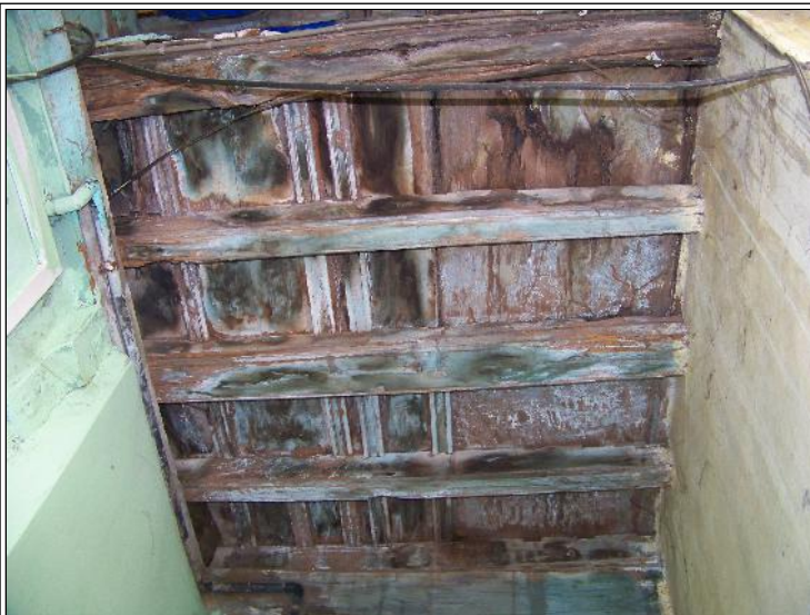
Image Title: Mandlik Wada Image Type: Top-View Reference: Water leakage in the wooden ceiling
