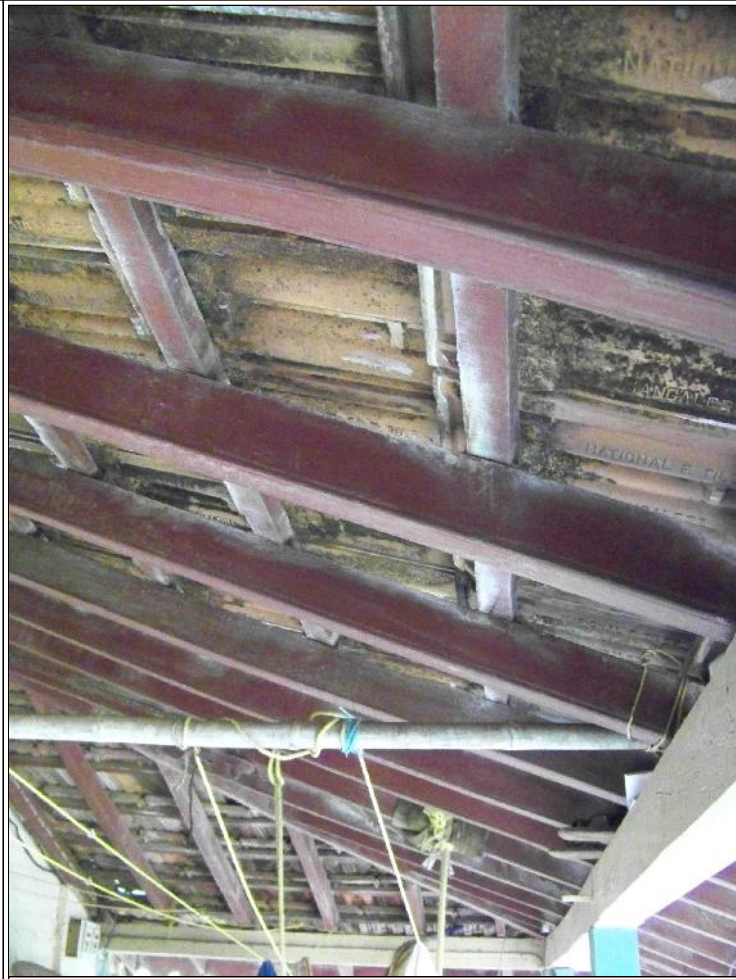
Image Title: Mukadam House Image Type: Top-View Reference: Close up of ceiling with timber members and mangalore tiles
