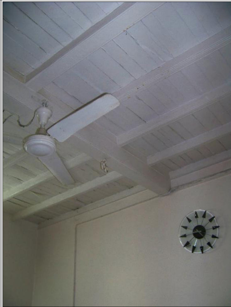
Image Title: Kale House Image Type: Front-View Reference: Timber floor of ceiling as seen in the interior
