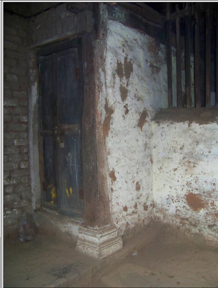
Image Title: Pimputkar Wada Image Type: Front-View Reference: Wooden column of load bearing walls form the structural support.
