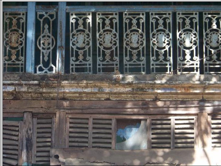
Image Title: Bafna House Image Type: Top-View Reference: The wooden ventilators of the cast iron balusters of the first floor
