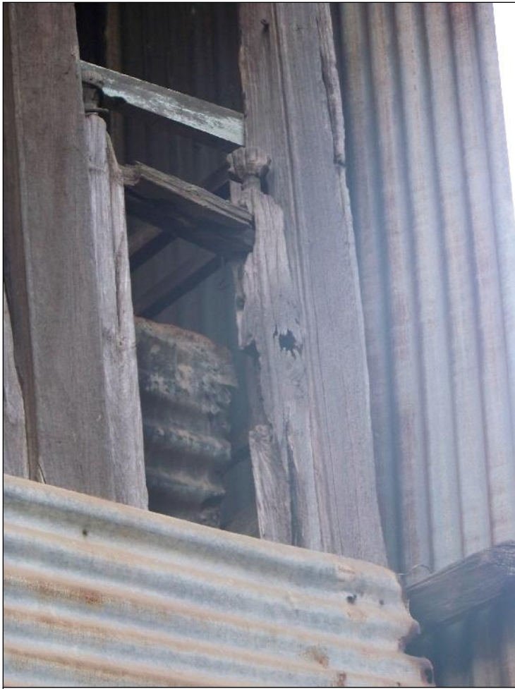
Image Title: Medhi House Image Type: Front-View Reference: deteriorating timber work
