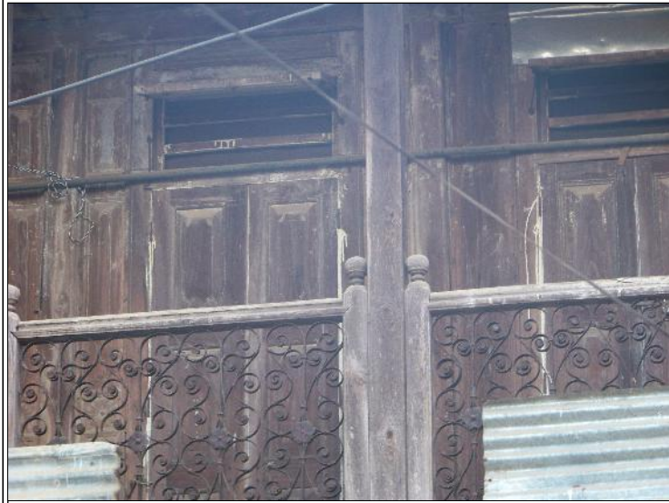
Image Title: Medhi House Image Type: Front-View Reference: Close up of the wrought iron grill of the first floor gallery
