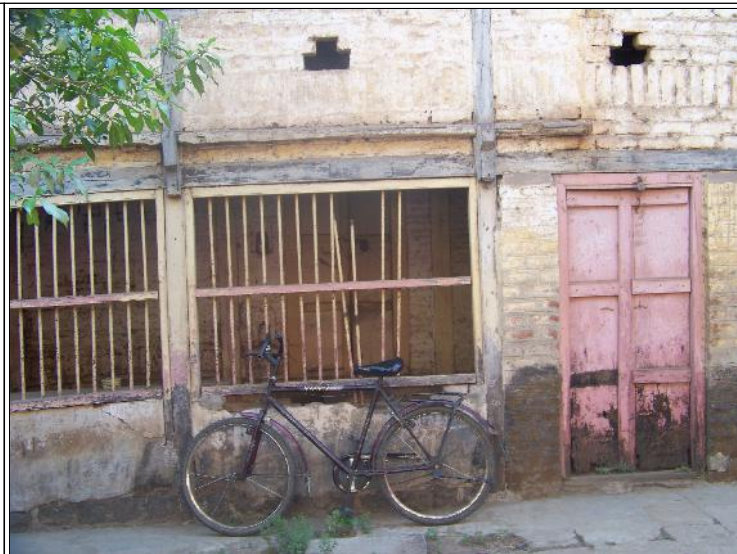
Image Title: Vaidya House Image Type: Front-View Reference: Broken grills on the ground floor
