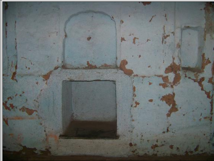
Image Title: Pimputkar Wada Image Type: Front-View Reference: Niches in the load bearing walls
