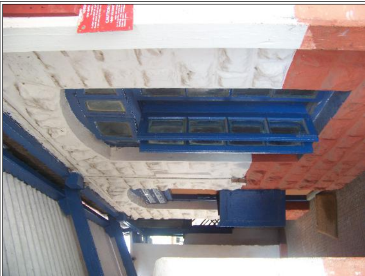
Image Title: Railway Station Image Type: Front-View Reference: Room along the platform built in rusticated masonry
