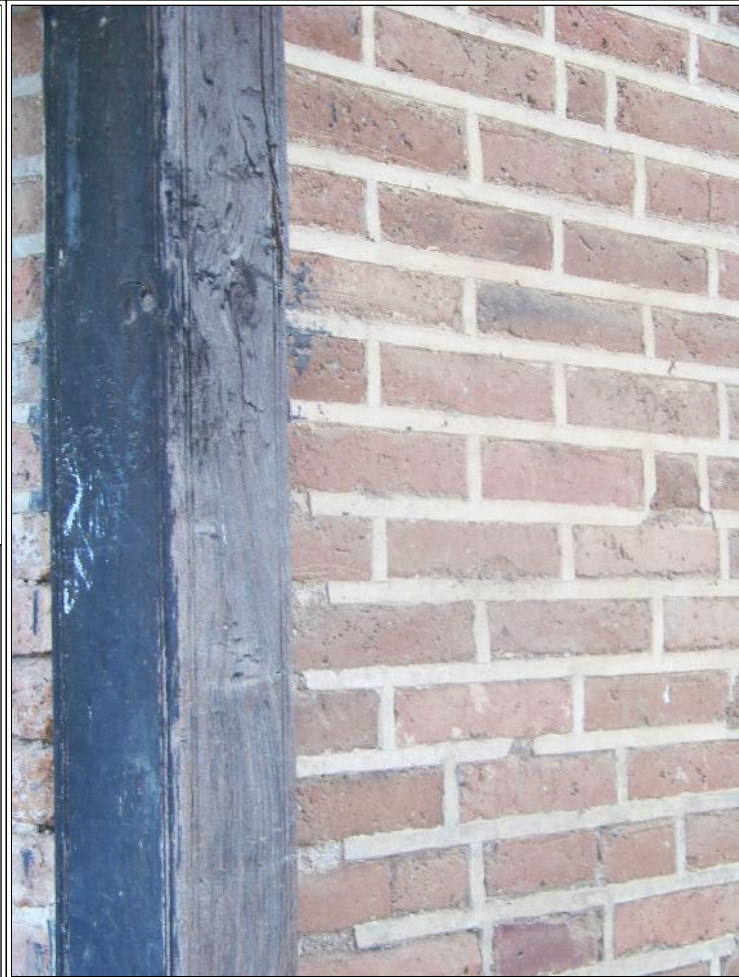
Image Title: Medhi House Image Type: Front-View Reference: Close up of the stretcher bond brick work
