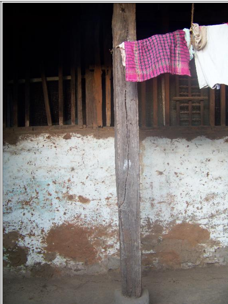
Image Title: Pimputkar Wada Image Type: Front-View Reference: Deterioration of timber
