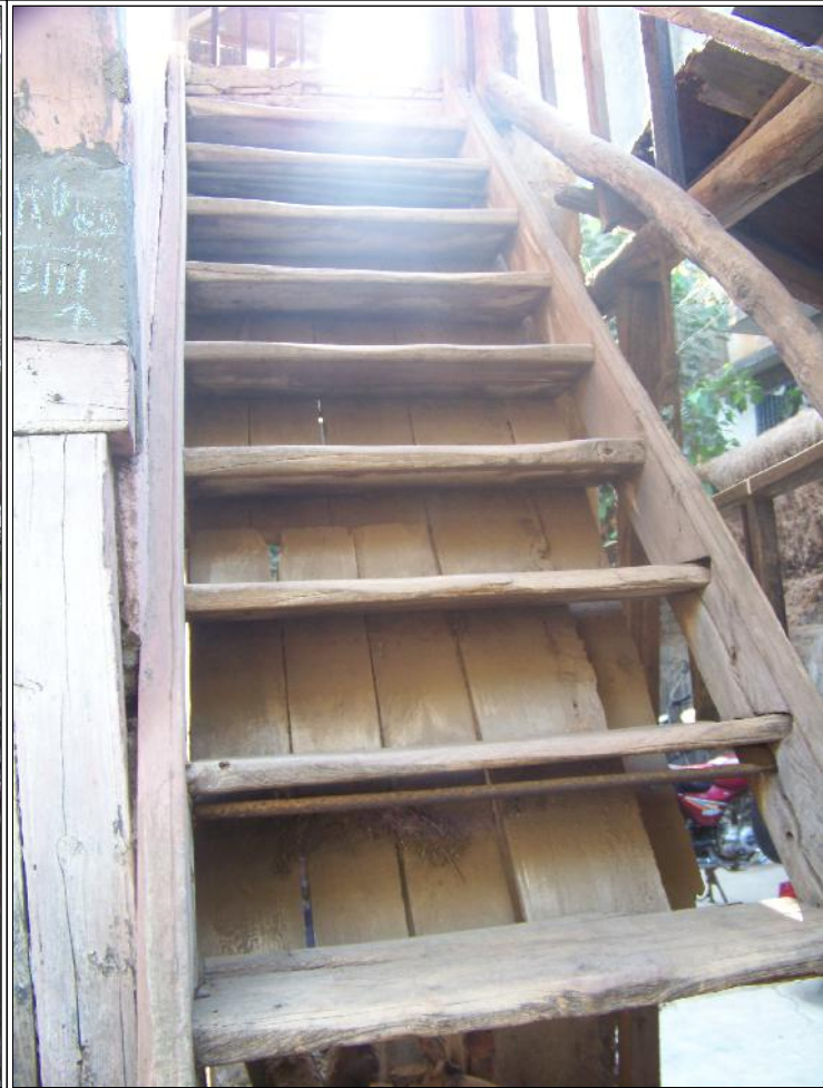
Image Title: Vaidya House Image Type: Front-View Reference: Detail of the weakened stairs.
