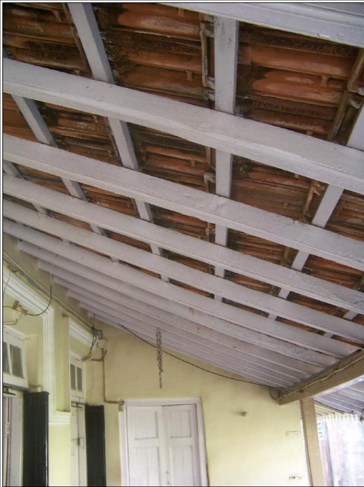
Image Title: Kale House Image Type: Top-View Reference: Leaned Mangalore tile and wooden roof from inside
