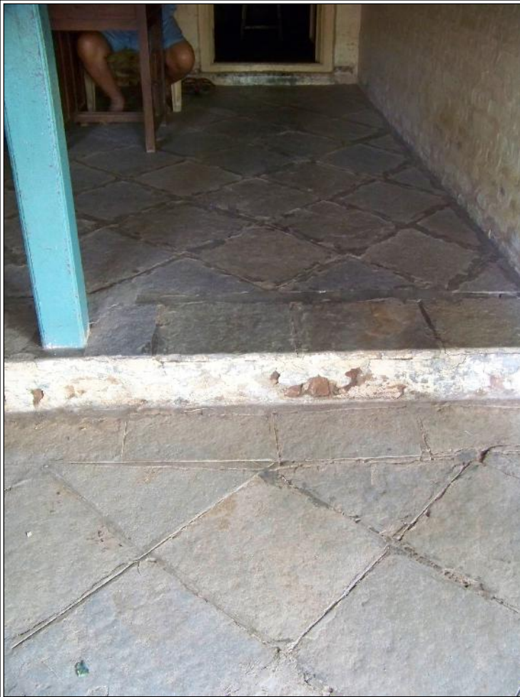
Image Title: Mukadam House Image Type: Front-View Reference: Diamond pattern shahabad flooring inside the house.
