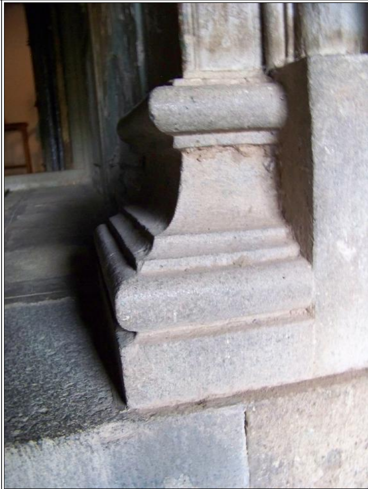
Image Title: Medhi House Image Type: Front-View Reference: Stone base to timber column
