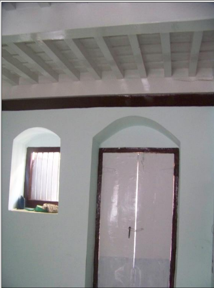
Image Title: Adv. Mulekar House Image Type: Front-View Reference: Arcuate openings with flat lintels above doors and windows
