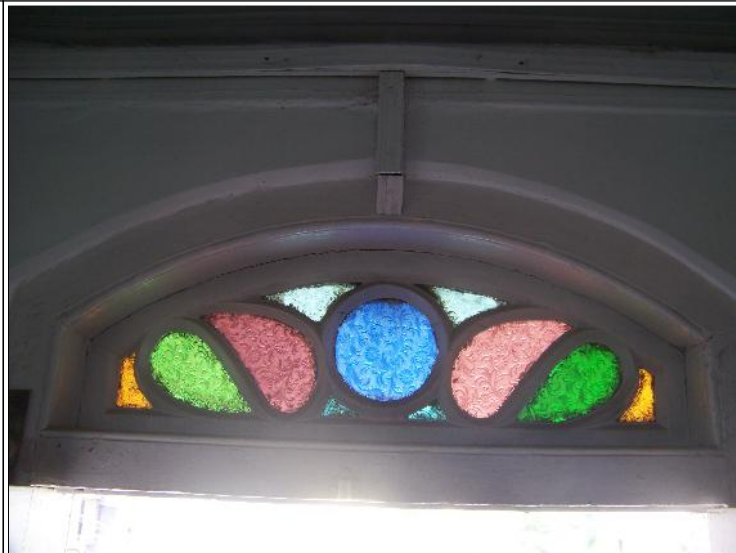
Image Title: Tilak Wada Image Type: Front-View Reference: Fanlight with coloured glass
