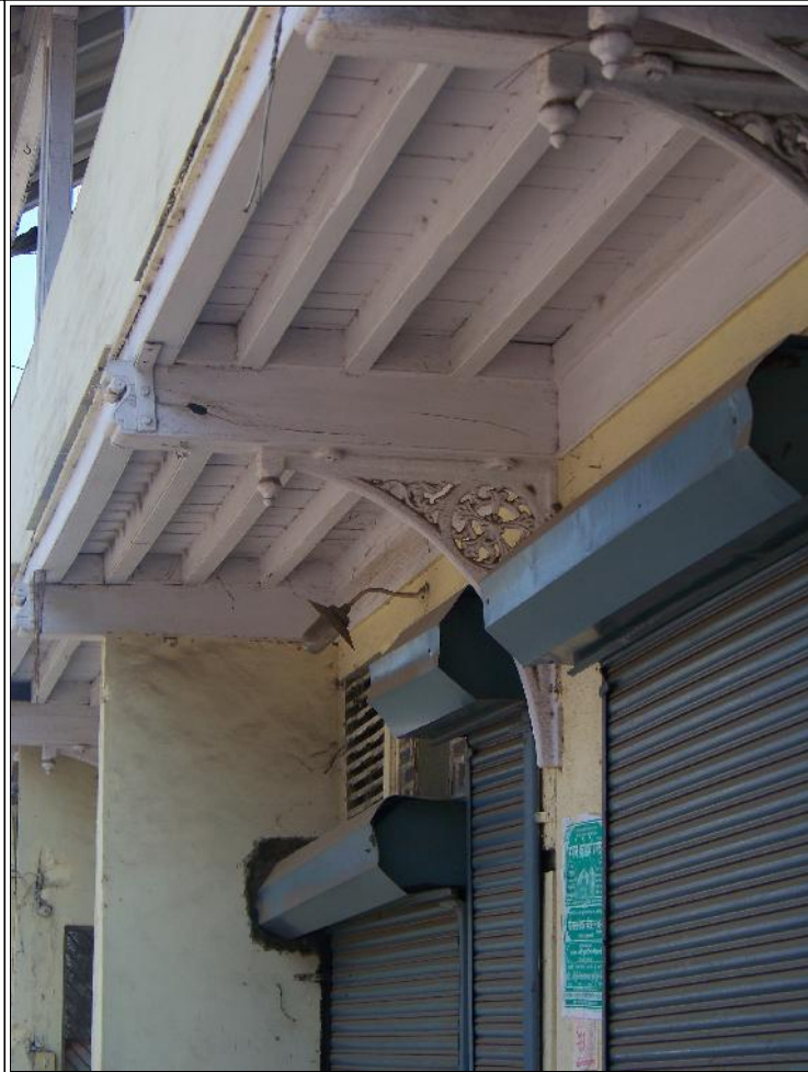
Image Title: Tilak Wada Image Type: Top-View Reference: Cast iron brackets
