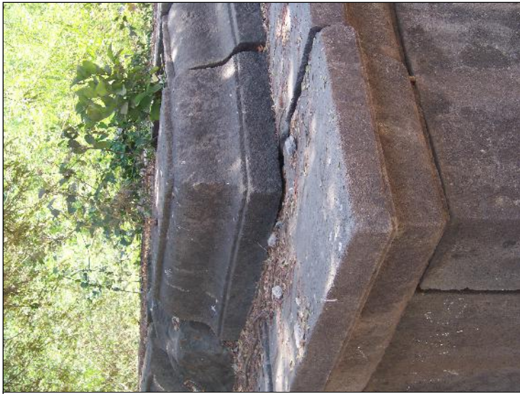
Image Title: Samadhi Image Type: Top-View Reference: Loosening of corner stones from top to bottom due to differential settlement
