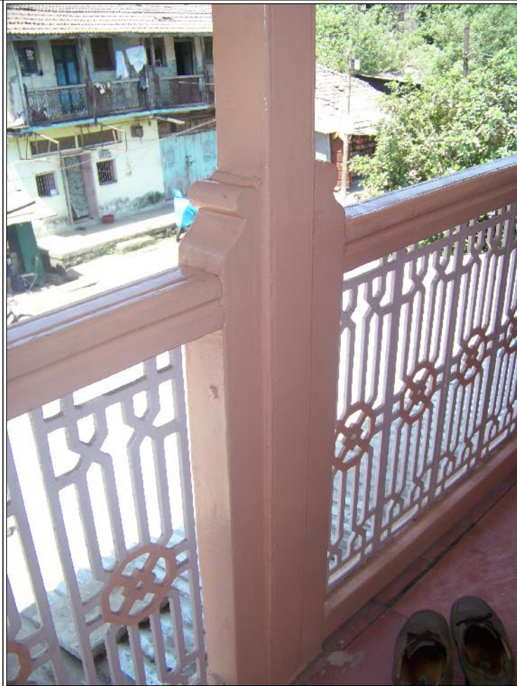
Image Title: Adv. Mulekar House Image Type: Front-View Reference: Wooden railing on first floor with cast iron infill panels
