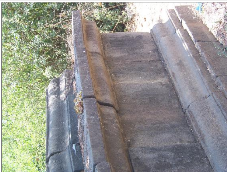
Image Title: Samadhi Image Type: Front-View Reference: Loosening of corner stones from top to bottom due to differential settlement
