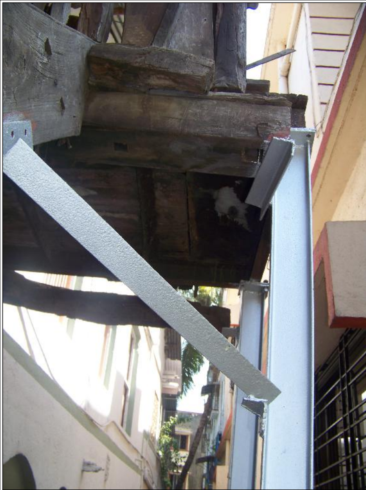
Image Title: Adv. Mulekar House Image Type: Front-View Reference: MS Bracket stays added to strengthen canti
