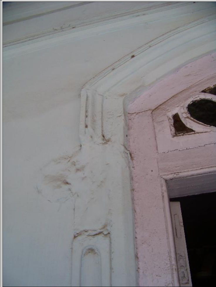
Image Title: Tilak Wada Image Type: Front-View Reference: Moulding around the openings obscured due to coats of paint
