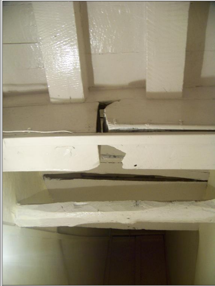
Image Title: Adv. Mulekar House Image Type: Front-View Reference: One of the roof beams showing signs of distress
