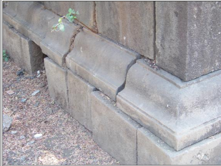
Image Title: Samadhi Image Type: Front-View Reference: Loosening of corner stones from top to bottom due to differential settlement
