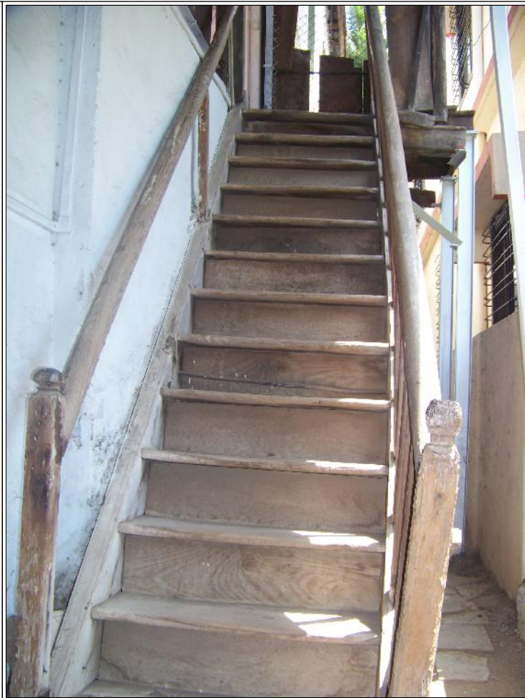
Image Title: Adv. Mulekar House Image Type: Front-View Reference: Wooden staircase connecting to first floor
