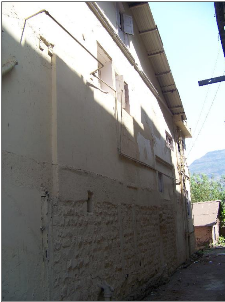
Image Title: Tilak Wada Image Type: Side-View1 Reference: View from side lane showing ground floor construction instone
