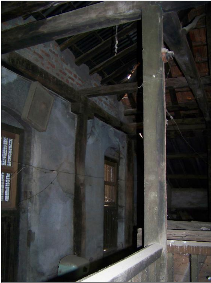
Image Title: Tilak Wada Image Type: Front-View Reference: Illmaintained first floor plaster peeling off unmaintained wood work
