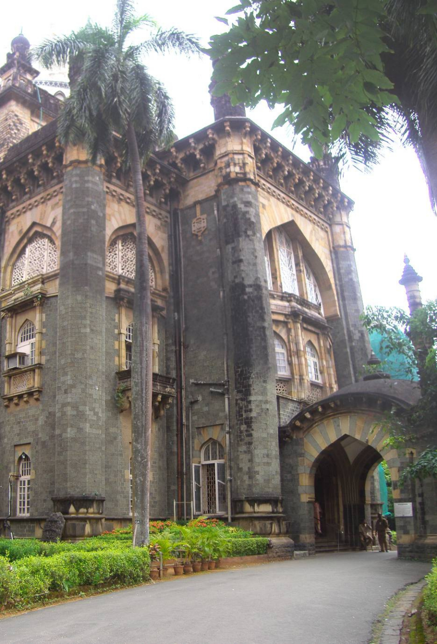
BEFORE RESTORATION BEFORE & AFTER RESTORATION
