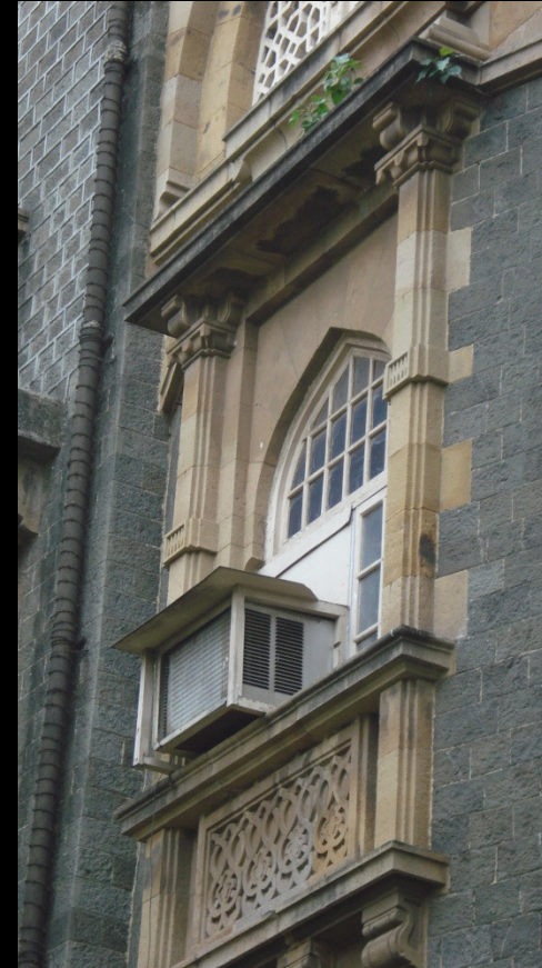
Photograph showing the Deterioration of the window frames Right: Photograph showing a window air conditioner unit mounted on the sill Below: Photograph showing the original window design with a glass fanlight and glazed shutters.
