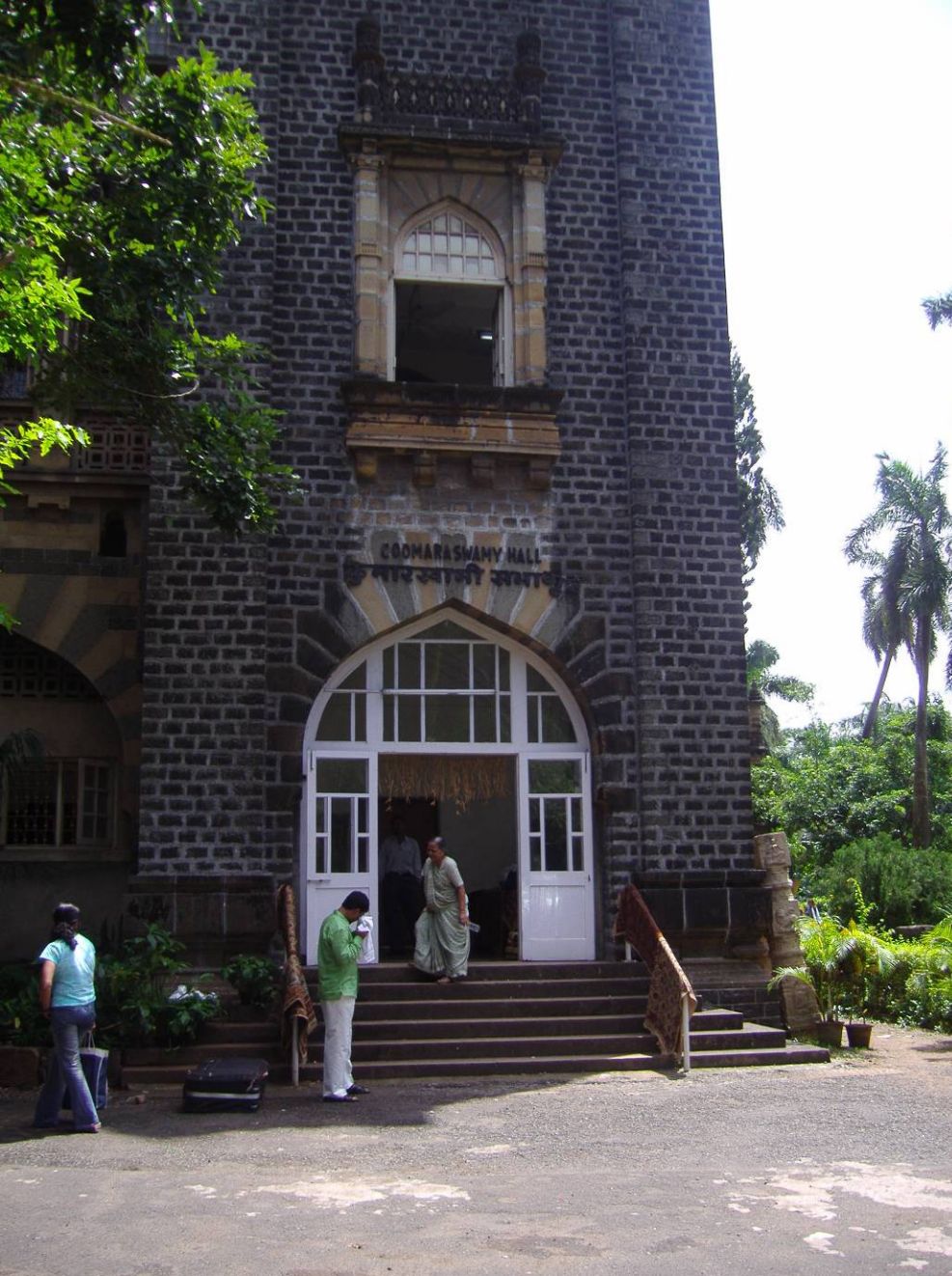
BEFORE RESTORATION BEFORE & AFTER RESTORATION
