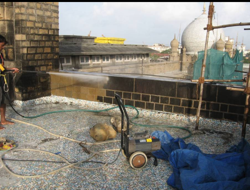
WATER MISTING AND SPECIALISED STONE CLEANING
