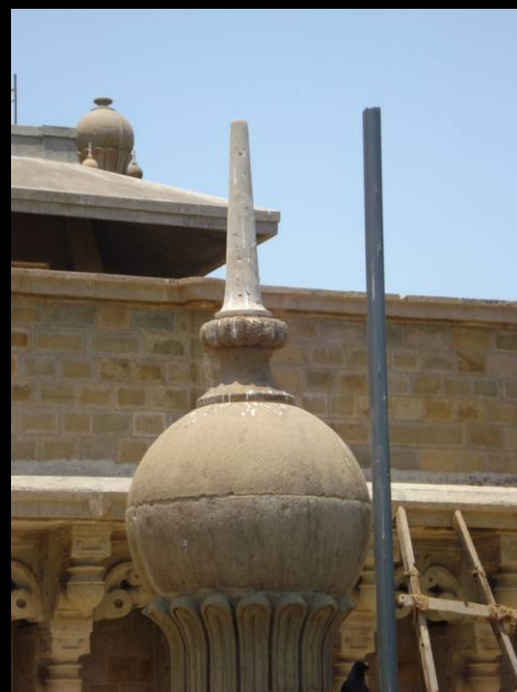
DUTCHMAN REPAIR AND REPLACING MISSING SECTIONS OF STONE GULDASTAS
