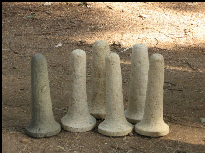
DUTCHMAN REPAIR AND REPLACING MISSING SECTIONS OF STONE GULDASTAS
